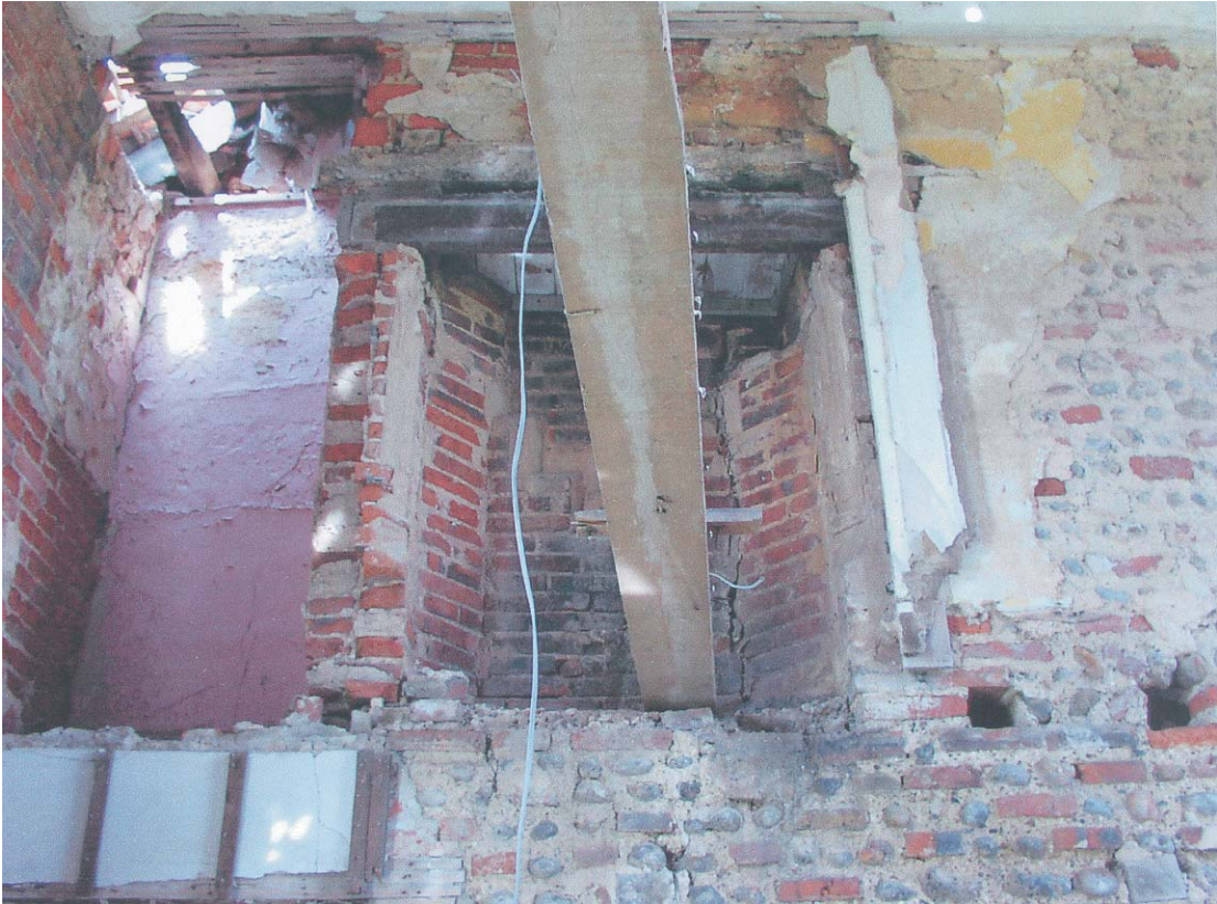
Plate 6 The 16th-century fireplace, north wall, at first floor level
