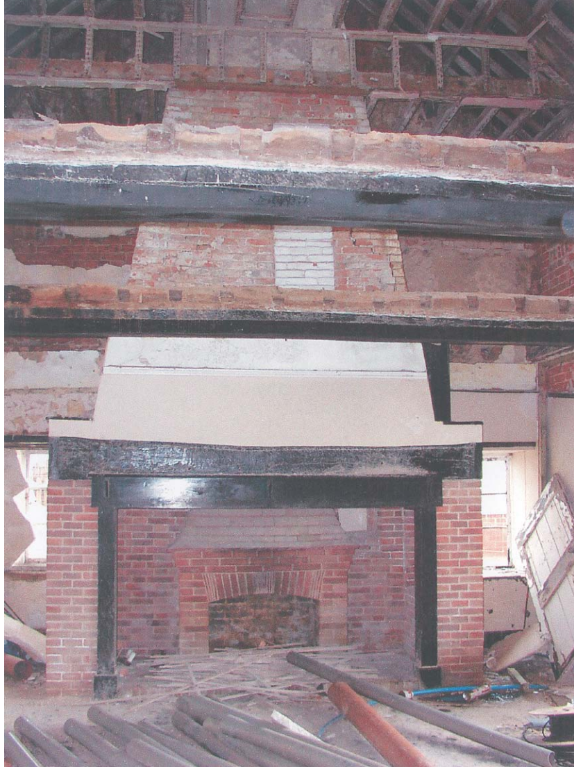
Plate 12 The 20th-century fireplace inside the 18th-century south stack
