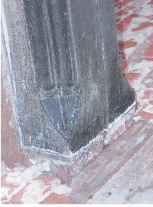
Plate 4 Chamfer and stop on 16th-century beam ('A' on Fig. 4)
