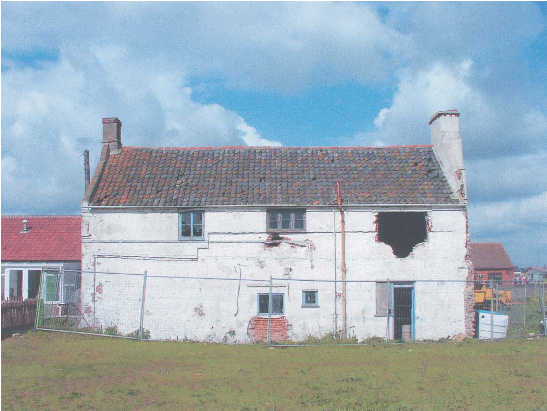
Plate 2 The east elevation
