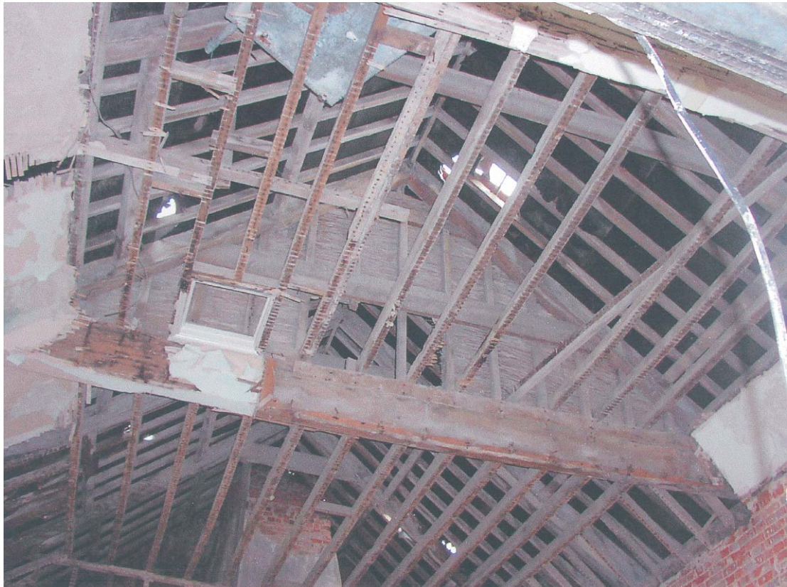
Plate 11 The partition at the attic floor level
