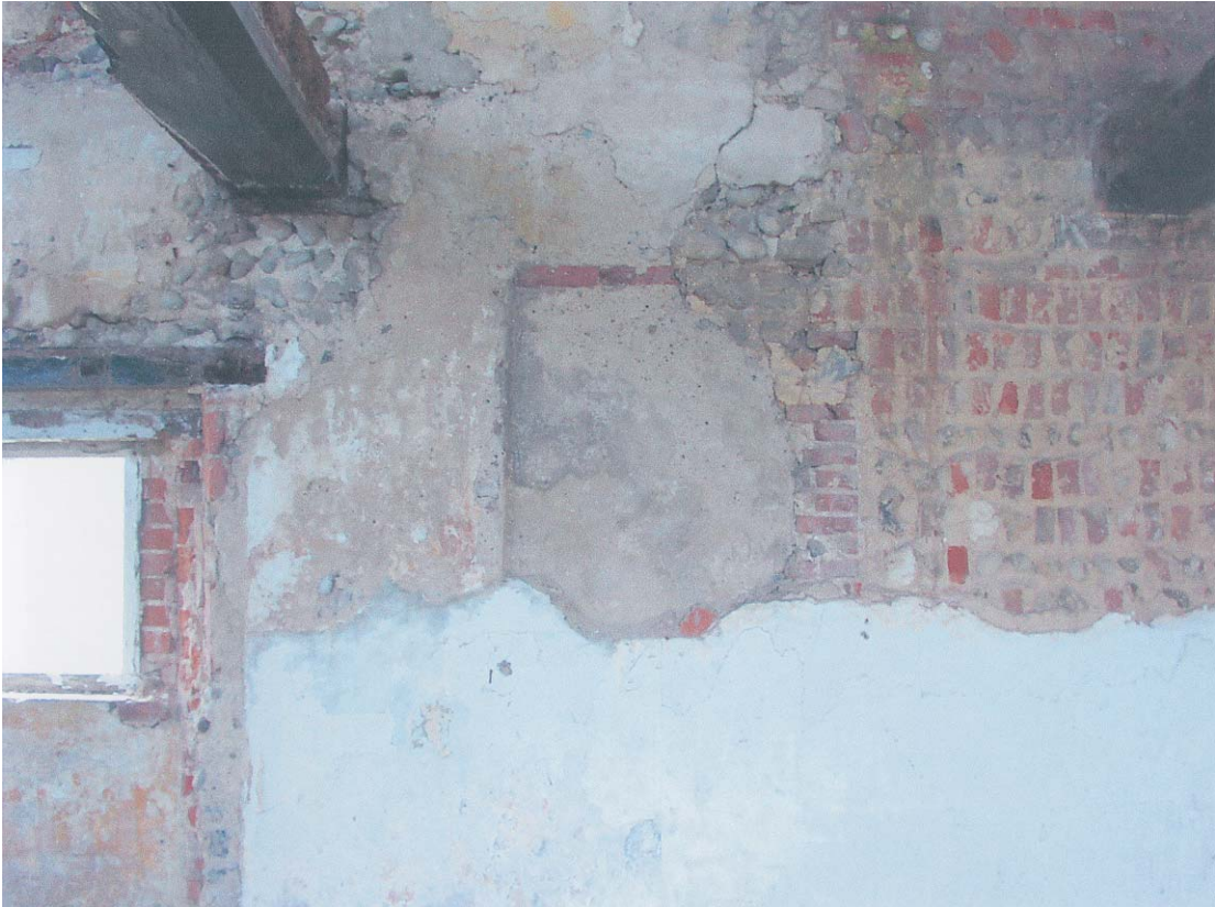
Plate 8 Junction between brick and beach pebble and brick construction
