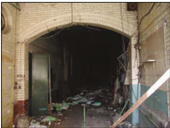
Plate 31: The Electric Lighting Station Gatehouse, Detail of Internal Arch
