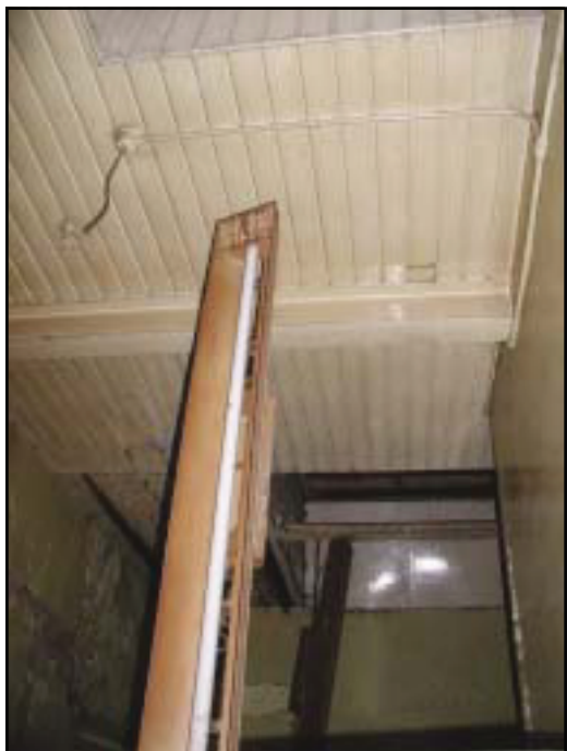
Plate 47: The Electric Lighting Station Gatehouse, Detail of the Roof Underside
