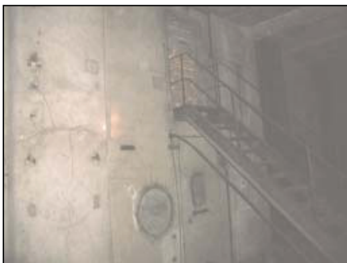
Plate 50: The Electric Lighting Station Gatehouse, Stairs in Switch Room
