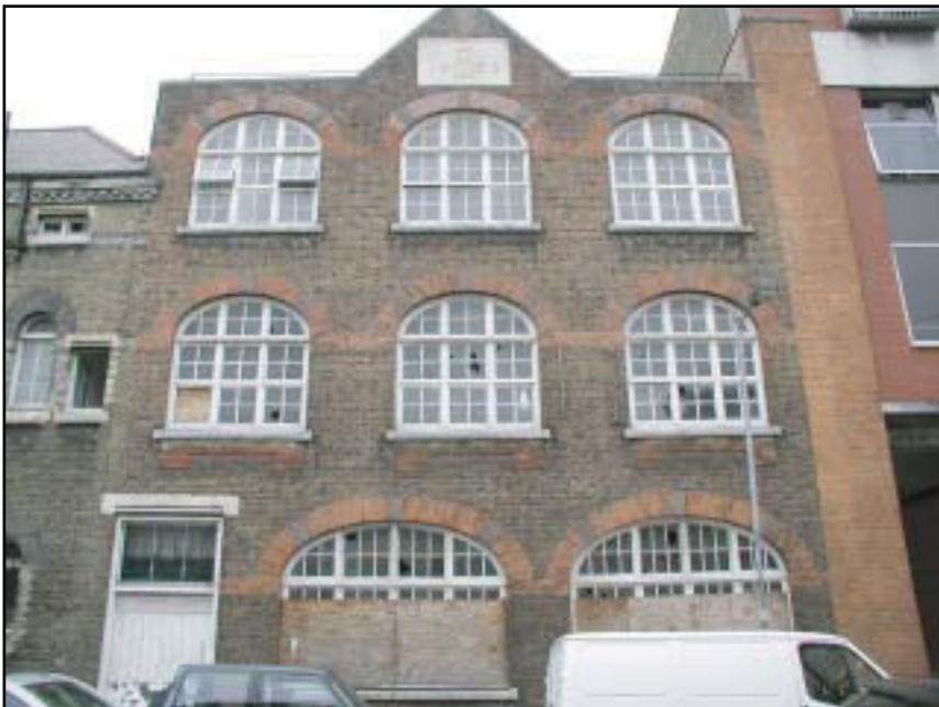
Plate 7: Lady Sion Convent Extension Courtyard
