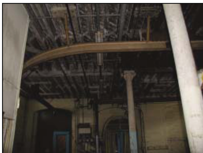
Plate 26: The Star Brush Works, Detail of Ground Floor Goods Hoist
