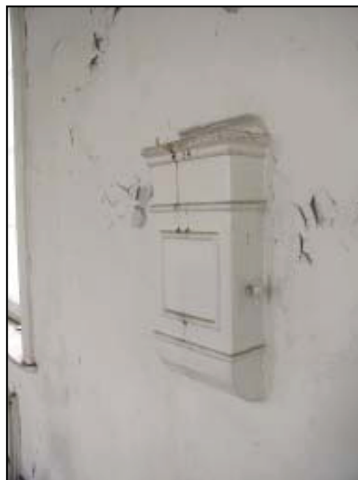
Plate 55: Mount Carmel School, Detail of Dormitory Ventilation Grille
