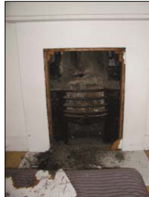
Plate 4: 2 Piper Close, Detail of Fire Place
