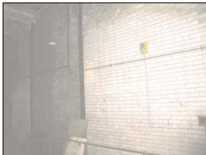
Plate 49: The Electric Lighting Station Gatehouse, Wall in Switch Room
