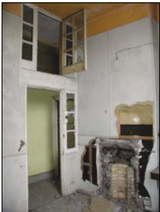
Plate 39: The Electric Lighting Station Gatehouse, Interior View of 1st Floor Office
