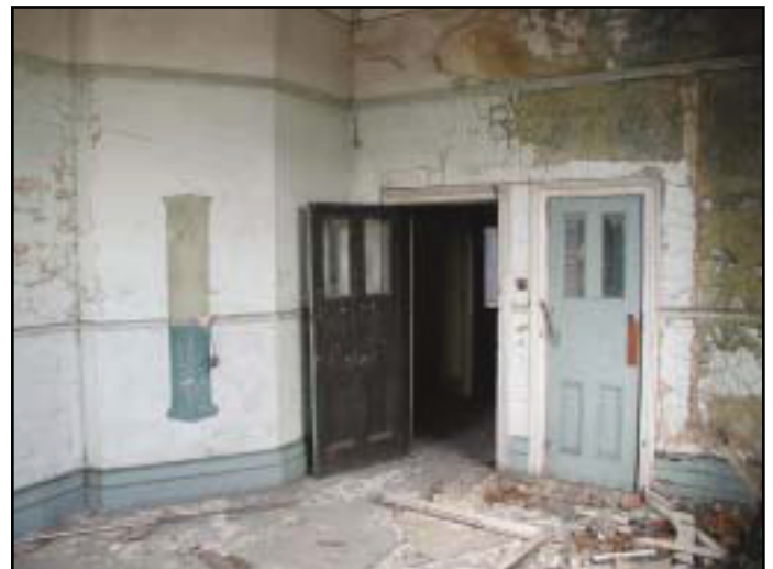
Plate 38: The Electric Lighting Station Gatehouse, Interior View of 1st Floor Corridor and Doors
