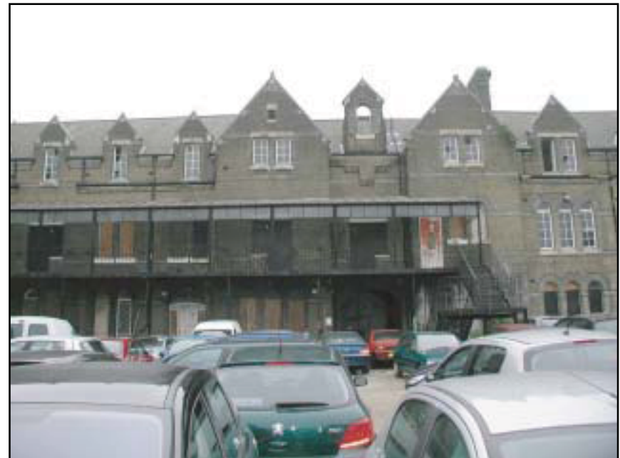
Plate 8: Lady Sion Convent Extension Courtyard
