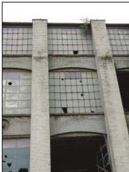
Plate 24: The Star Brush Works, Detail of Original Window Settings and Frames
