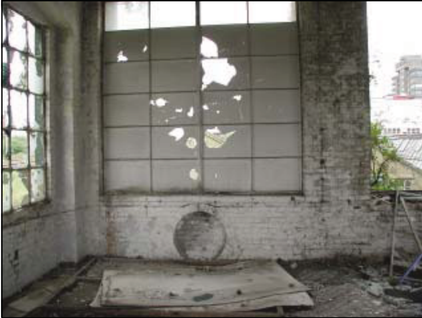
Plate 19: The Star Brush Works, Detail of Windows
