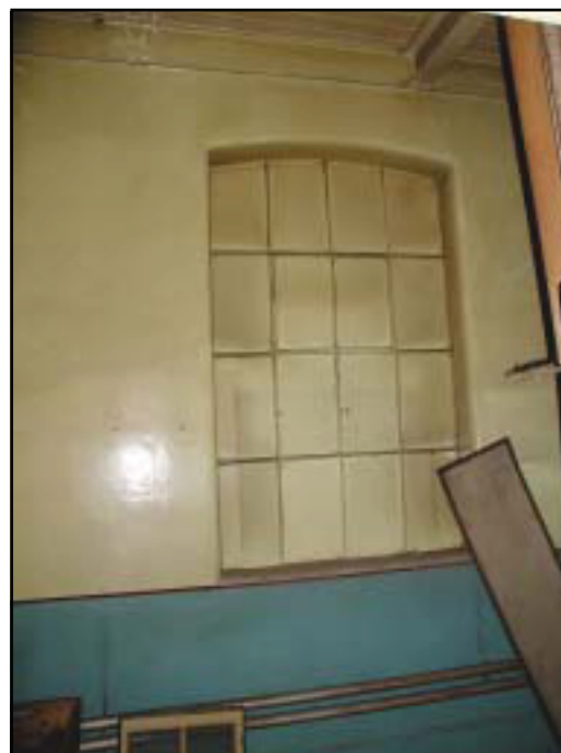
Plate 46: The Electric Lighting Station Gatehouse, Internal Window
