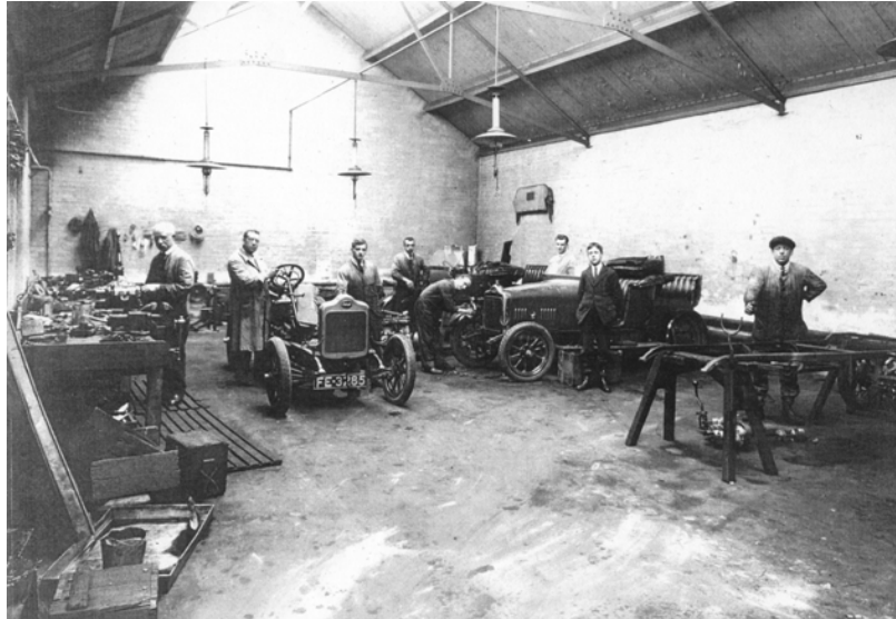
Plate 3: Car assembly in the Calcott Works, 1921 (previously demolished CTM)
