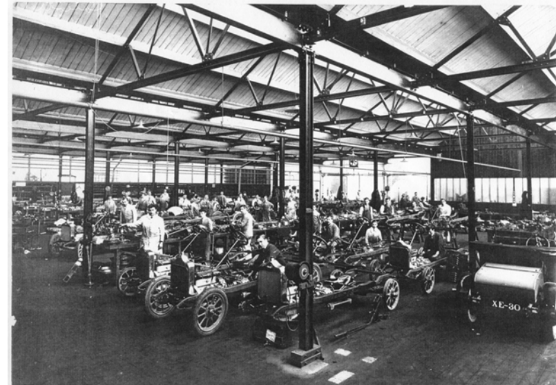
Plate 4: Car assembly in the Calcott Works, 1921 (Building 1c see below - CTM)
