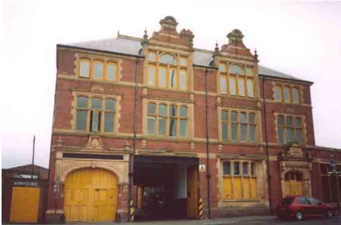
Plate 10: Building 1b (and 2f – left hand side) – Calcott Brothers Office Buildings of 1896 Far Gosford Street frontage
