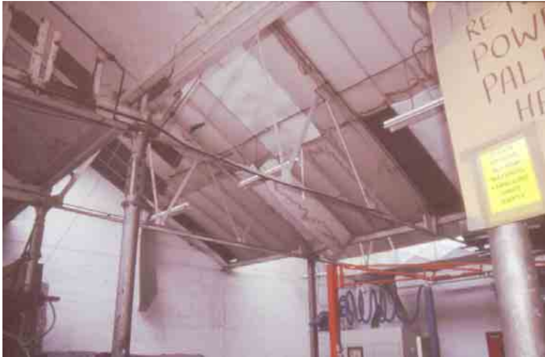
Plate 17: Replaced Roof Trusses (Building 3).
