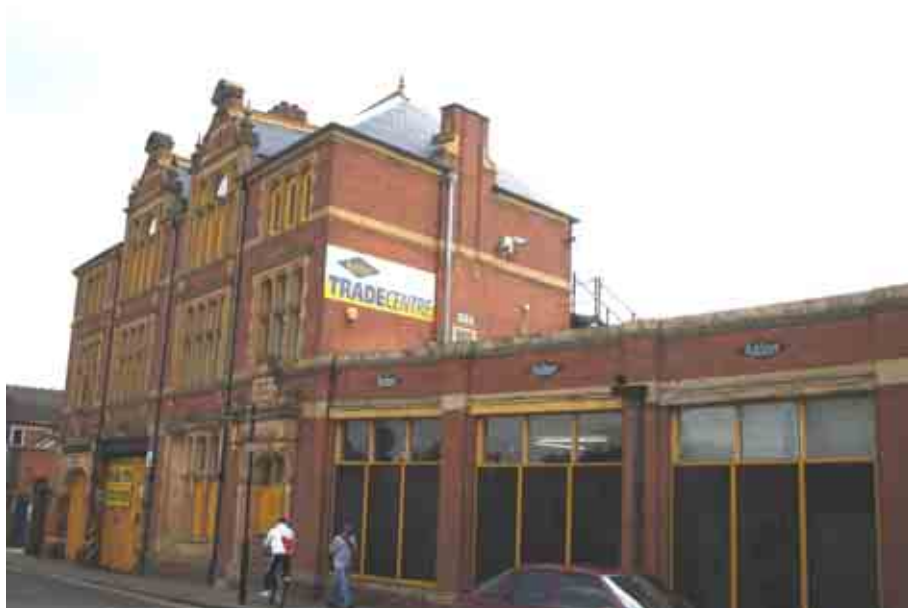
Plate 8: Astley's Far Gosford Street Frontage.
