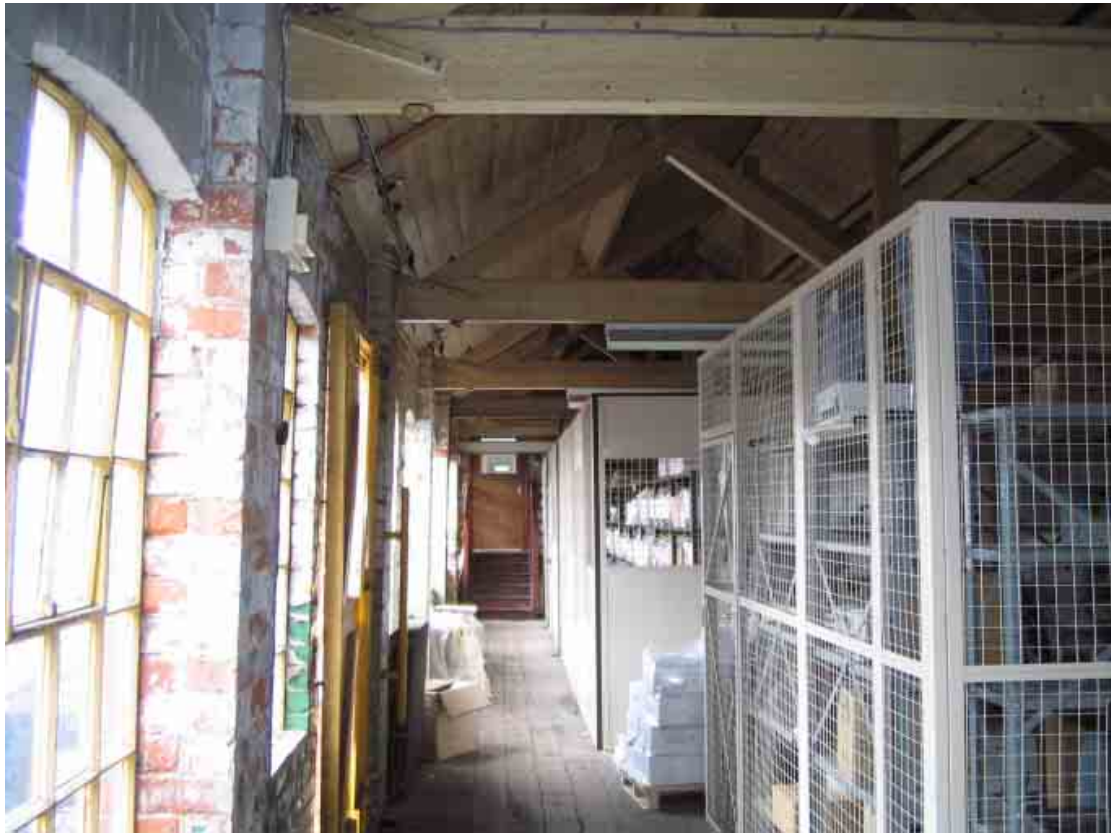
Plate 16: Building 2a , First Floor.
