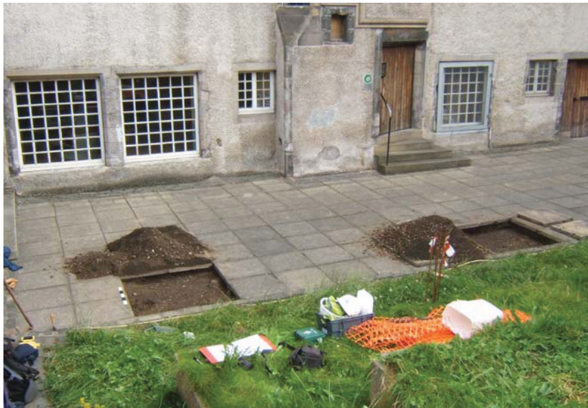
Plate 1: Phase 1 test pits, facing NE with Lamb's House in the background.
