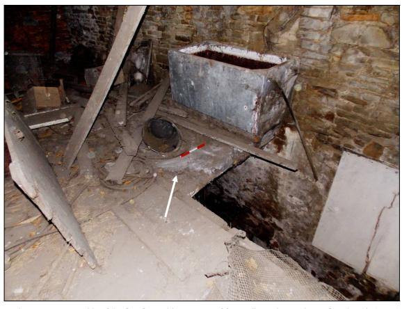
Figure 16: Western side of the first floor with remnants of former lime ash screed over floor boards (arrow)
