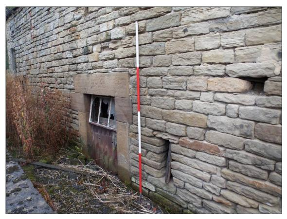
Figure 9: Detail of former doorway and ventilation slit within the south elevation
