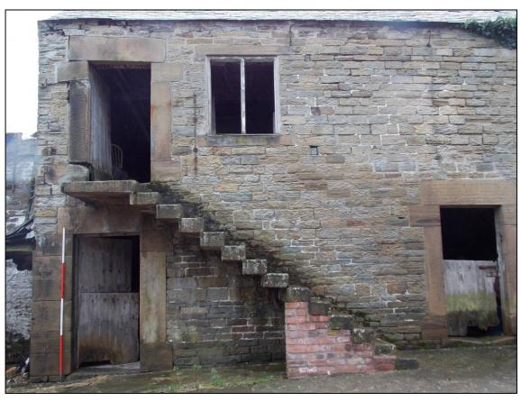
Figure 6: Eastern side of the north elevation with cantilever staircase
