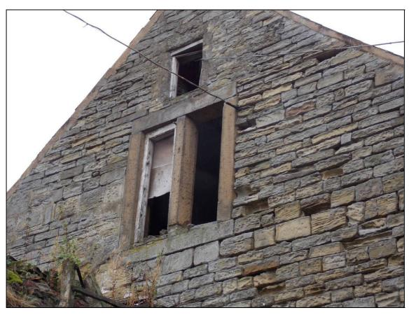
Figure 11: Detail of mullioned window
