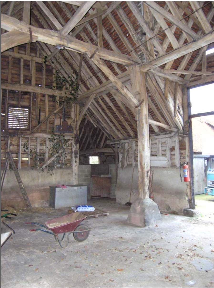
Plate 9 Reused medieval studs in north east frame and removed north corner
