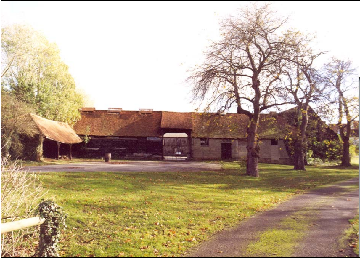
Plate 11 Front range from driveway with Cartlodge 7 to left
