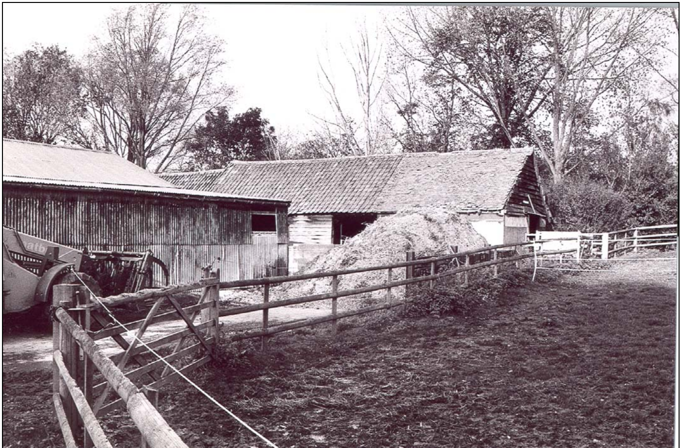
Plate 20 Loose Box 6 and Cowshed 9 viewed from paddock south-east
