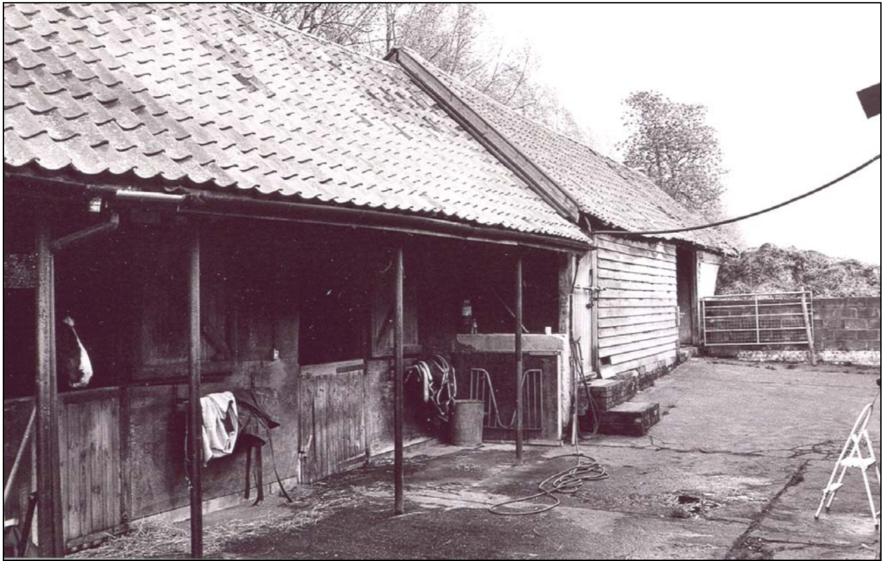
Plate 19 Stables 5 and Loose Box 6 viewed from west
