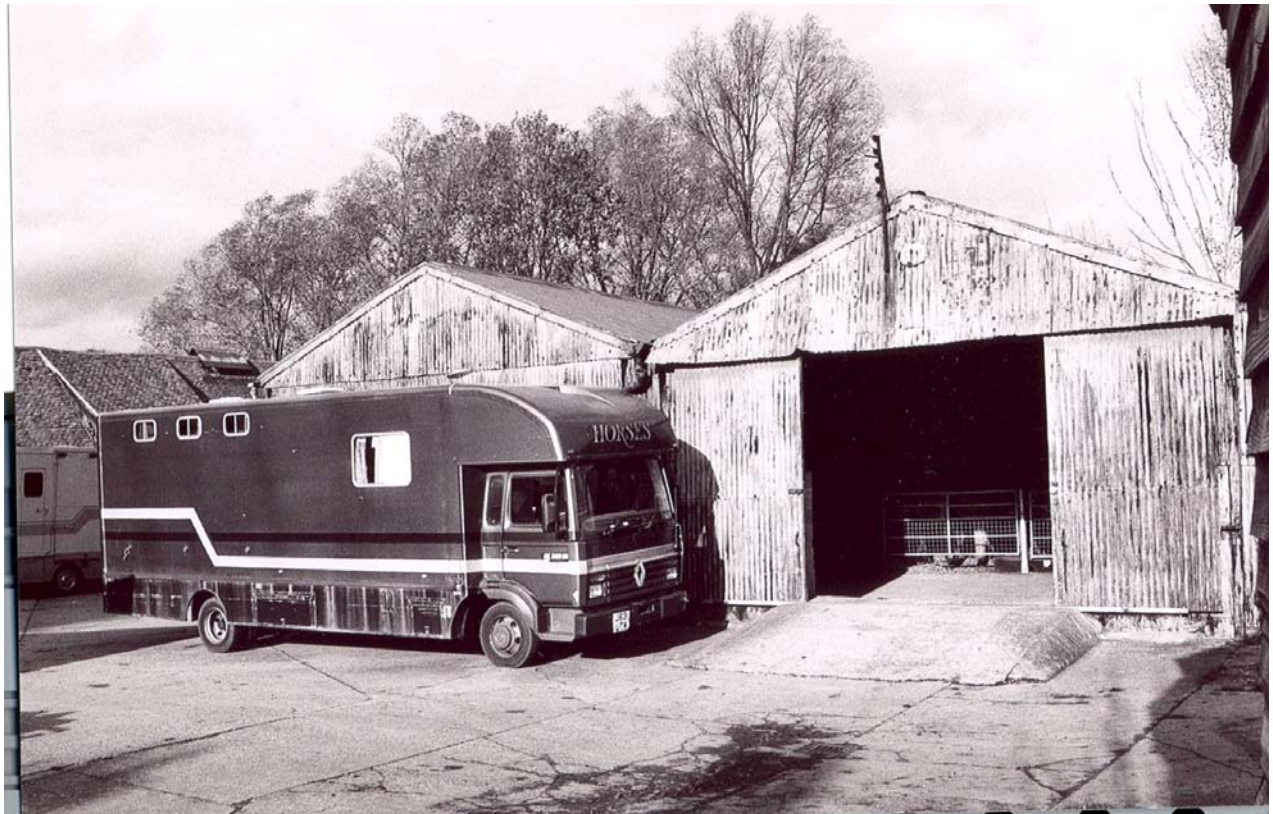
Plate 26 Cowshed 9 viewed from south
