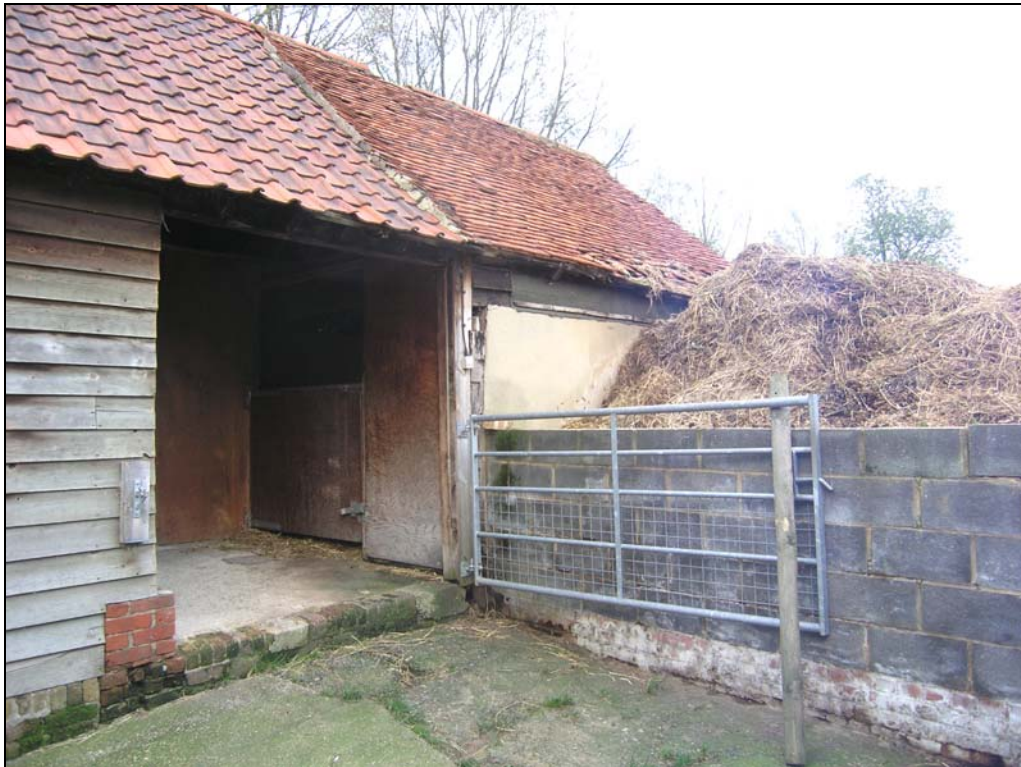
Plate 21 Inserted door into Loose Box 6 and plinth wall to late 19th-century south-east range
