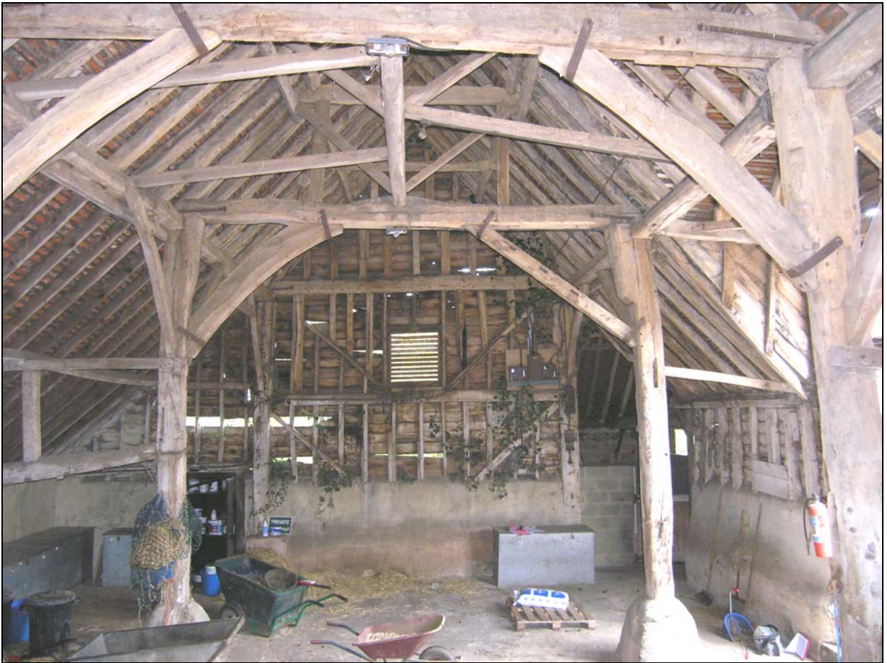
Plate 5 Interior of Barn 1 viewed to north-east end
