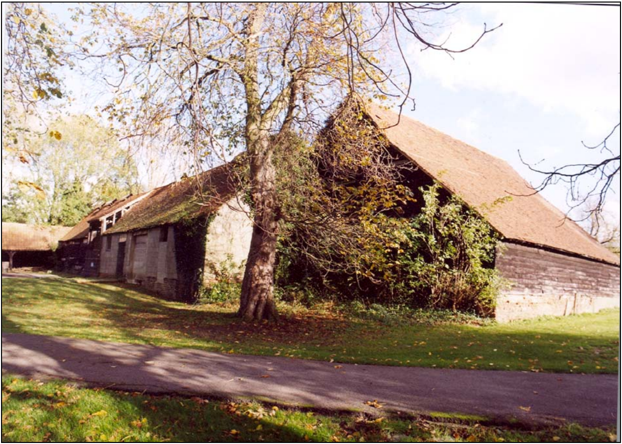
Plate 3 Rear of Barn 1 and front range viewed from south-west
