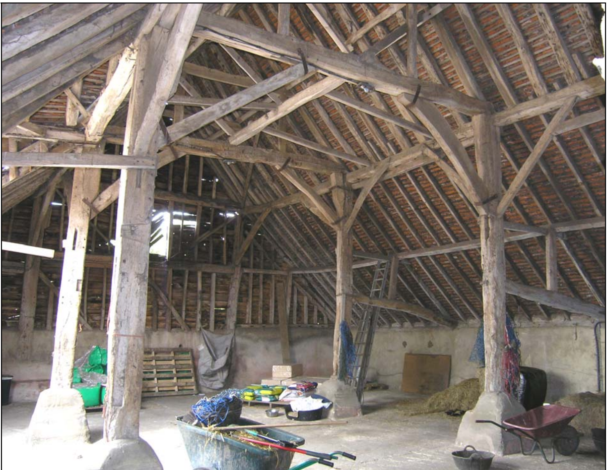
Plate 4 Interior of Barn 1 viewed from north
