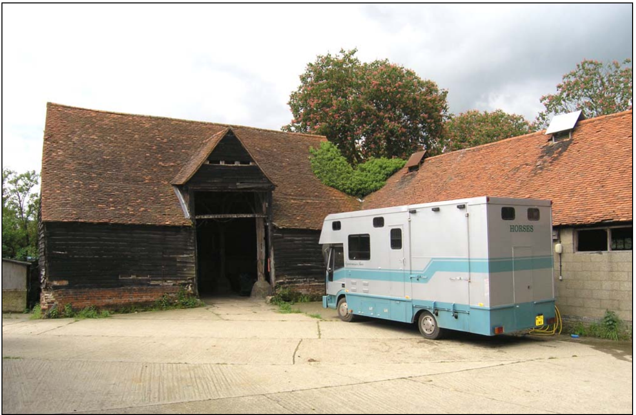
Plate 1 Barn 1 and Stock House 2 in north corner of yard
