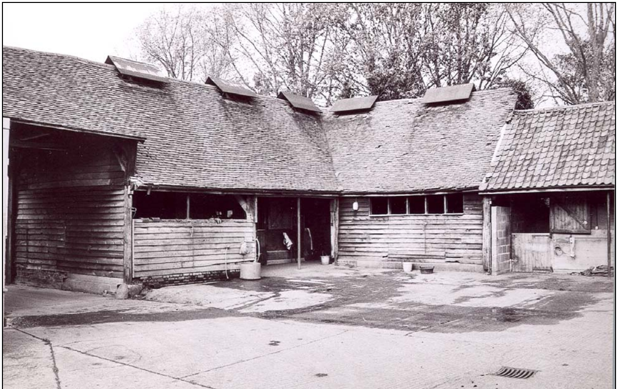
Plate 16 Stables 4 viewed from south, inside yard
