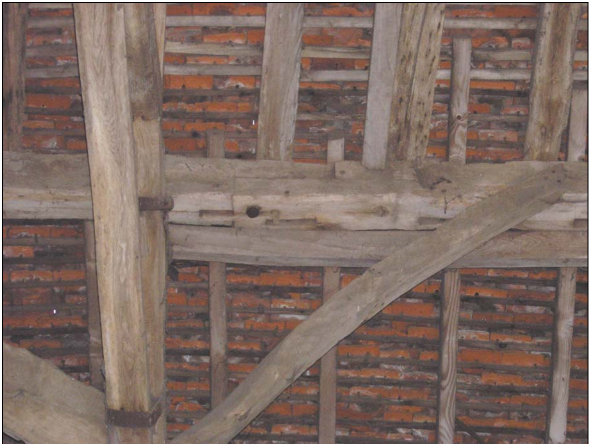
Plate 6 Archaic bridle scarf joint in south-west arcade plate
