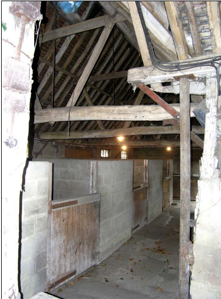
Plate 14 Interior of Stock House 2 showing sawn off wall plate and weatherboarding to Barn 1
