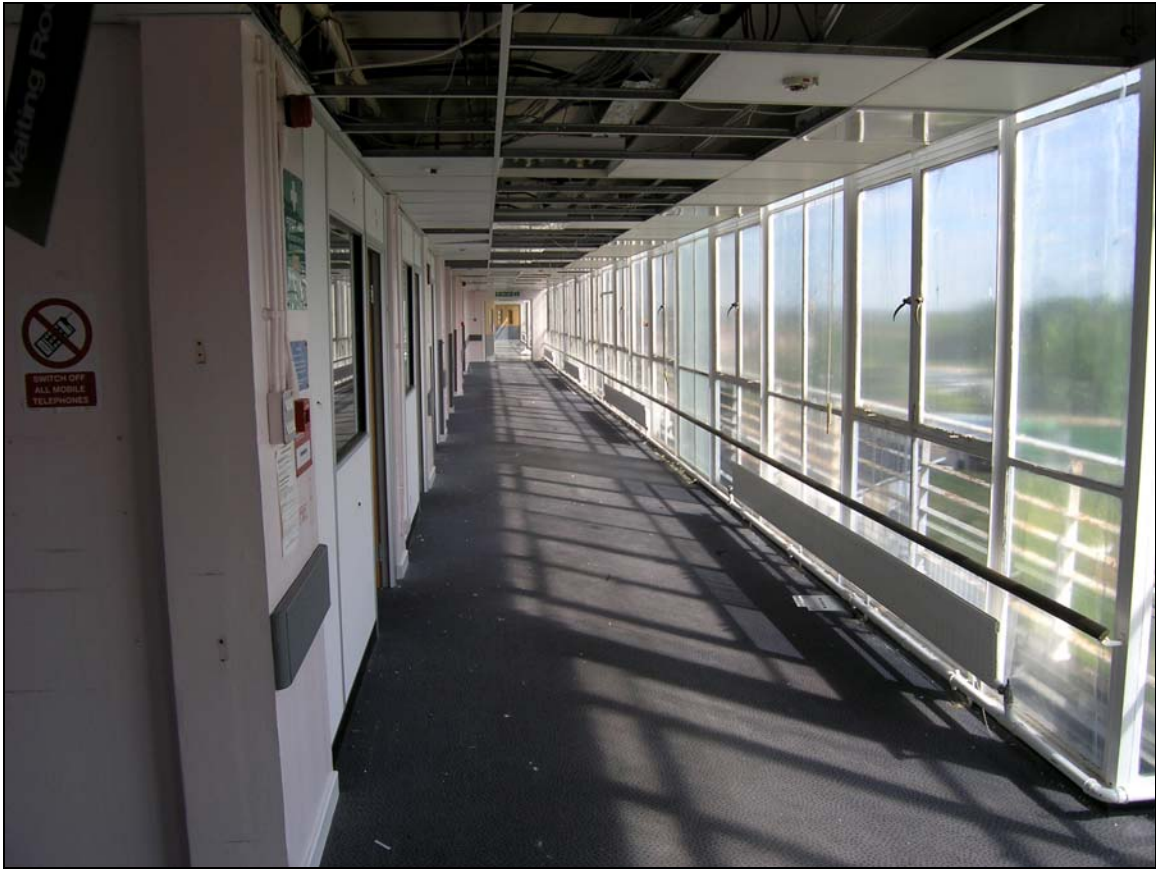
Plate 13 Second floor viewed from west, middle section
