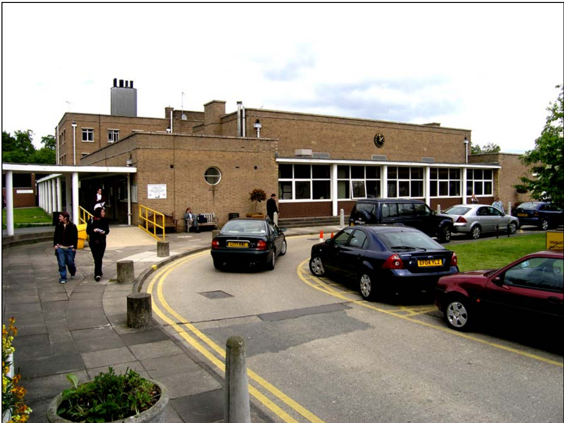
Plate 28 Cafeteria (4) main façade with colonnade to left
