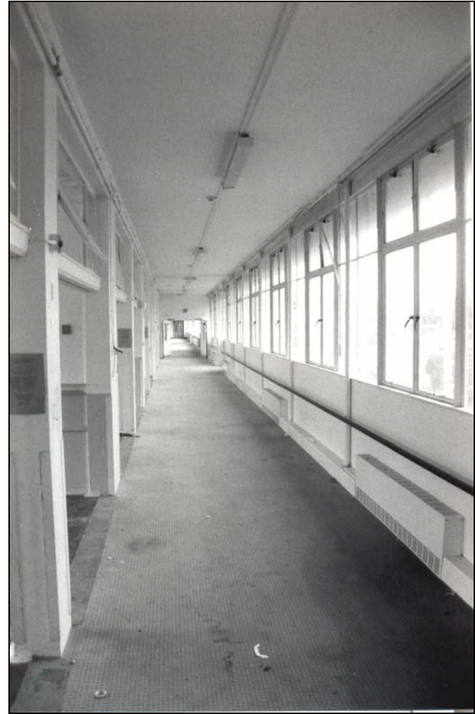
Plate 6 Ward B10 (ground floor) viewed from west
