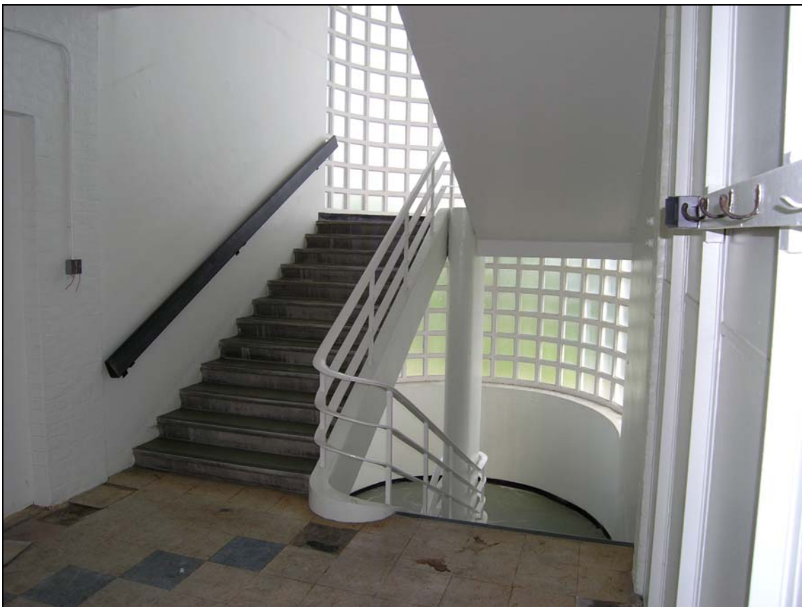
Plate 18 Stairs on first floor level, showing later vinyl handrail
