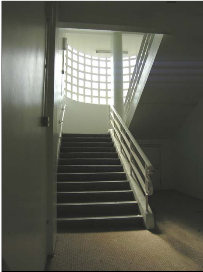
Plate 17 Tubular steel stair rail fixture on ground floor
