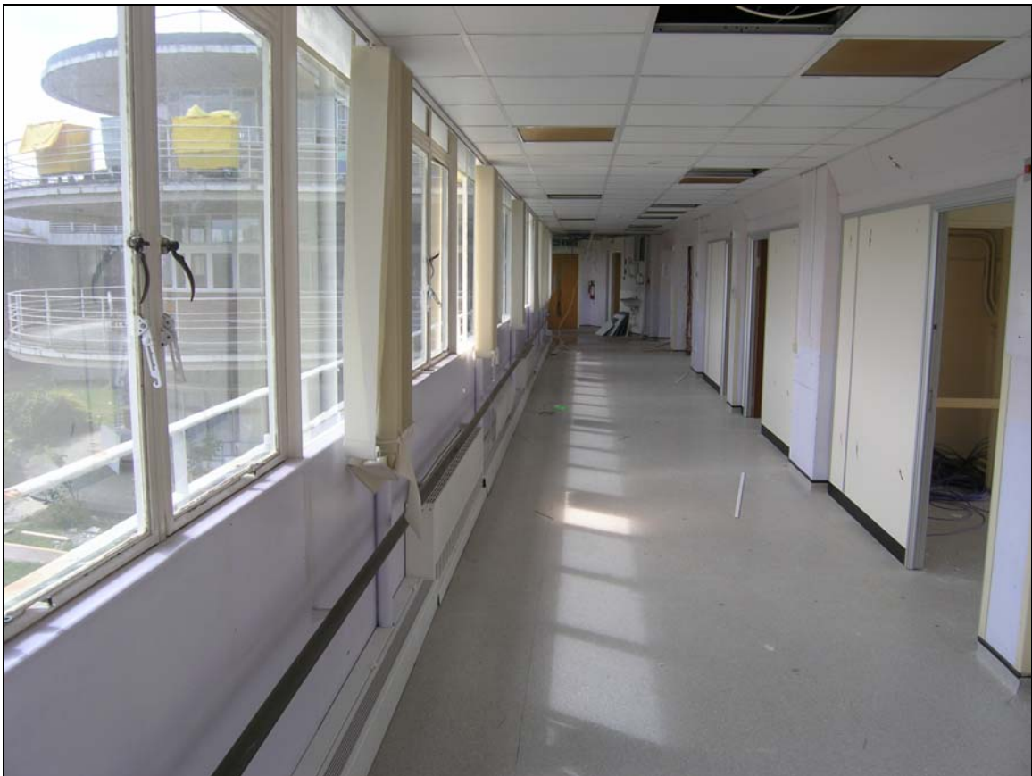
Plate 10 Ward B12 (first floor) viewed from east
