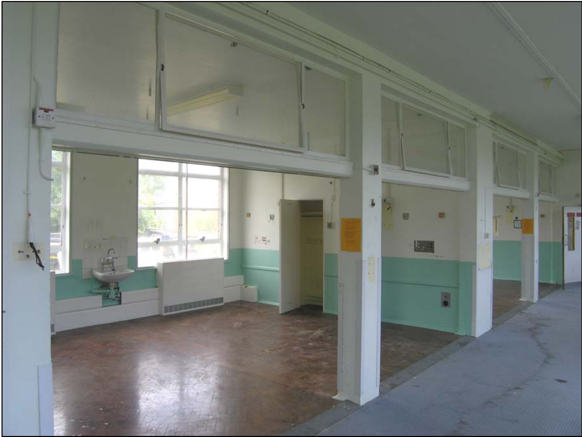
Plate 7 Typical four-bed cubicle in ward B10 showing 'Korkoid' floor
