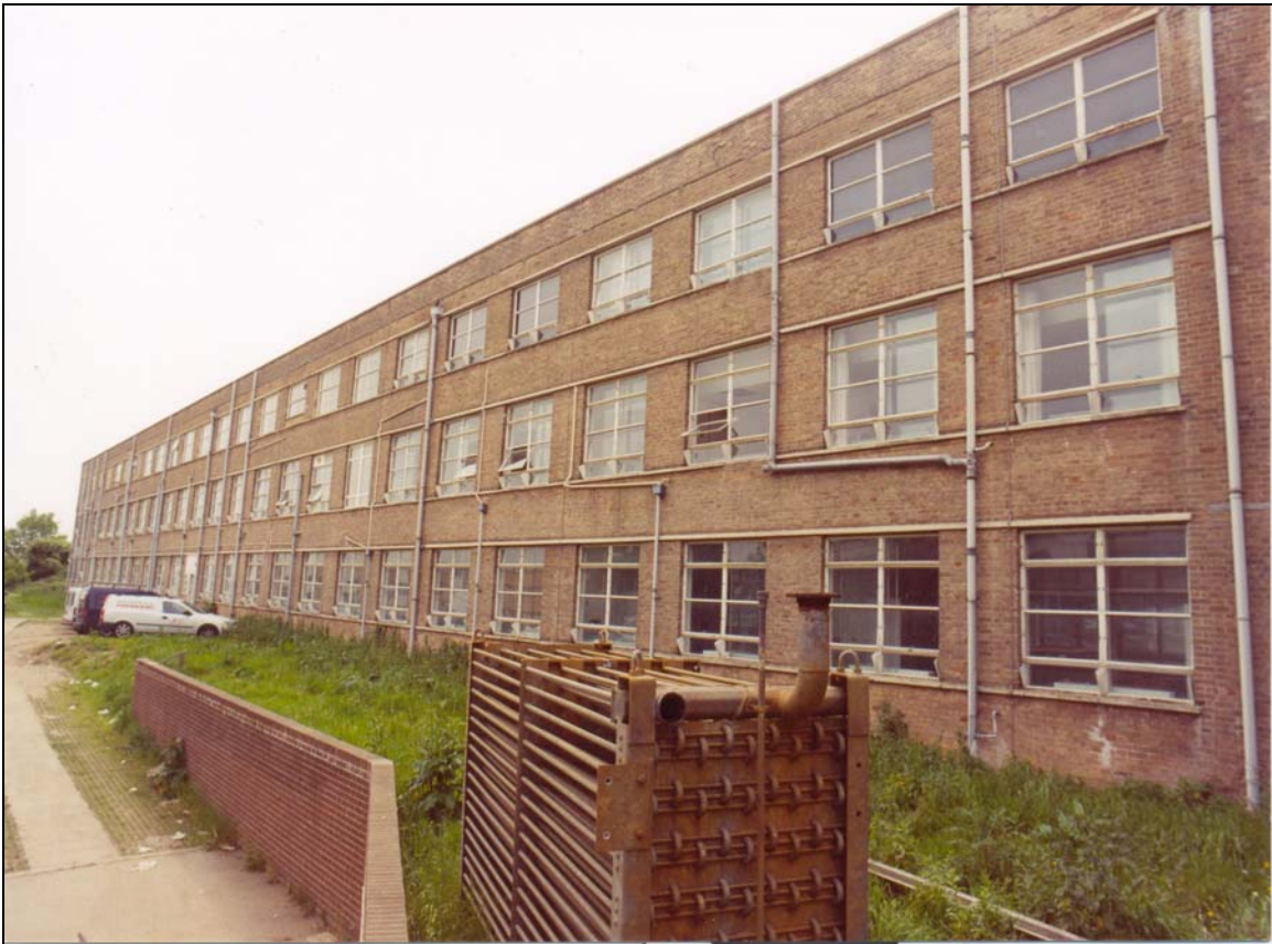
Plate 4 North elevation of east wing, viewed from north-west
