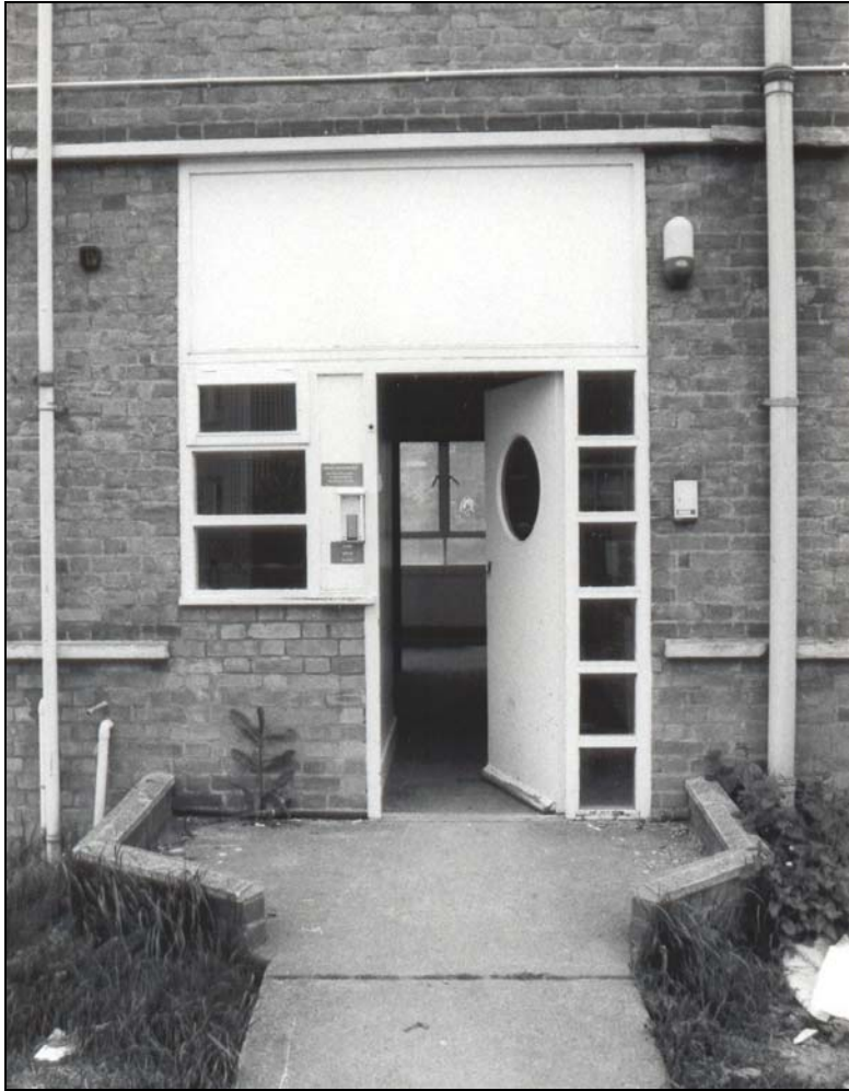
Plate 5 North entrance to east wing
