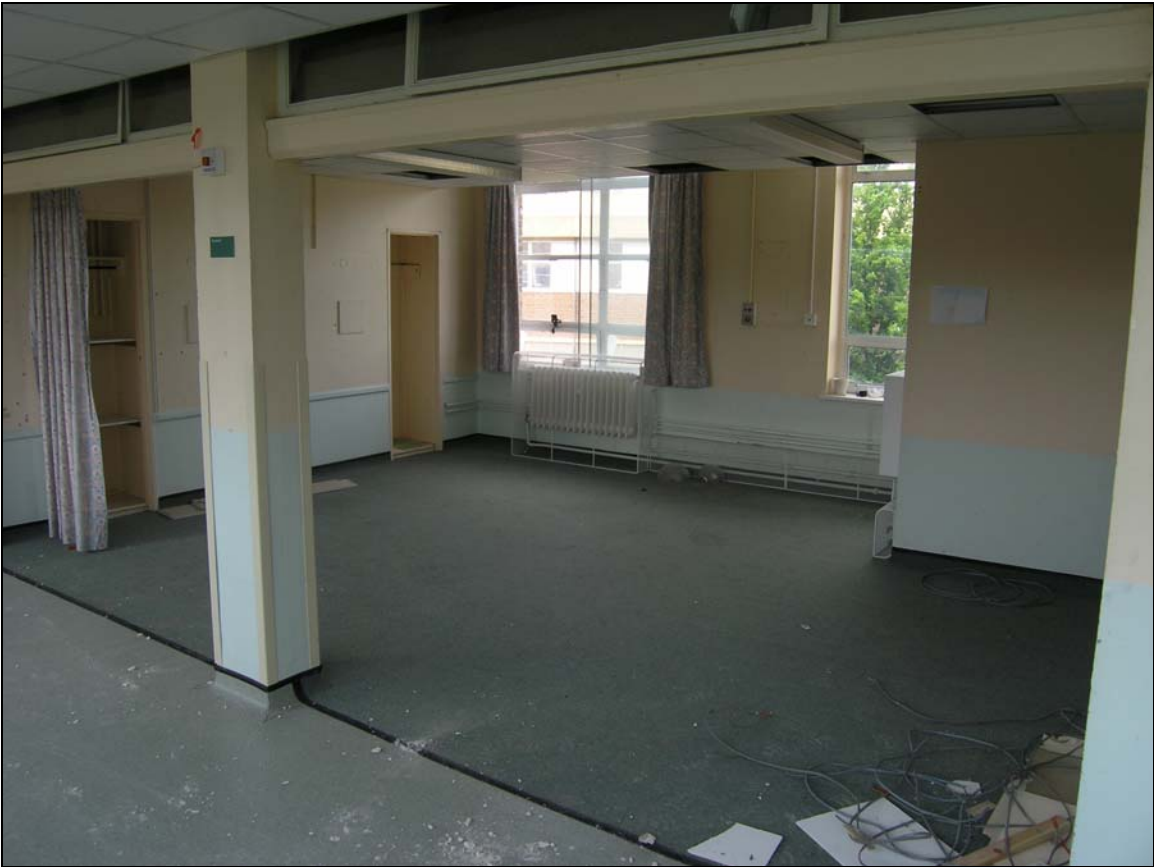
Plate 12 Typical four-bed cubicle on Ward B13 (first floor)
