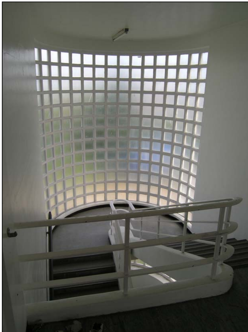
Plate 16 Glazed stair turret and stairs from second floor
