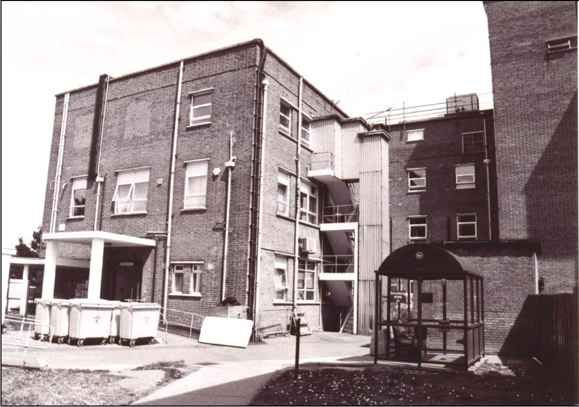
Plate 25 Treatment block (3) east elevation
