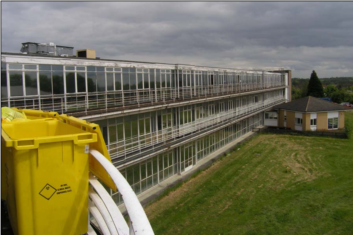
Plate 1 South elevation viewed from east sun-ward
