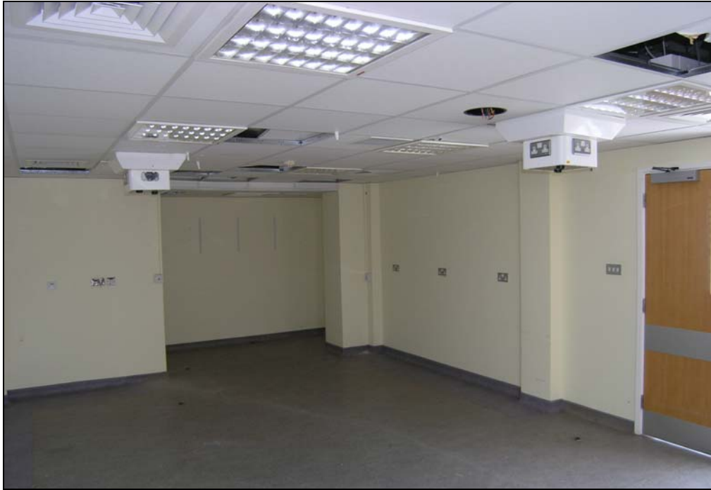
Plate 15 Stripped-out operating theatre on second floor
