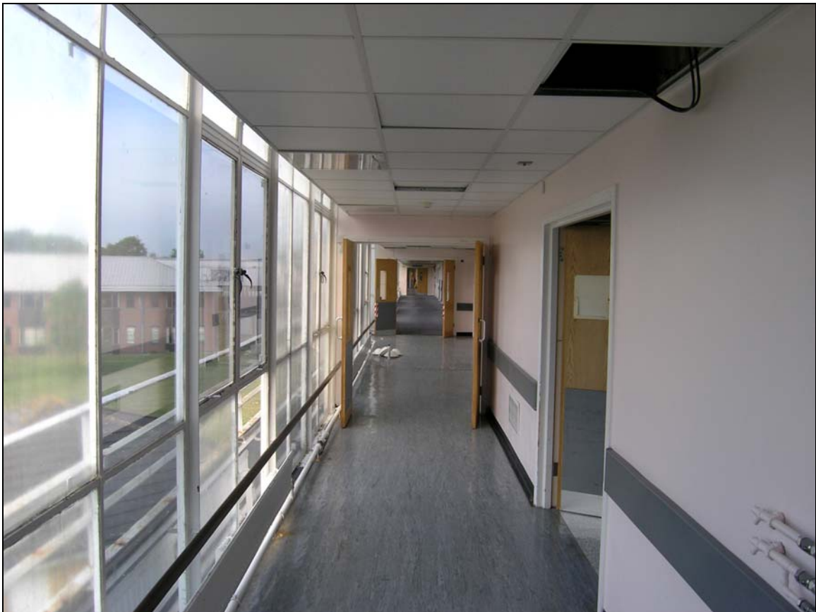
Plate 14 Second floor viewed from east
