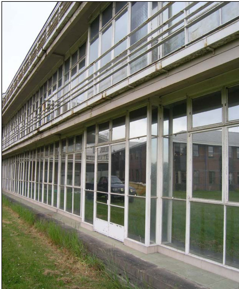
Plate 2 Detail of glazing on south elevation
