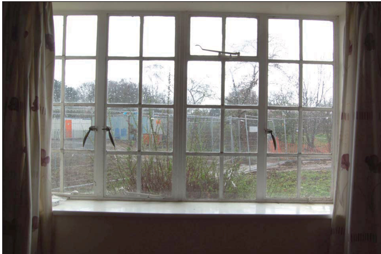
Plate 20 Typical later Crittalls window fixtures in Block F
