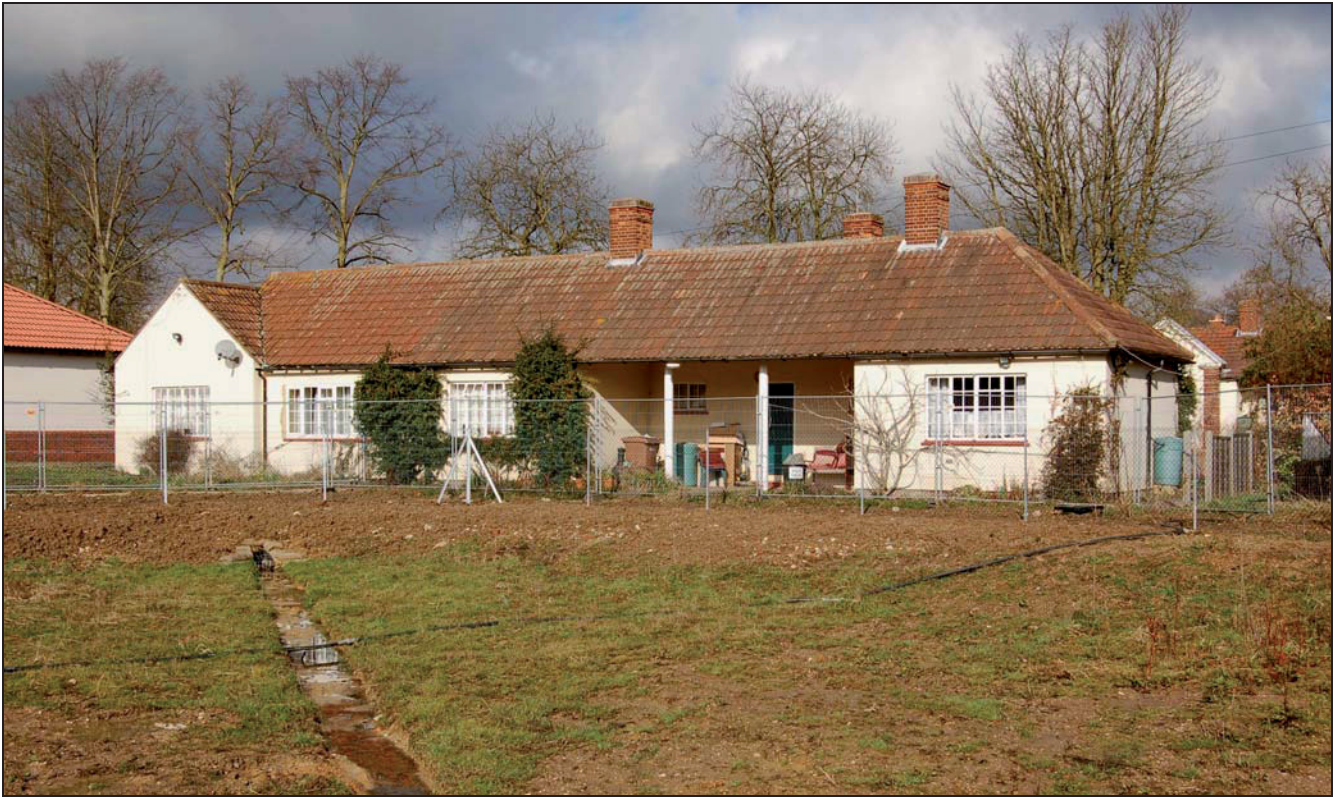
Plate 17 South elevation of Block F
