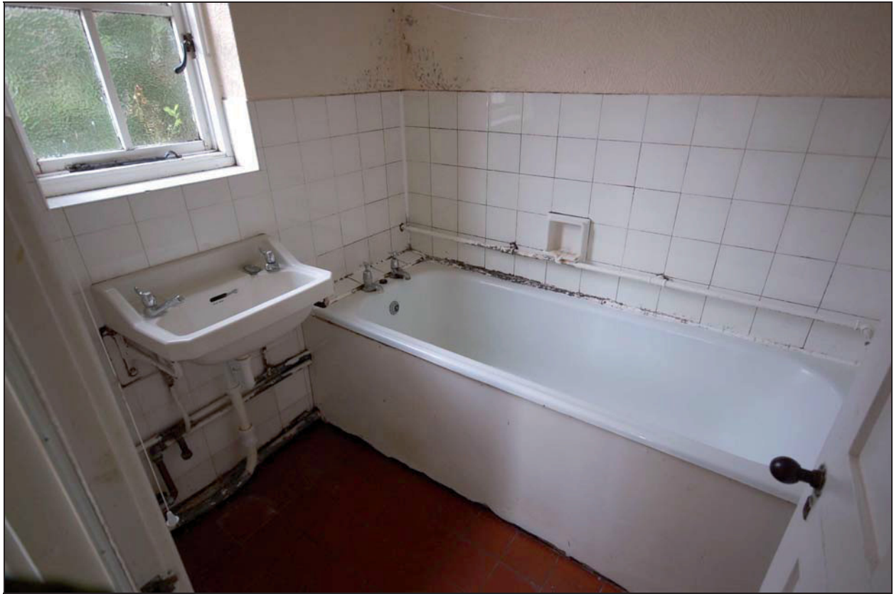
Plate 15 Original bathroom fixtures inside Block C (flat 13)
