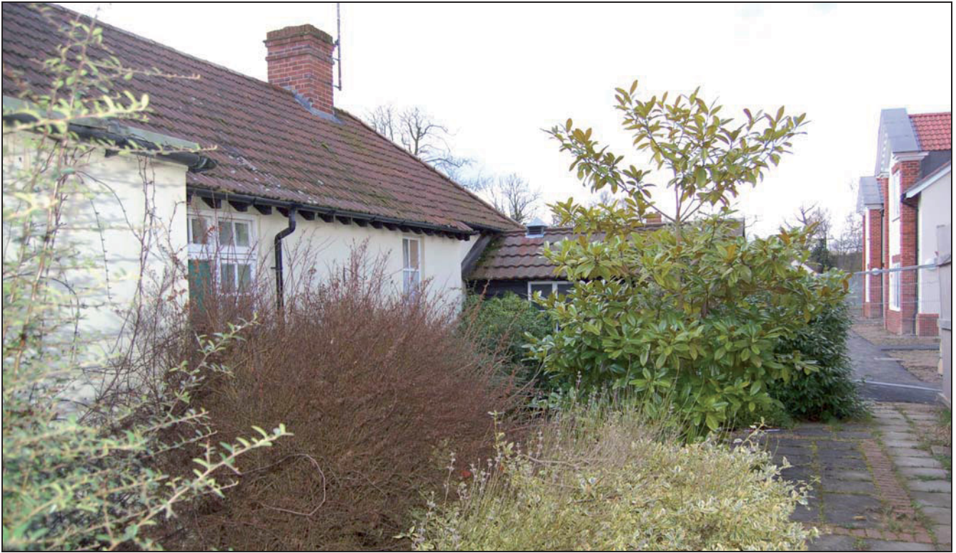
Plate 11 Chapel to rear of Block C
