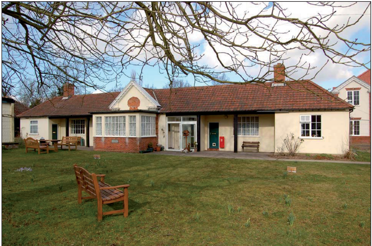
Plate 2 Block A main façade (south)
