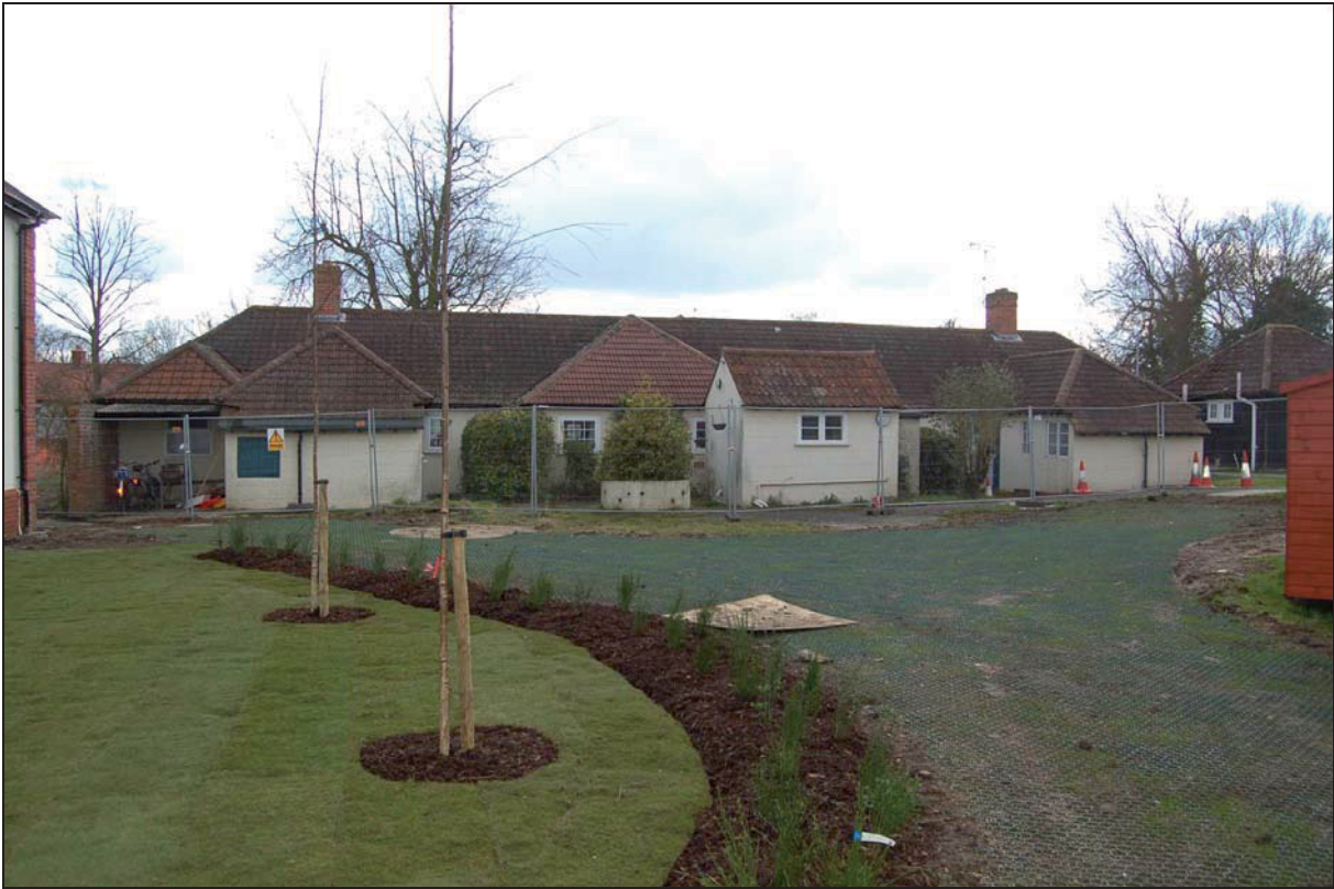
Plate 3 Rear elevation of Block A with guest chalet to right
