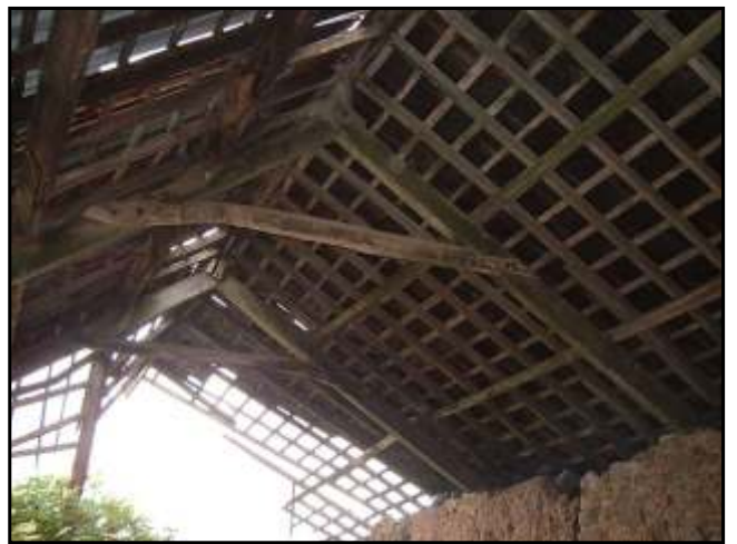
Plate 6 The surviving A-frame roof trusses within the ruined cattle shed.
