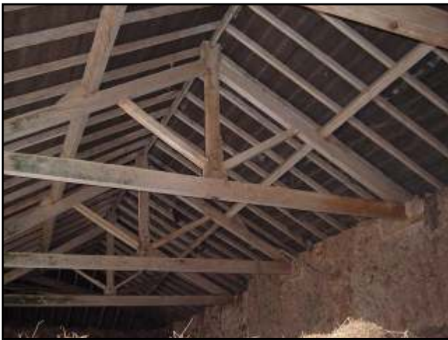
Plate 3 Tie-beam trusses with kingposts in the linhay.
