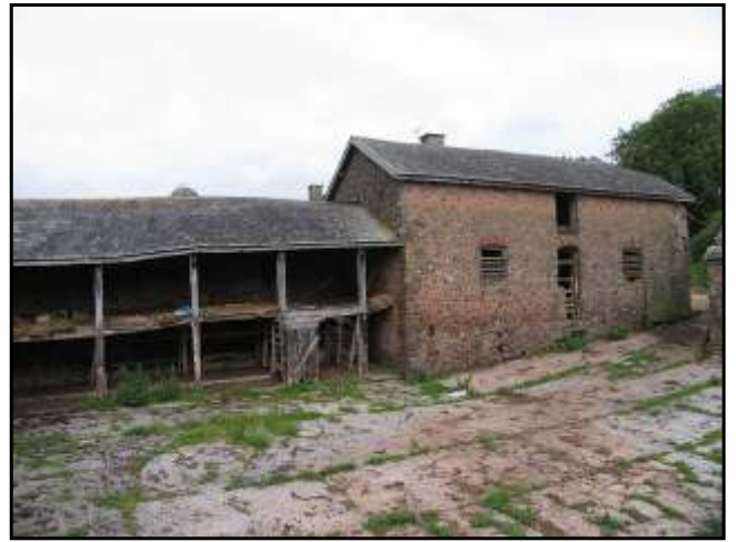
Plate 2 Eastern end of the stable and adjoining linhay on the left.
