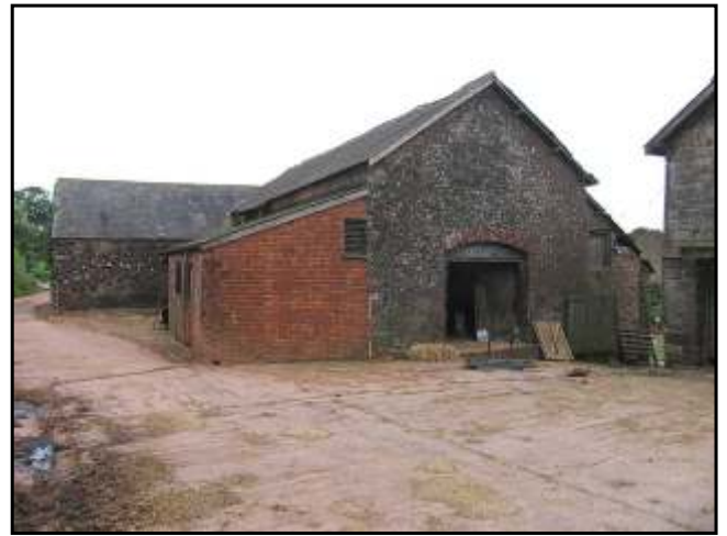
Plate 4 Threshing barn with appendages - late looseboxes on the left, with mill building beyond and another lean-to to the right.
