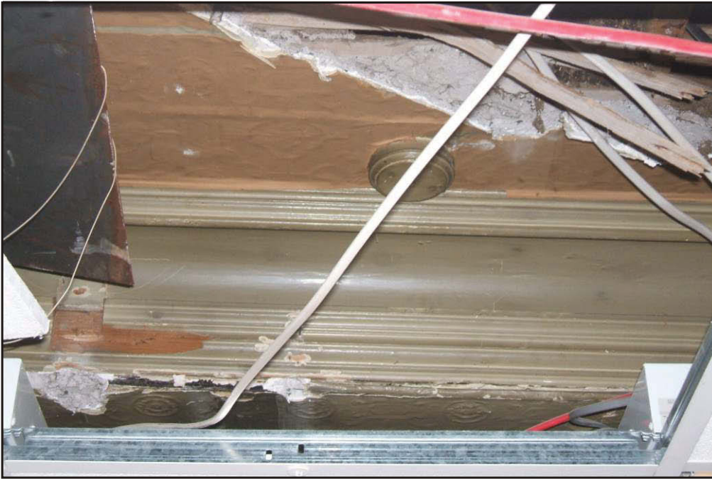
Plate 1 Ground-floor front room showing cornice above modern suspended ceiling, looking northwest.
