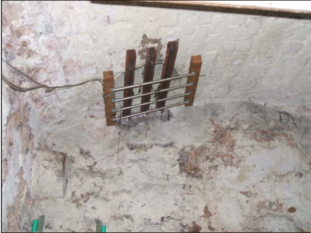
Plate 3 Basement brick vault in rear store, looking northwest.
