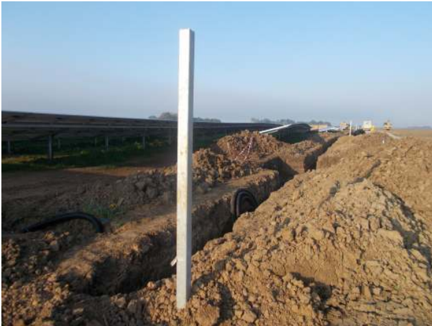
DP 1. Service trench, east end. Looking west.
