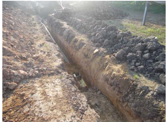
DP 4. Service trench, central part. Looking south-east.
