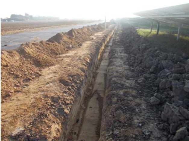
DP 5. Service trench, east end. Looking east-south-east.
