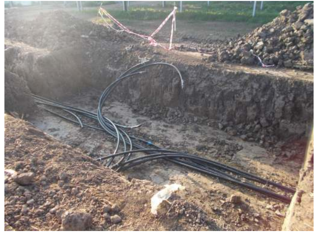
DP 2. Service trench, west end. Looking south.
