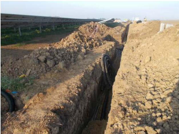
DP 3. Service trench, central part. Looking west.
