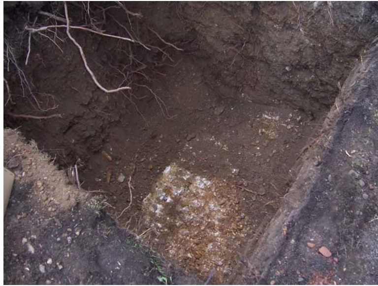
Plate 5: Area 4, excavations for gate pier foundation
