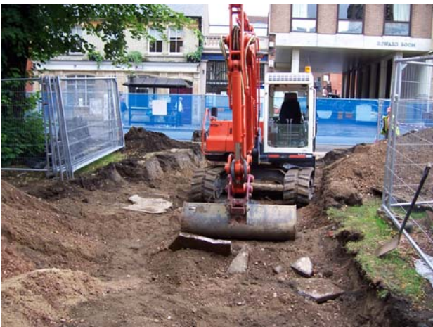
Plate 3: Area 3, removal of overburden prior to the construction of new driveway
