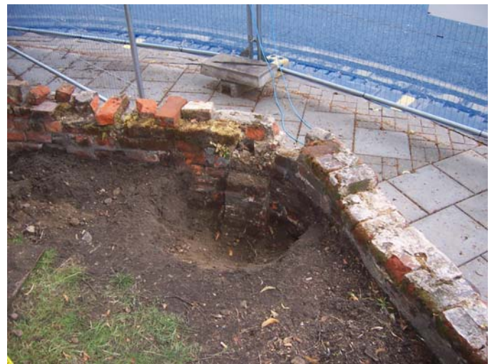
Plate 7: Area 5, excavation of pier against the north churchyard wall
