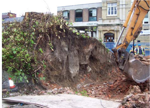
Plate 2: Area 2, during the removal of the earth mound
