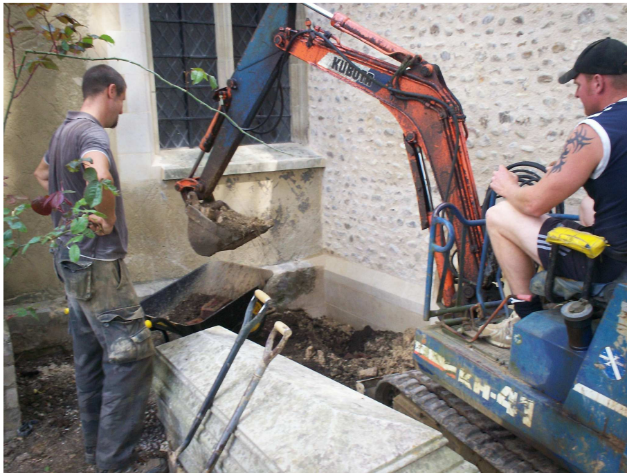
Plate 1: Excavation of trench adjacent to the porch
