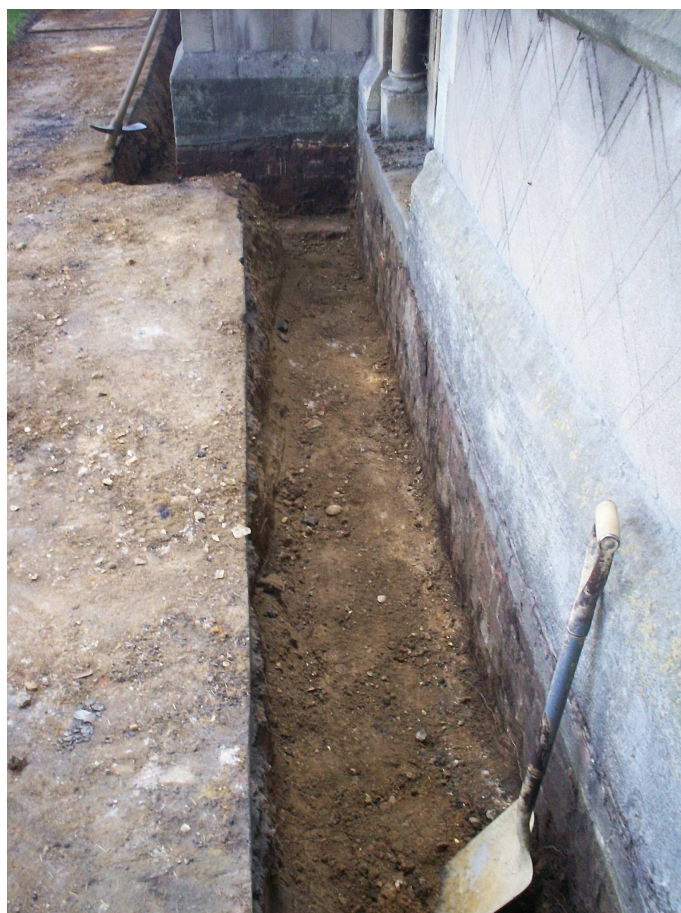
Plate 2: Excavated trench adjacent to chapel
