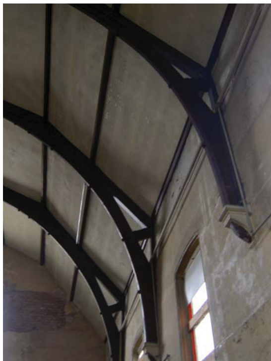
Plate 18: Ends of the trusses supported on corbels
