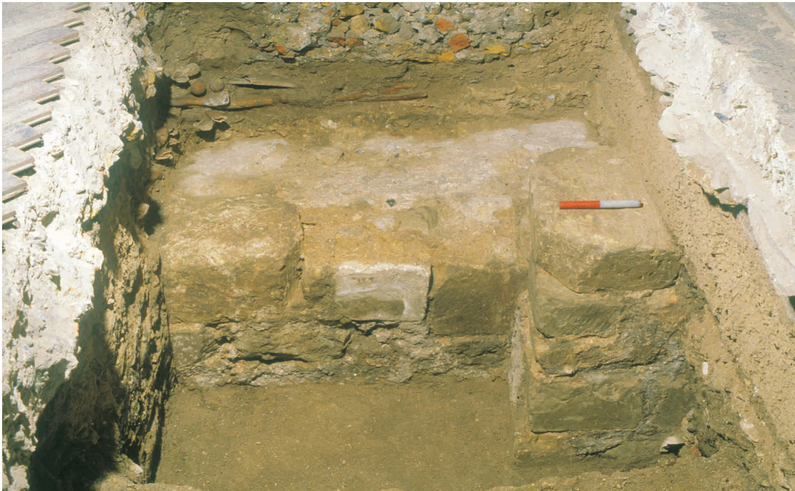
Fig 10 Photograph of the foundations [18] and [22], looking south, TP2
