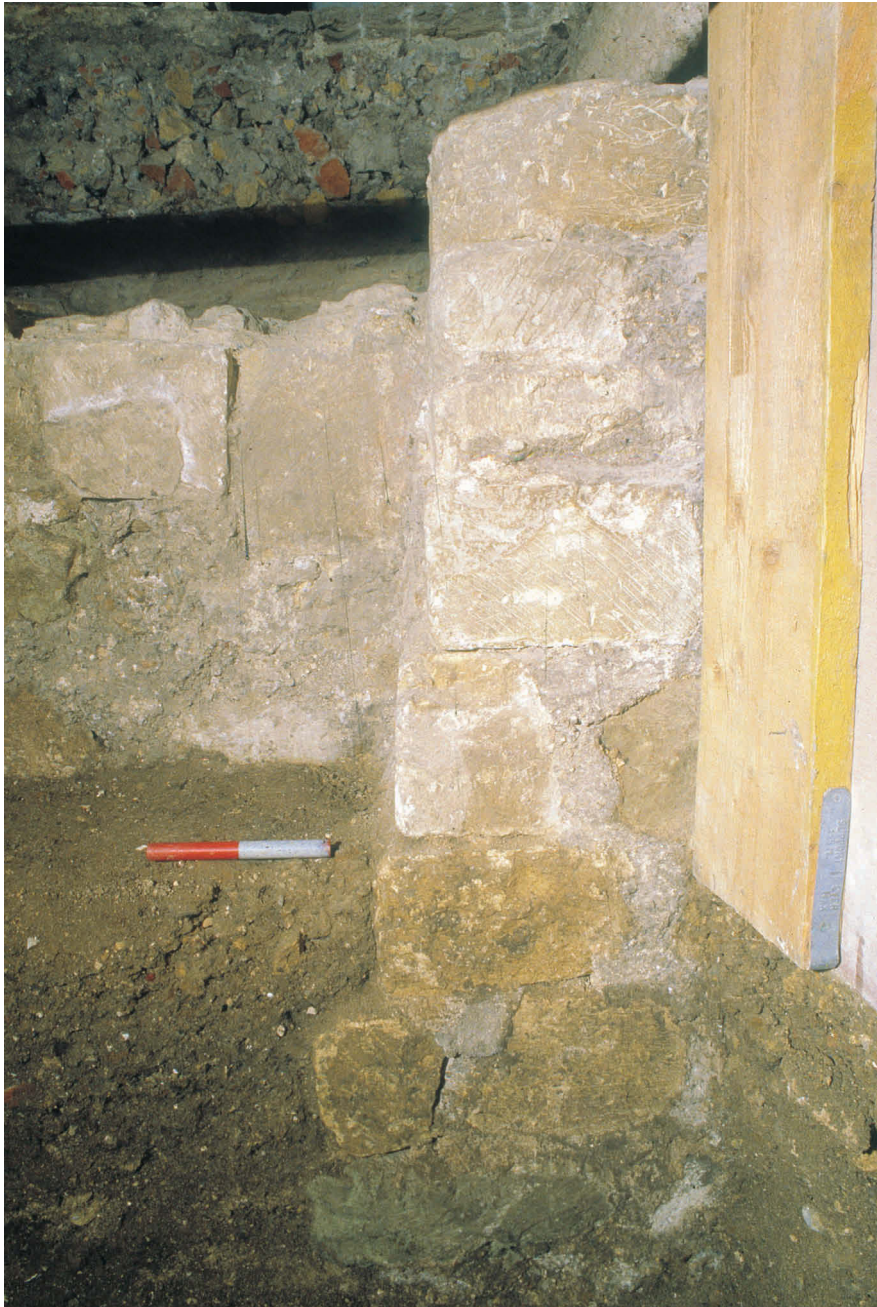
Fig 11 Photograph of foundations [18] and [22], after full depth of excavation, TP2
