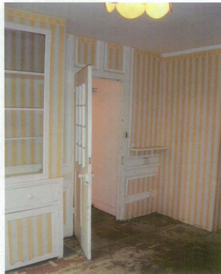
Fig 37 High-quality panelling [15] inserted to form a new west wall in the former kitchen, dividing B16 from a passage beyond, B17; looking north-west. The panelling is too large for its present position and was perhaps taken from elsewhere in the house. The dado rail has been shaved to allow the glass-panelled door to swing flat against this wall, suggesting that the dresser was added to the wall later (A J Browne, Architects)
