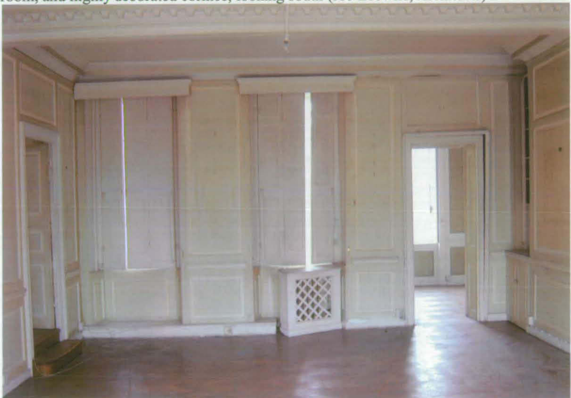
Fig 41 Northern half of 1F6, showing second of two chimney breasts and fireplaces in this room, RSJ running from west to east across the ceiling, decoratively boxed, and a different form of cornice from that in the southern half of the room; looking north, with 1F7, a small room in the east rear wing, beyond (A J Browne, Architects)
