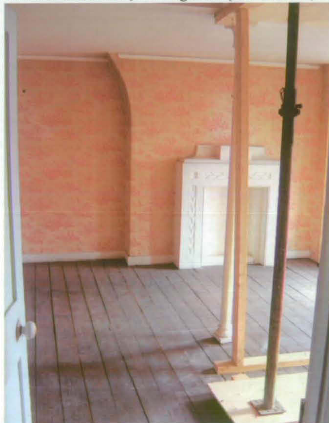
Fig 45 Fire surround in 3F5 and steel column inserted, probably after the north wall of this room was moved northwards; looking east. The steel column has been reinforced recently with acrow props (A J Browne, Architects)
