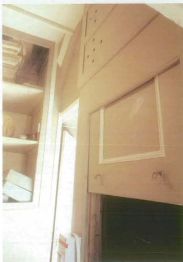
Fig 29 Isolated stair string [9] surviving above a door frame in G3, indicating the former existence of a staircase there between the ground and 1st floors; looking north-west. Hatch to later food hoist [17] in foreground
