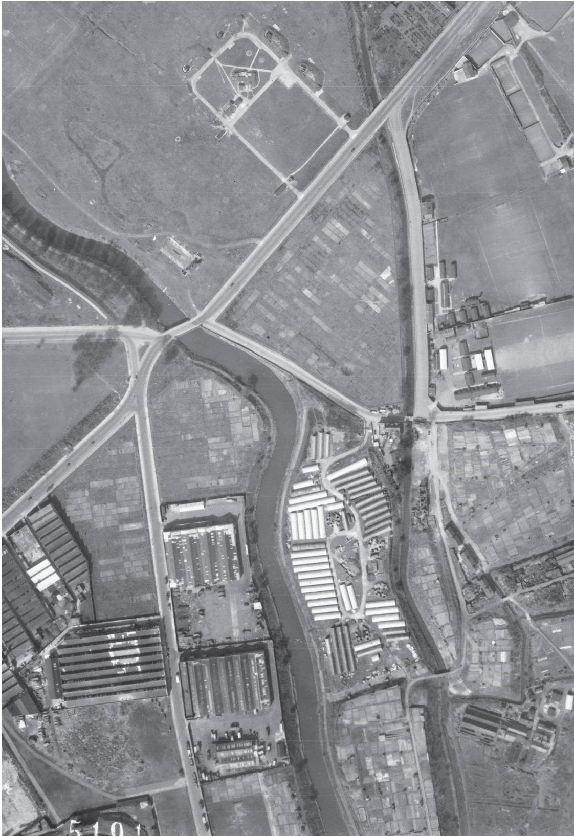
Fig 7 View of OL-01907: aerial photograph taken by the RAF, 2nd April 1946
