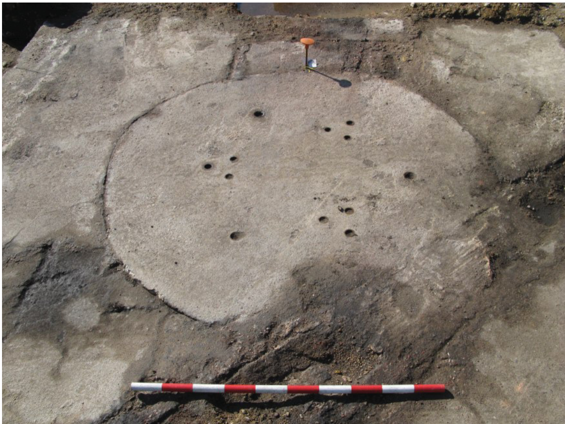
Fig 22 Detail of possible sockets for the mounting points of the rotating circular base of the predictor (mechanical computer) instrument
