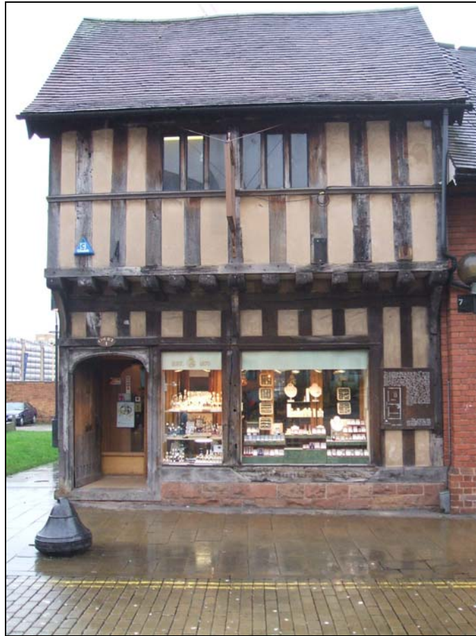
Plate 37: Court 6, Spon St (formerly 7 Much Park St)
