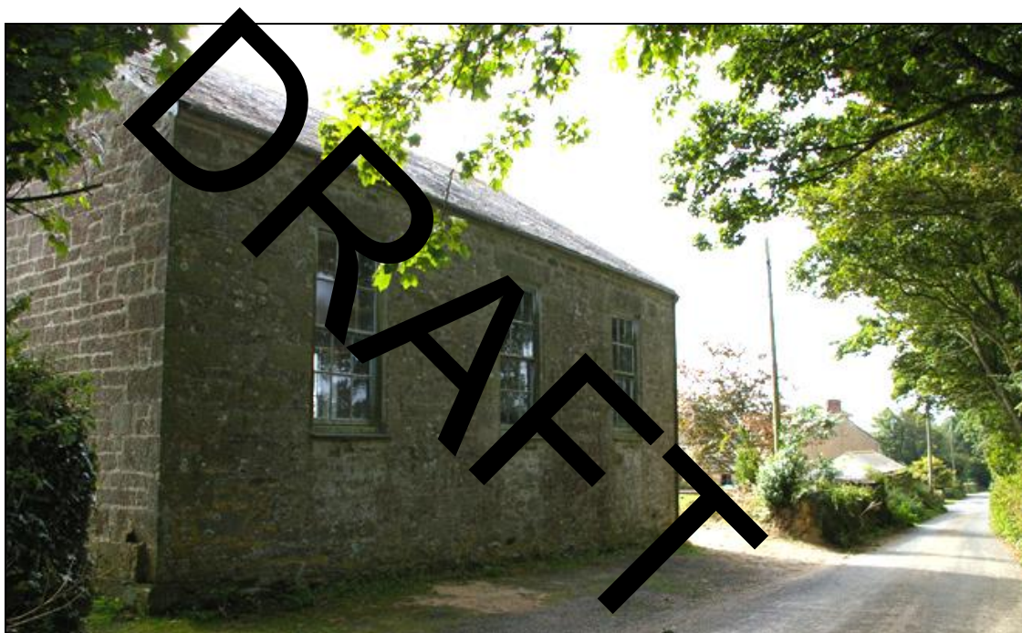
Figure 5: The exterior west elevation of the chapel; viewed from the north.
