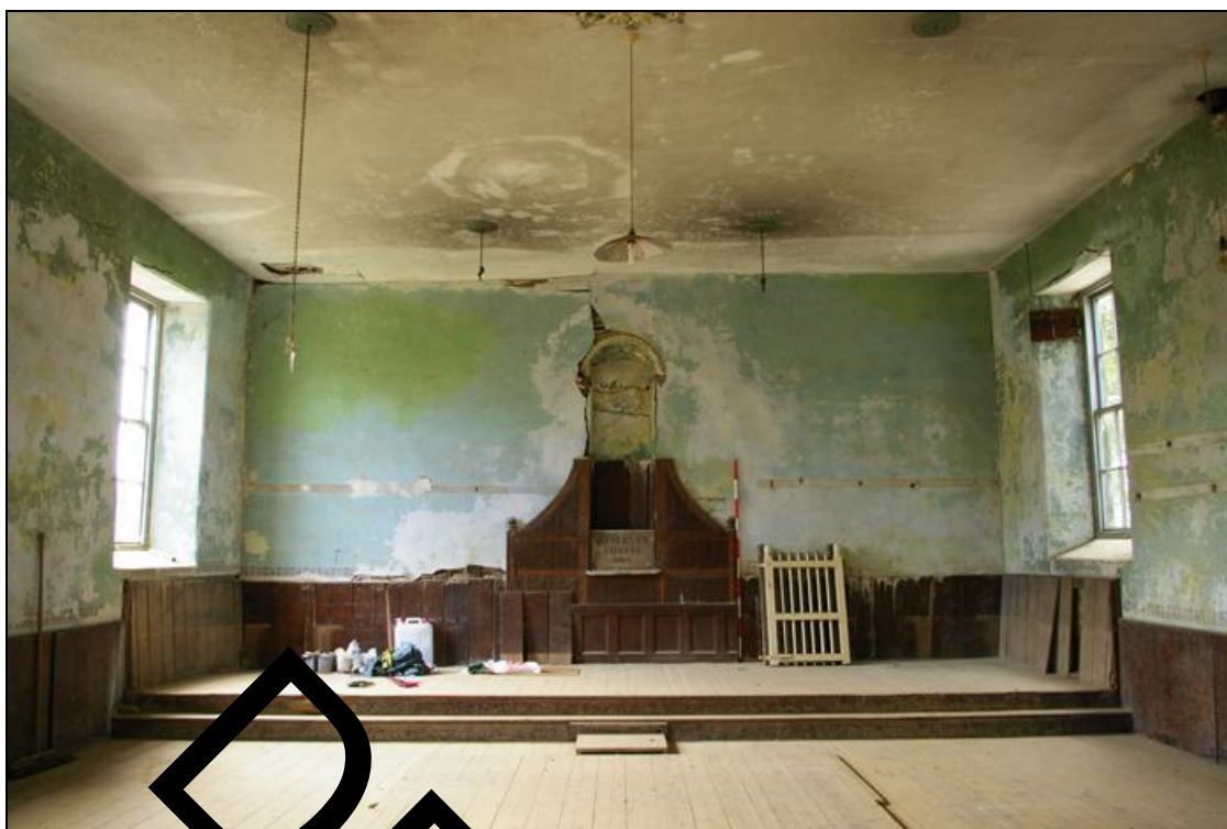
Figure 13: The interior south wall of the chapel; viewed from the north.
