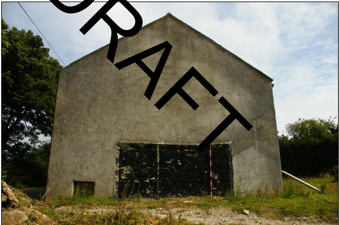
Figure 6: The exterior south elevation of the chapel; viewed from the south-west.
