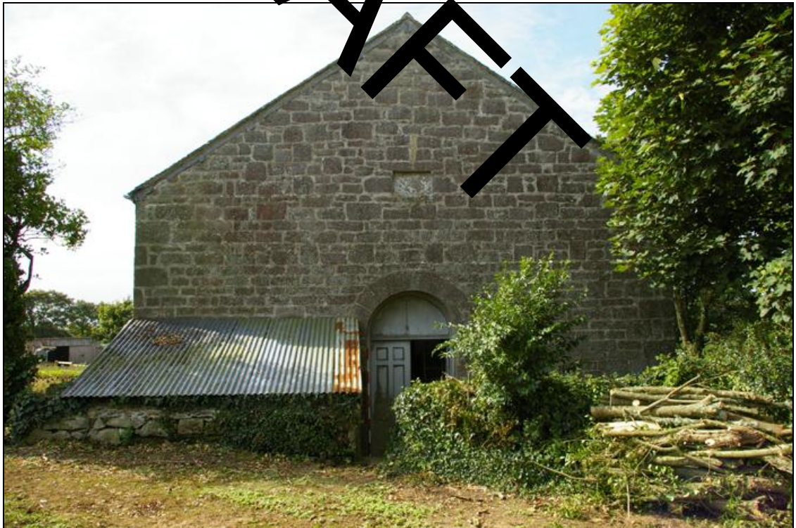
Figure 8: The exterior north elevation of the chapel; viewed from the north-east.
