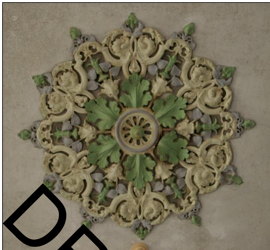
Figure 17: The central ceiling rose and vent.
