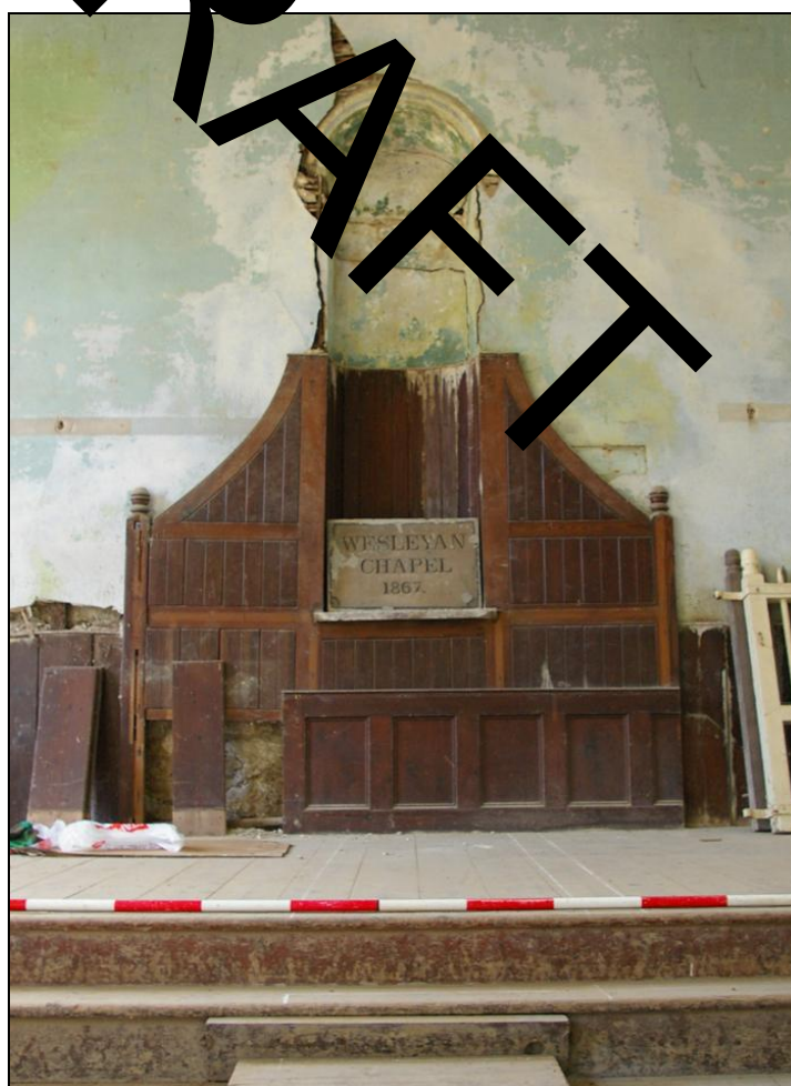
Figure 14: Detail of screen and alcove on the south wall.
