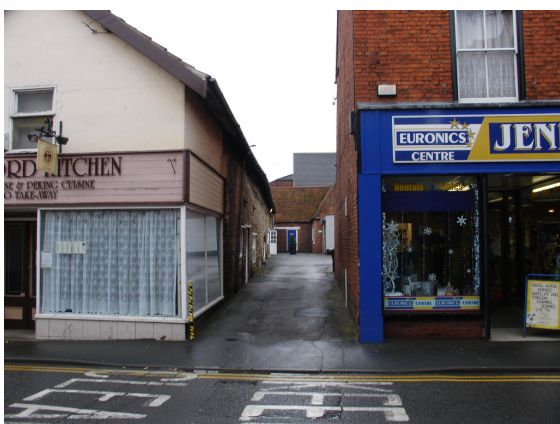
Plate 2 General view from Boston Road showing access to surveyed building
