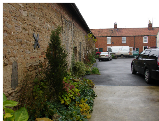
Plate 5 General view of surveyed building and funeral parlour yard, Boston Road at rear of photograph, looking north
