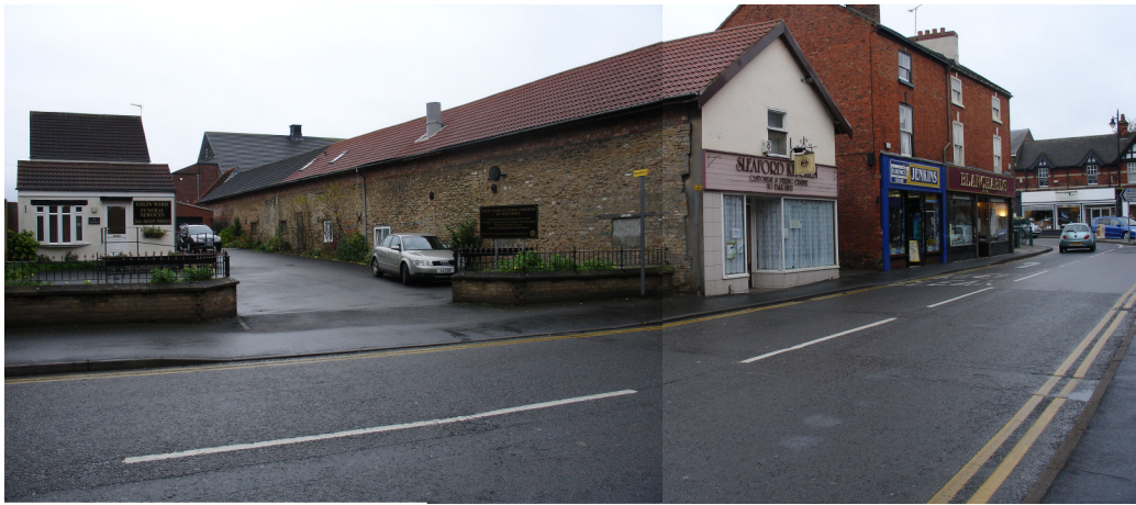
Plate 1 General view of the surveyed building and continuation as restaurant from Boston Road, looking southwest
