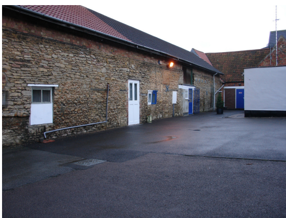
Plate 3 General view of surveyed building from yard, looking southeast
