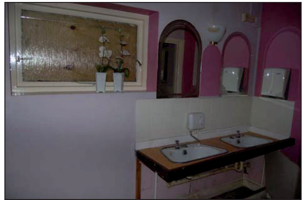
Plate 22: Room G8: north wall
