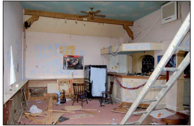
Plate 20: Room G3: north wall
