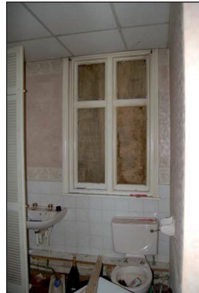
Plate 34: Room F4: north wall
