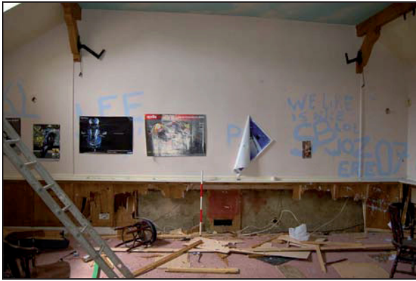
Plate 19: Room G3: west wall
