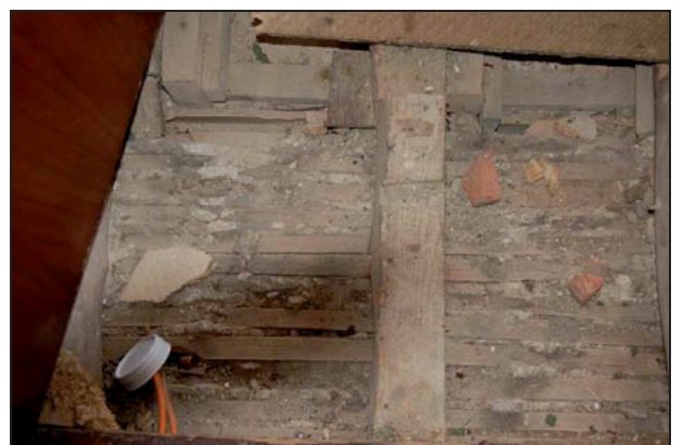
Plate 30: Room F1: lath & plaster ceiling below floor
