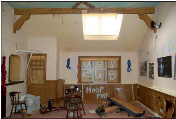
Plate 21: Room G3: south wall
