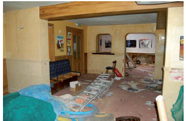
Plate 16: Room G2 looking west
