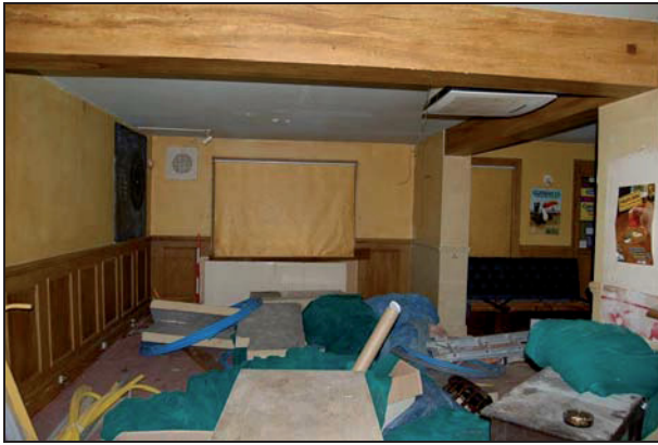
Plate 13: Room G2: south wall
