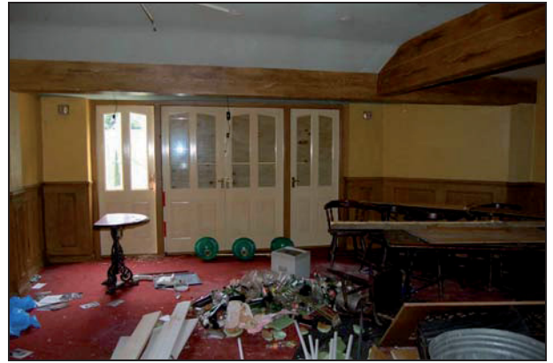
Plate 8: Room G1: north wall
