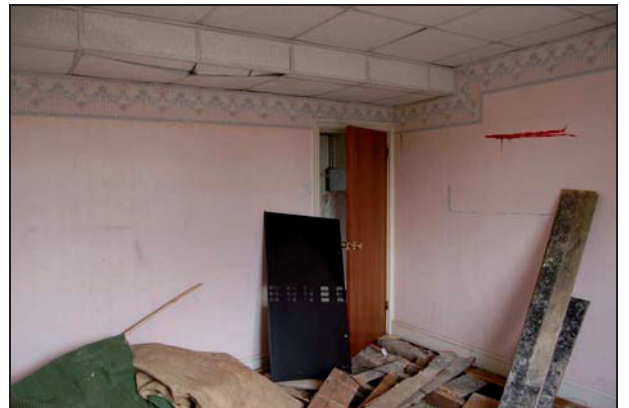
Plate 28: Room F1: northeast corner
