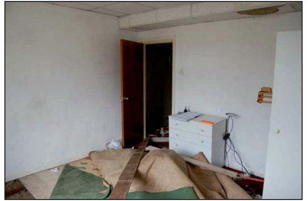
Plate 32: Room F2: northwest corner
