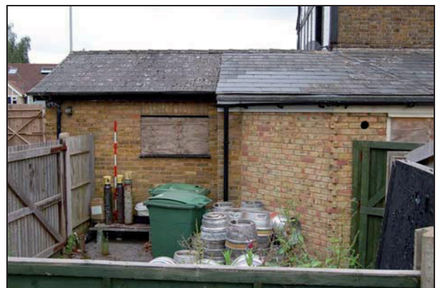
Plate 6: North elevation, east end
