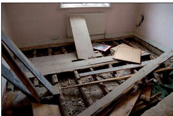
Plate 29: Room F1: floor
