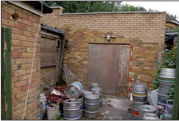
Plate 7: North elevation, west end
