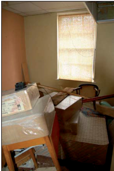
Plate 33: Room F3: east wall
