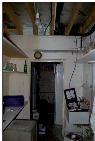
Plate 24: Room G10: looking north
