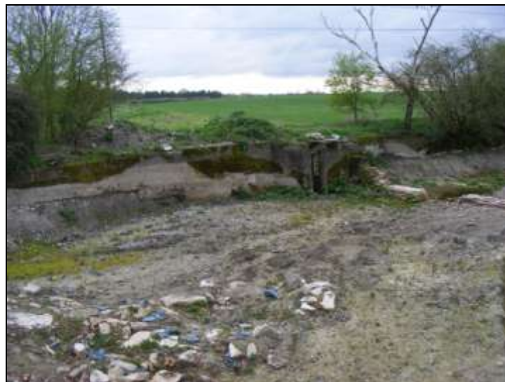
Plate 12: Concrete retaining wall, facing northwest
