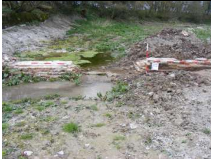
Plate 1: Footings of former dam, facing north
