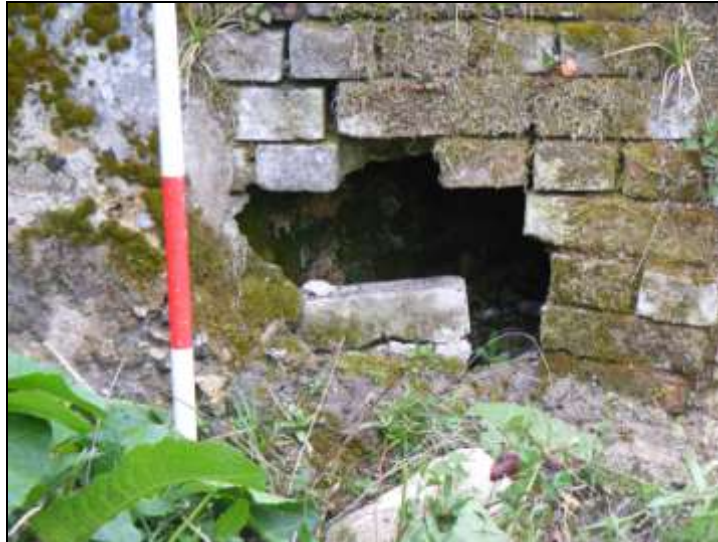
Plate 4: Culvert, facing north
