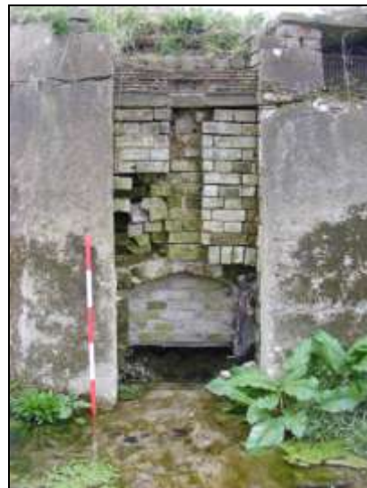
Plate 11: Outlet sluice, facing west
