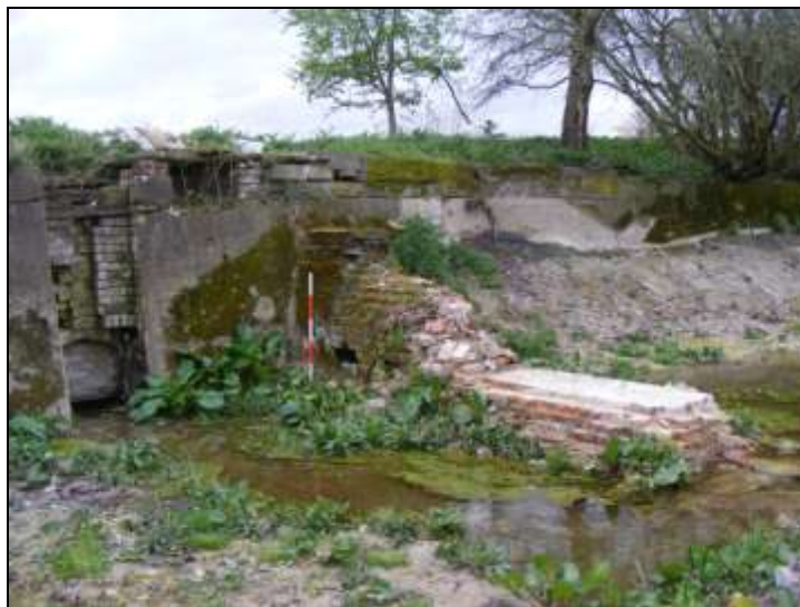
Plate 3: Western section of dam, facing northwest
