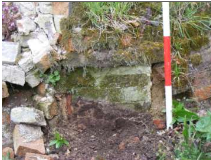
Plate 5: Culvert, facing south
