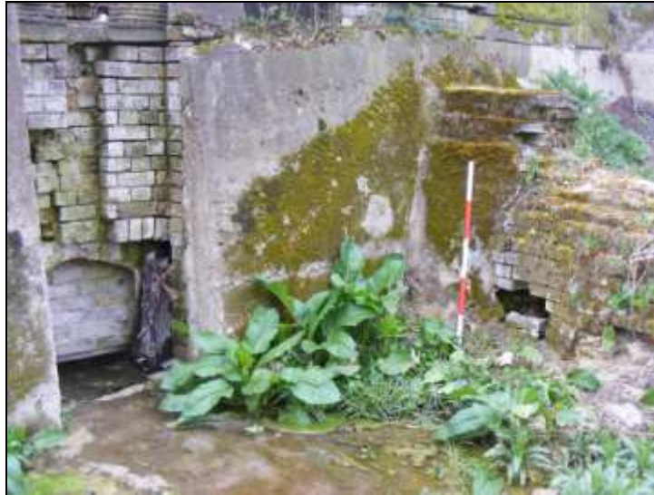
Plate 15: Rendered retaining wall, facing northwest
