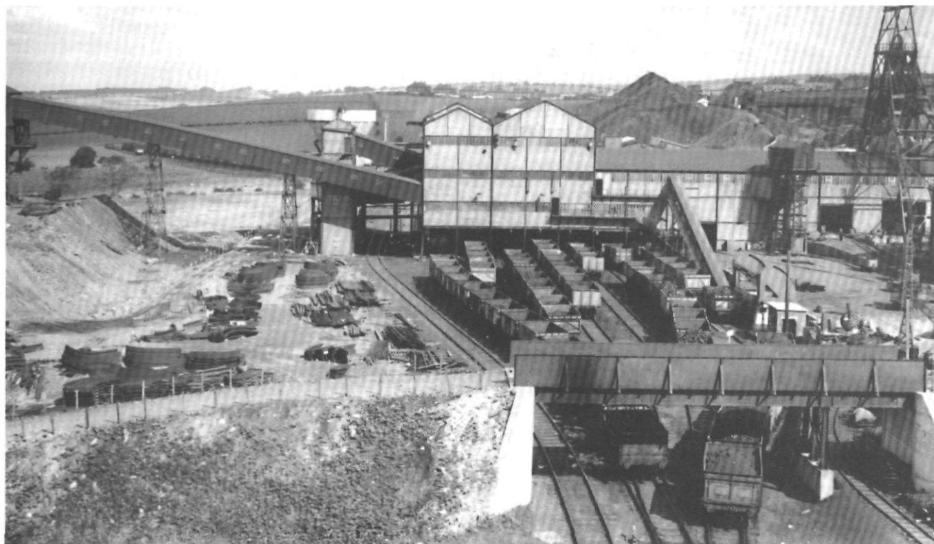
Fig 48 National Monuments Record of Scotland: a view of Littlemill Colliery, East Ayrshire, in 1958, showing dirt disposal, Preparation Plant and Car Circulation Hall, from the Harrison Collection. (RCAHMS: B 78904)
