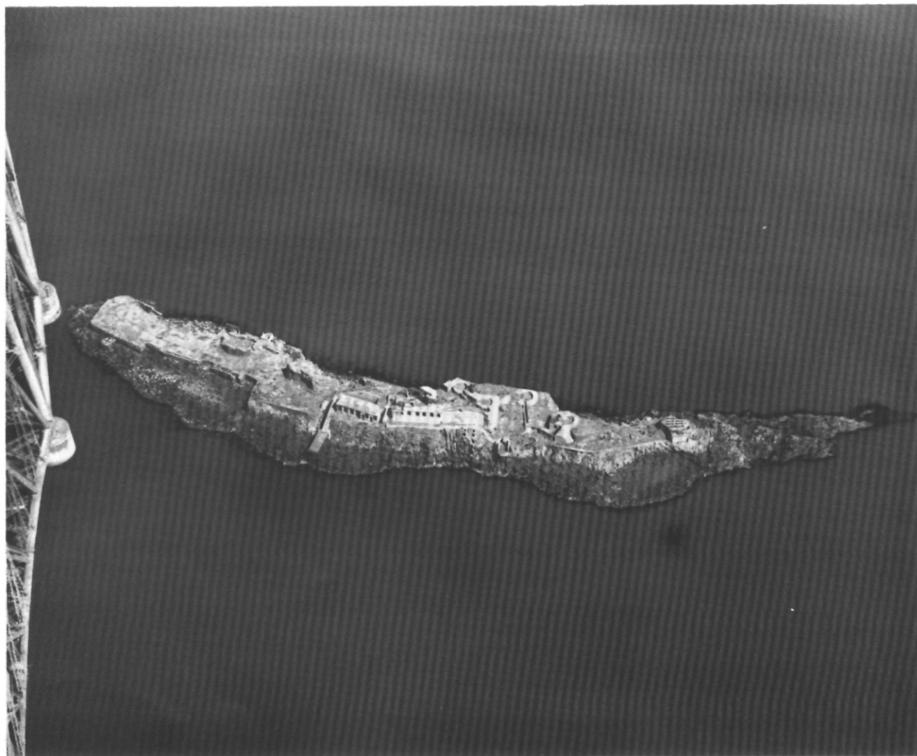
Fig 38. Aerial view of the fort and coastal batteries on Inchgarvie Island at the foot of the Forth Bridge in the Firth of Forth. (© RCAHMS, D32226)
