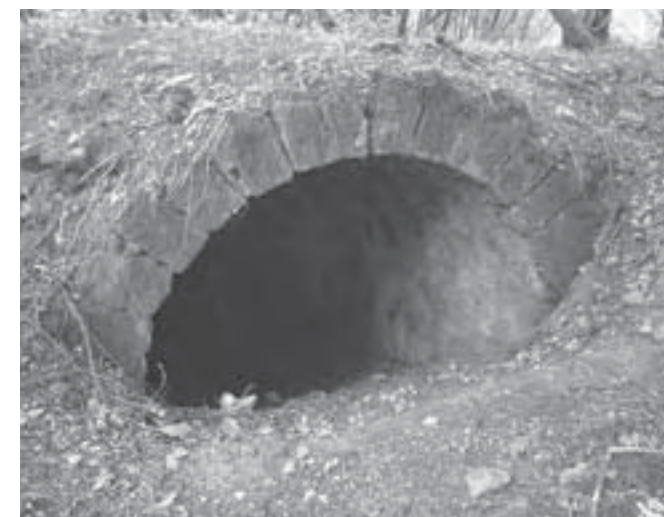
Fig 31. Blinkbonny waggonyway tunnel.
