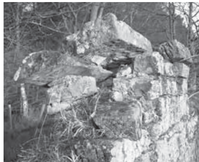
Fig. 52 Photo of wall cope.
