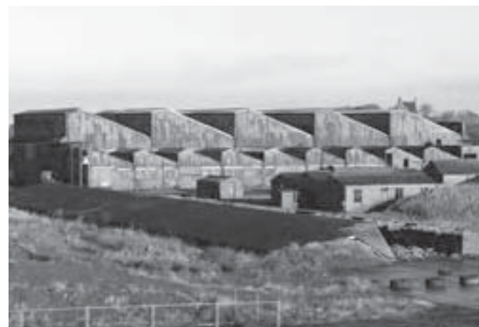
Fig 25. Crail Airfield, hangars.
