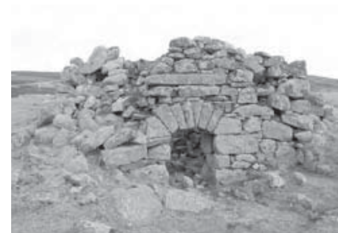
Fig. 63 View of a late-19th century limekiln at Fae, Braes of Abernethy (NJ01NE 27). The arched draw-hole is characteristic of both limekilns and kilnbarns on the former Seafield Estate. (© Crown copyright: RCAHMS DP02948).
