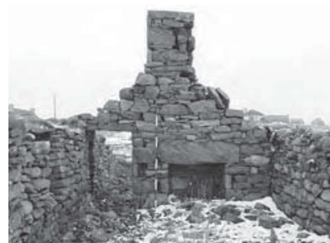
Fig. 54 Gable end of blackhouse with intact chimney, Knockaird, Ness, Isle of Lewis.
