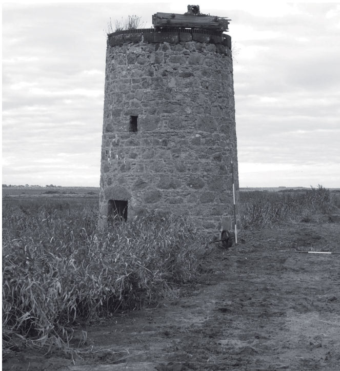
Tower of Strathbeg Pumping Mill from SE.
