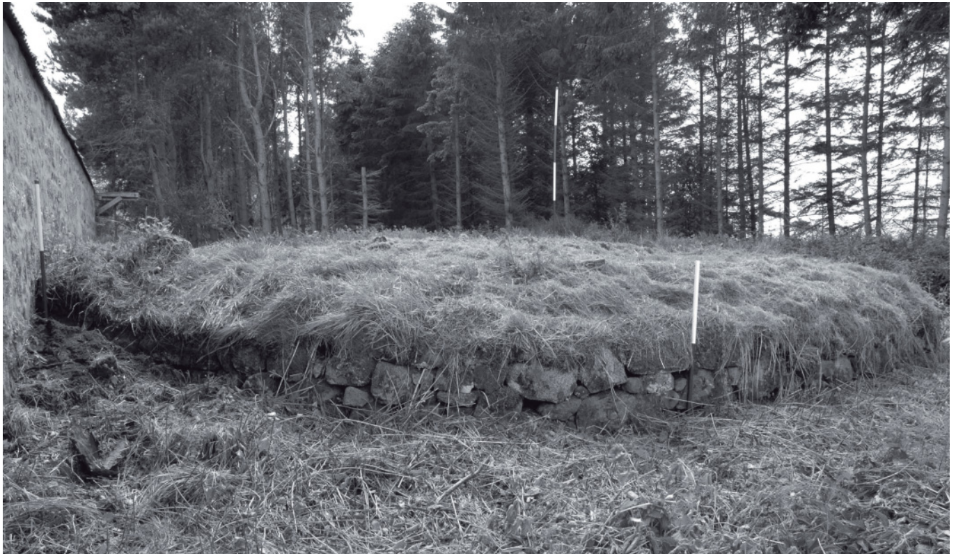
Tillychardoch horse mill showing the stone revetted horse engine platform.
