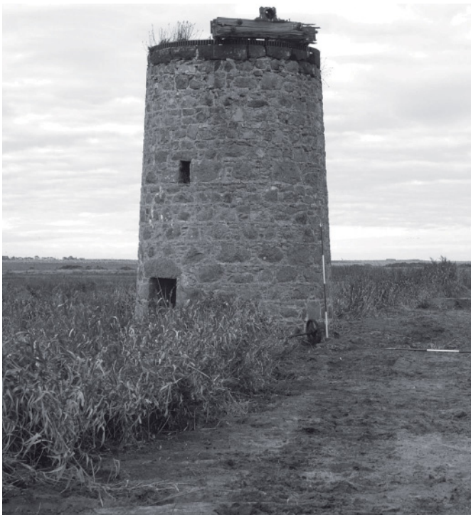
Tower of Strathbeg Pumping Mill from SE.
