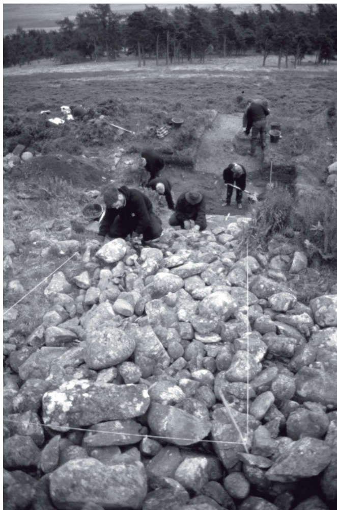
View of the rampart, ditch and counterscarp bank of the White Caterthun multivallate fort, taken during excavations by CFA Archaeology Ltd, 1995–6. Accession Number 2007/154 (Copyright: Historic Scotland SC 1097417).
