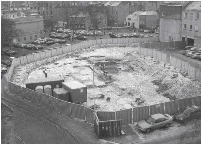
Excavations at Horse Cross, Perth, by SUAT Ltd, 2003. (Copyright SUAT Ltd: RCAHMS DP073192)
