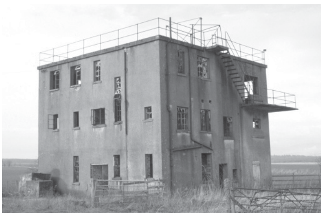
Photographs from a survey of the Second World War airfield at Clathymore, Findo Gask, Perth and Kinross, by SUAT Ltd, 2004. (Copyright SUAT Ltd: RCAHMS SC1138269 (control tower), RCAHMS SC1138271 (Nissen hut) and RCAHMS SC1138272 (detail of Nissen hut))
