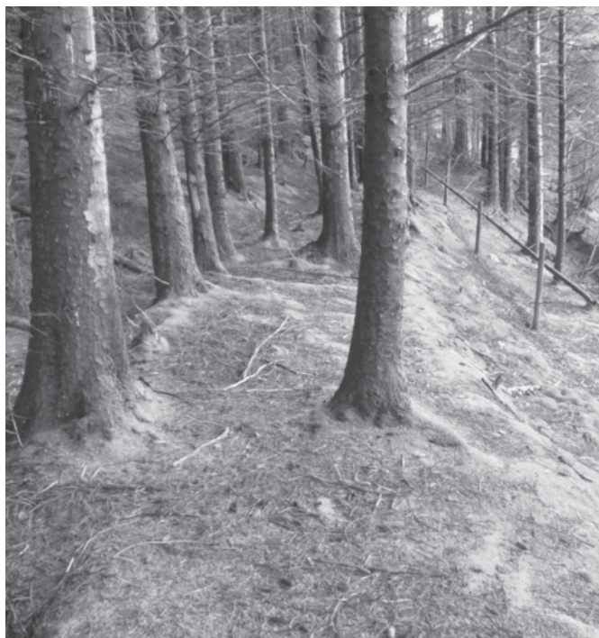
Exceptionally well preserved section of military road leading to the ferry at Callert
