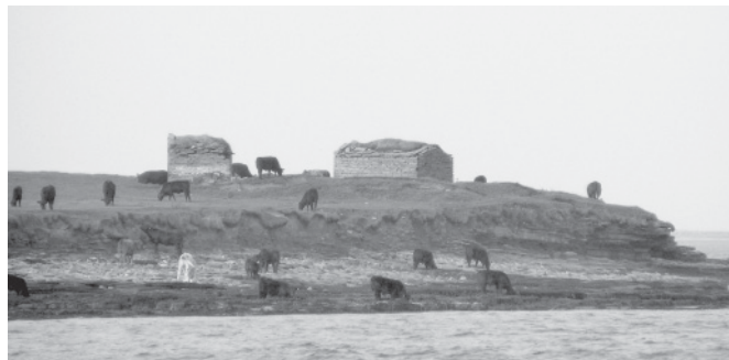
General view of emplacement from Egilsay ferry, with Hut A on left. From S, September 2009 © David Lynn
