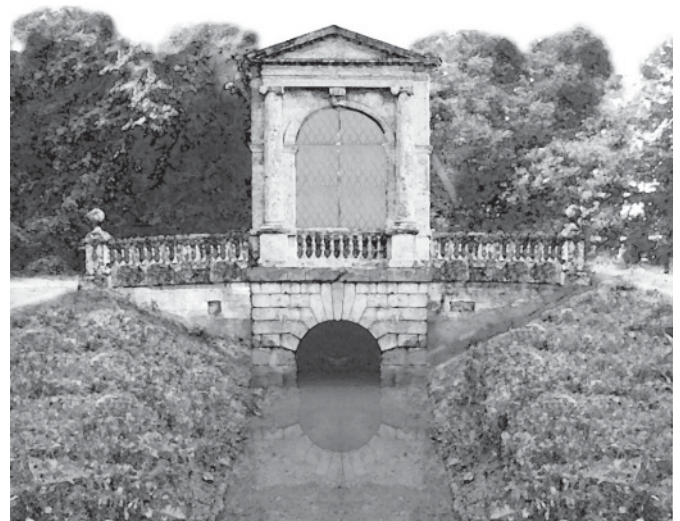
Reconstruction of the Newhailes Tea House
