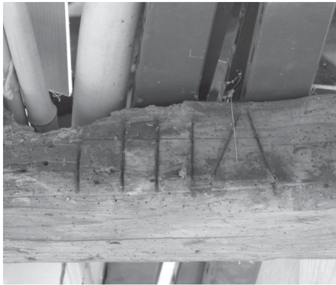
Cross Keys Close, Brechin. Carpenter's mark on roof timber
