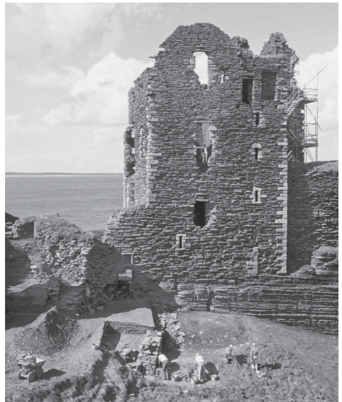
Excavation in progress at Castle Sinclair Girnigoe
