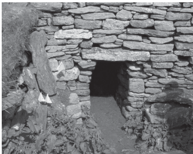
North Rona. View from WSW of the 'Oratory' adjoining the ENE end of the chapel. Although much of this end of the oratory has been rebuilt, the rest of the structure, including the corbelled walls which rise to a slab-capped ridge some 3.1m in internal height, is original, probably dating to the latter part of the 1st millennium AD. (Crown Copyright RCAHMS DP072352).
