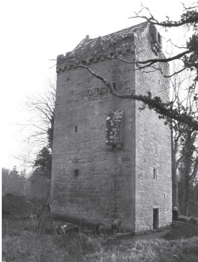
Excavations at Tower of Hallbar, South Lanarkshire, by GUARD, 1999. (Copyright GUARD: SC1136095)
