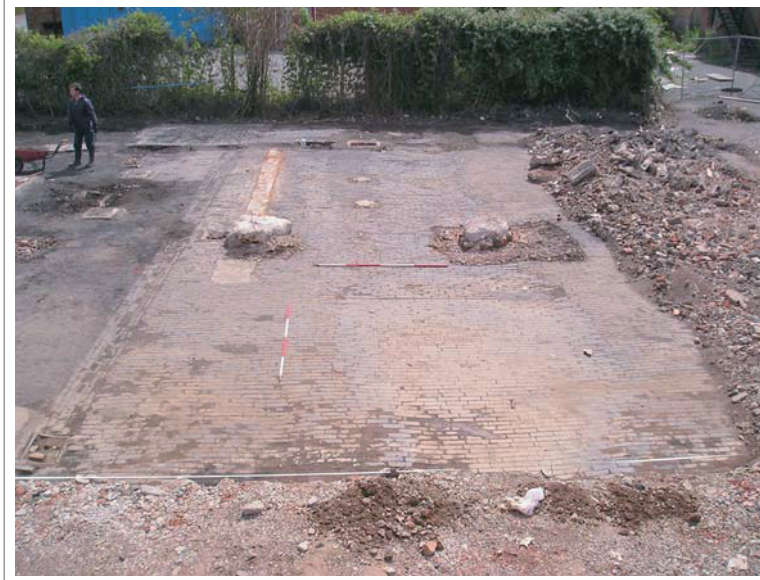
Plate 04: 1962 building supports in relation to 1887 floor, scale 2m x 2m
