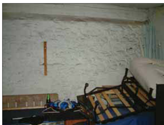
Plate 6: L-shaped building currently used for storage adjoining the northeast end of the Attic Bar and Nightclub, internal view showing modern brickwork over earlier stonework (whitewashed) in the northeast elevation, looking northeast
