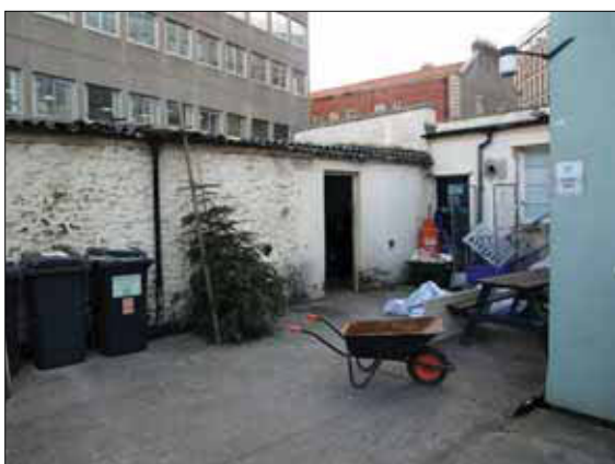
Plate 5: L-shaped building currently used for storage adjoining the northeast end of the Attic Bar and Nightclub showing earlier (whitewashed) stonework incorporated in the southwest elevation, looking southeast
