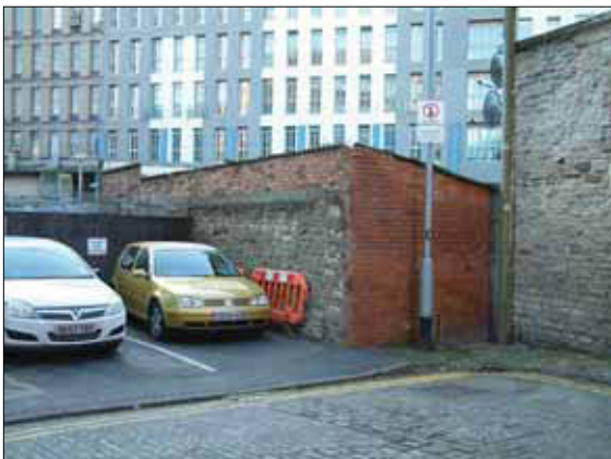
Plate 9: L-shaped building adjoining northeastern end of the Attic Bar and Nightclub showing modern brickwork constructed over earlier masonry in the unrendered rear (northeast) elevation, looking south from Wilder Street
