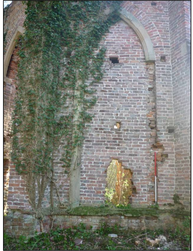
Plate 6: Exterior of Side A, looking S (photo 1/634).
