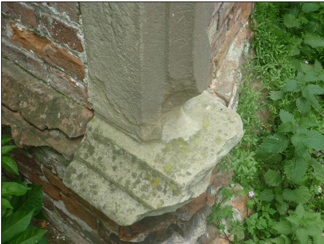
Plate 4: Typical brick and limestone moulding to plinth, base of Side C (photo 3/377).
