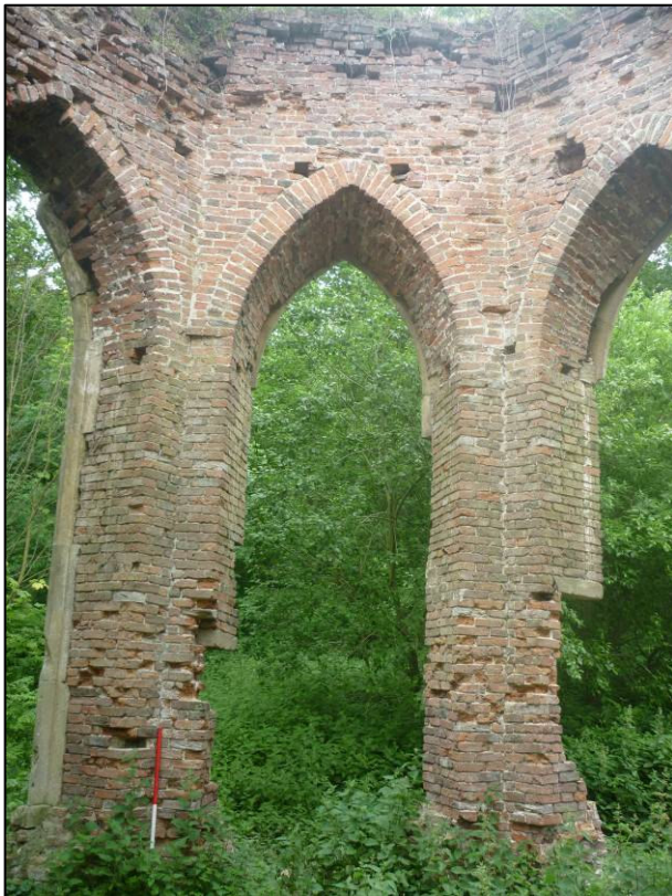
Plate 10: Interior of Side D, looking SE (photo 3/363).
