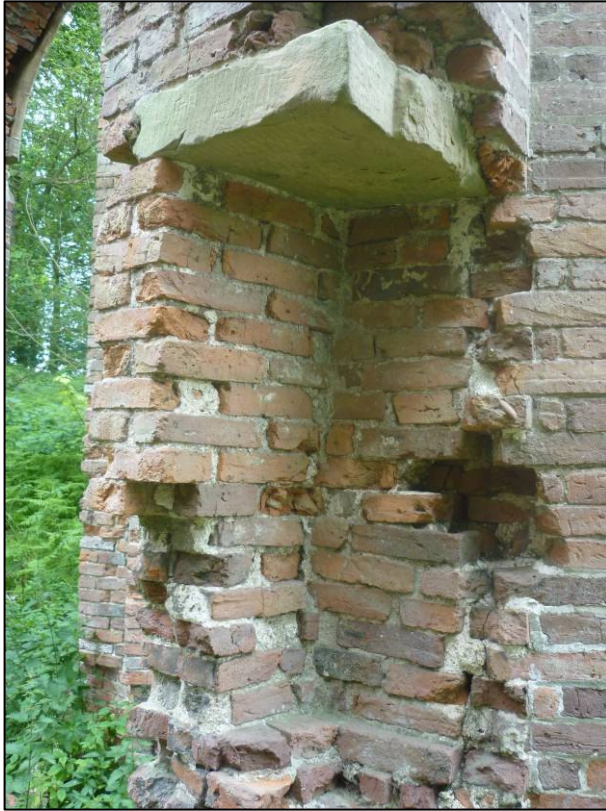
Plate 5: Recess to north side of Side D, looking NE (photo 3/378).
