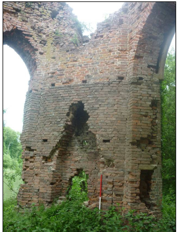
Plate 11: Interior of Side A with fireplace, looking N (photo 3/360).
