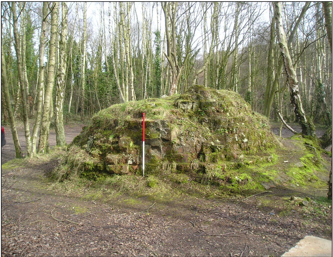
Plate 6: Furnace base (Site 8), looking NE.
