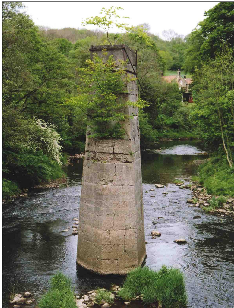
Plate 8: Bridge pier (part of Site 19), looking N.
