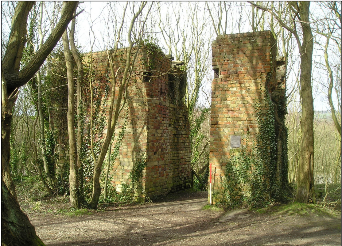
Plate 7: Remains of hoist / lift (Site 2), looking NW.
