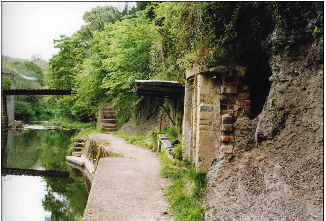
Plate 10: Wharf and related structures (Site 22), looking NE.
