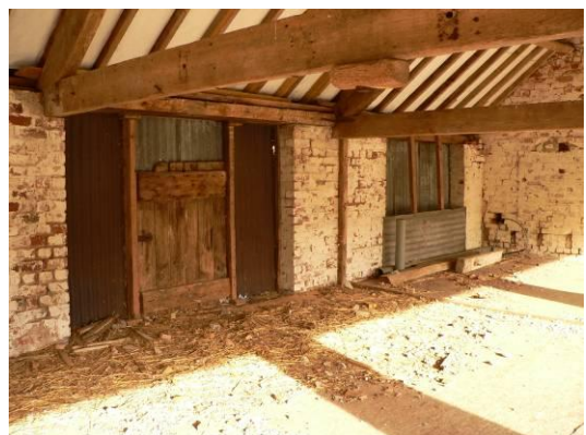
Closed openings in north wall, bays 6 and 7
