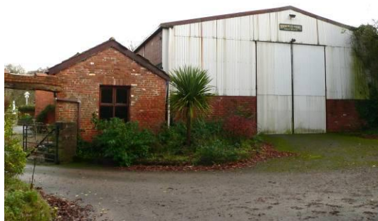
Modern shed and west gable of outbuilding, with farmyard entrance to left
