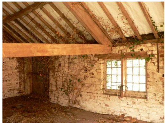
Linhay, first floor, bays 1 and 2, north wall
