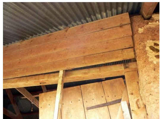
Timber cladding over west central doorway
