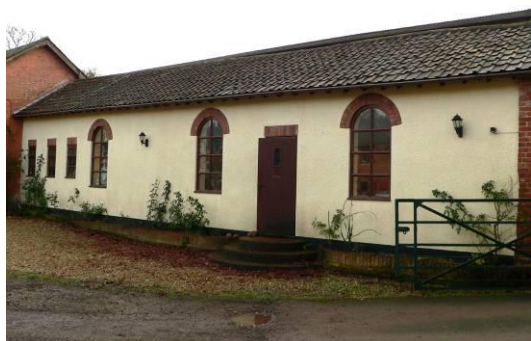
Converted outbuilding on south side of yard, west end
