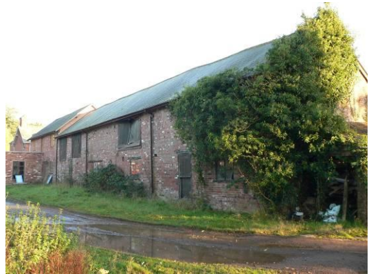
North side of linhay from north-west
