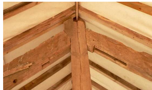
Roof truss apex, showing re-used timbers
