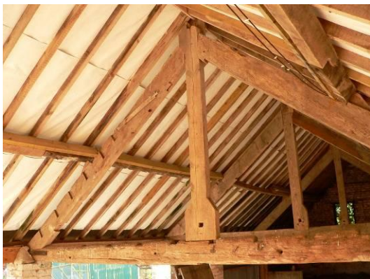
Roof truss, showing re-used timbers
