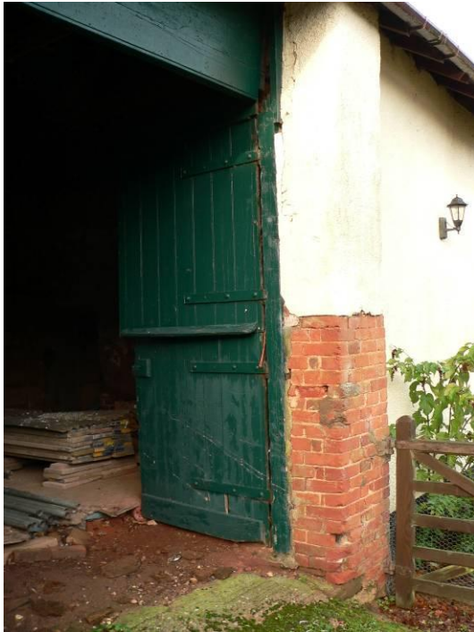
Brickwork repair to pier, east doorway
