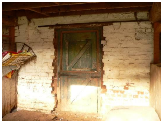
Inserted door in north wall of loose box, ground floor, bay 2
