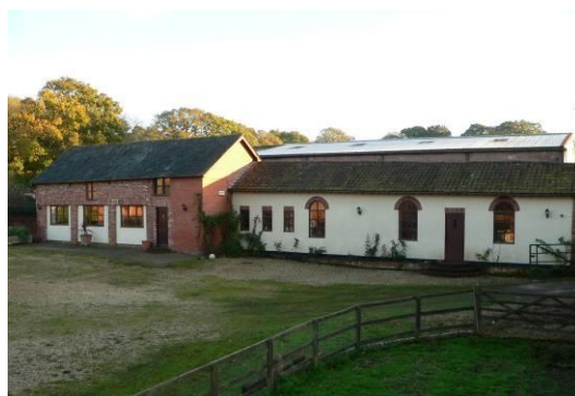
Converted buildings on south side of farmyard, from linhay
