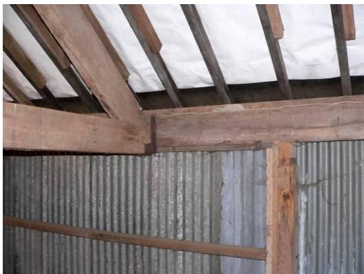
Tie beam support, south side, bays 1-2
