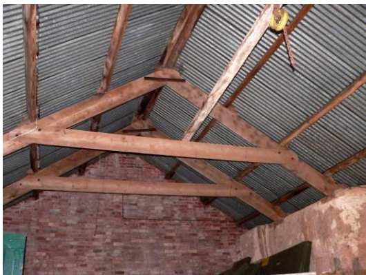
Barn roof, looking south
