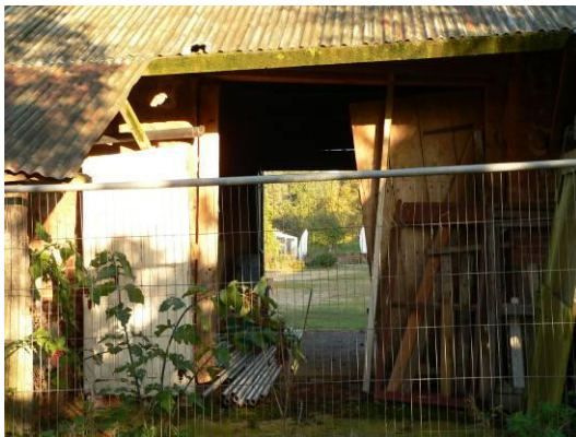
Barn, west elevation, lean-to
