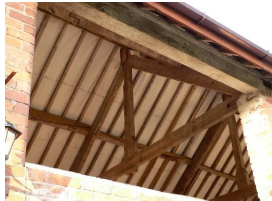
Looking up into roof of bay 5 from west
