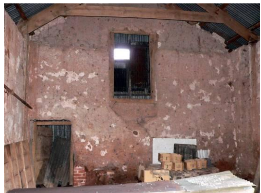
Cob north gable wall of barn
