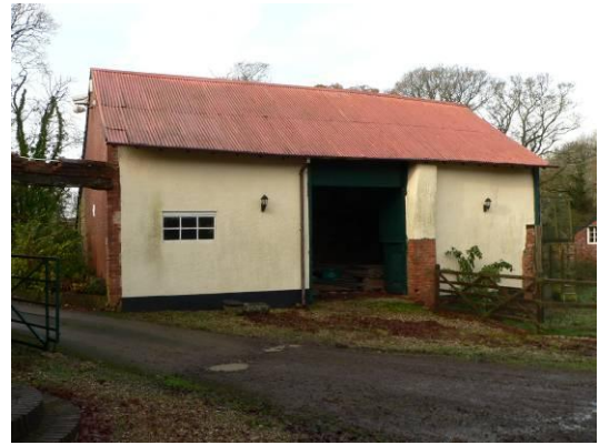
Barn, east elevation to farmyard
