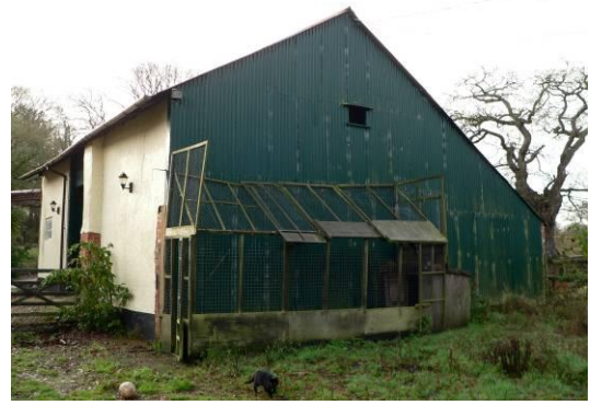
Barn, north gable
