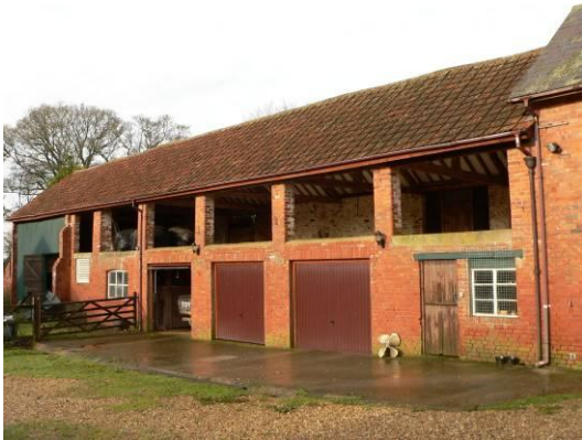
Linhay, south elevation from south-east
