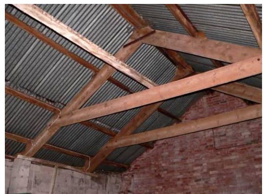
Roof structure, looking to south-east
