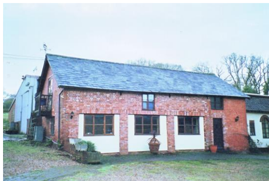
Converted outbuilding at east end, south side of farmyard
