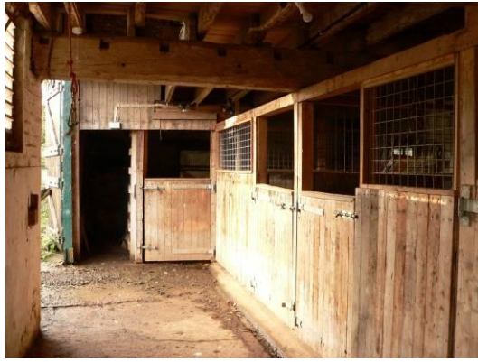
Loose boxes at west end of linhay
