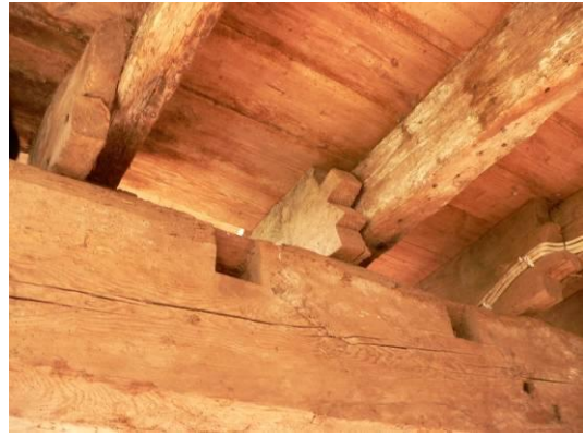
Re-used timbers supporting tallet floor
