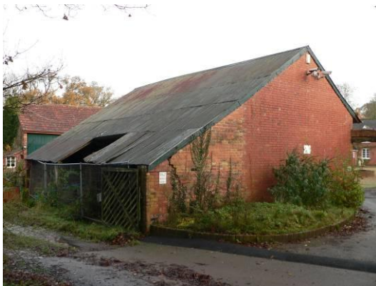
Barn from south-west
