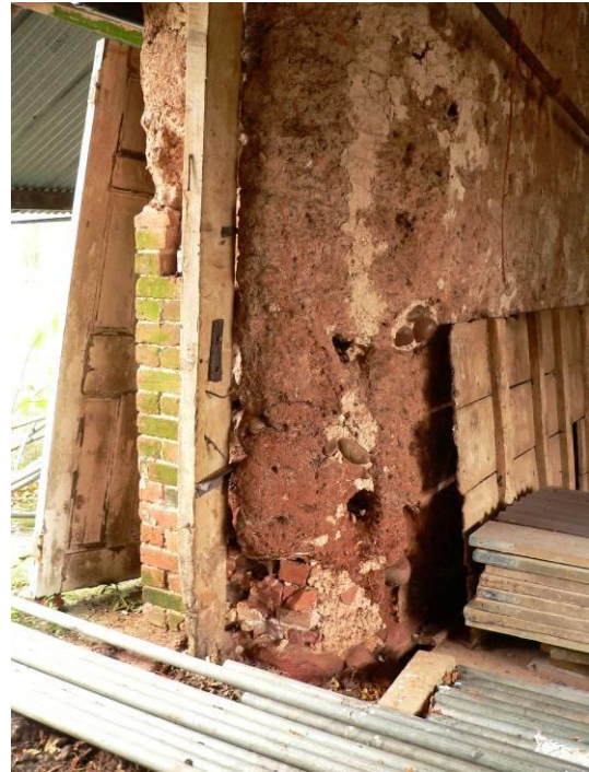
Cob repair and north side of central doorway on west side
