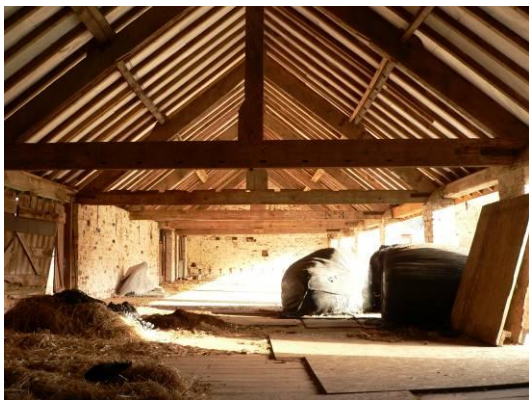
Tallet floor, looking from west end
