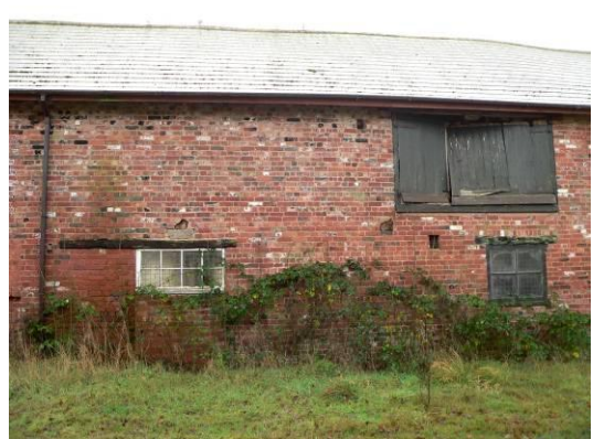
Former openings in north elevation of linhay
