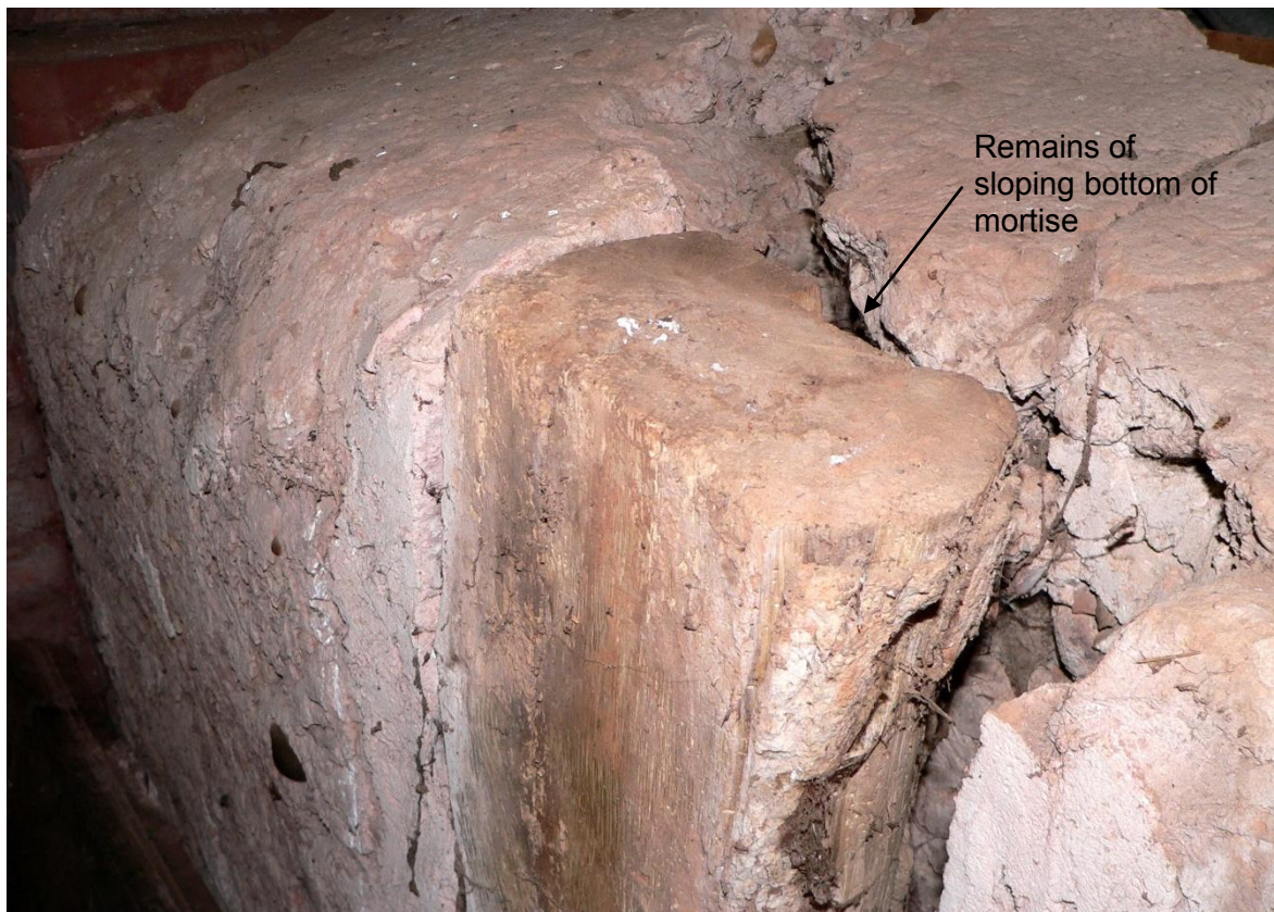
Sawn off head of south post
