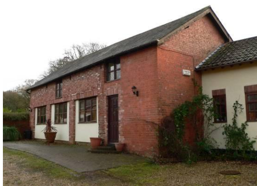
Converted outbuilding on south side of yard, east end
