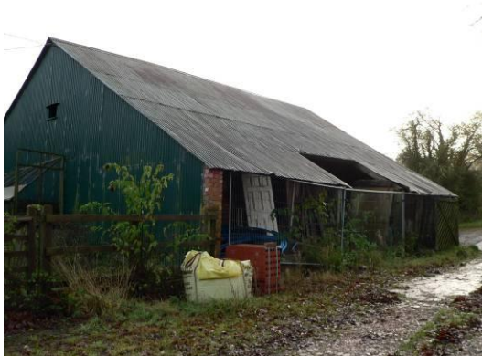
Barn from north-west
