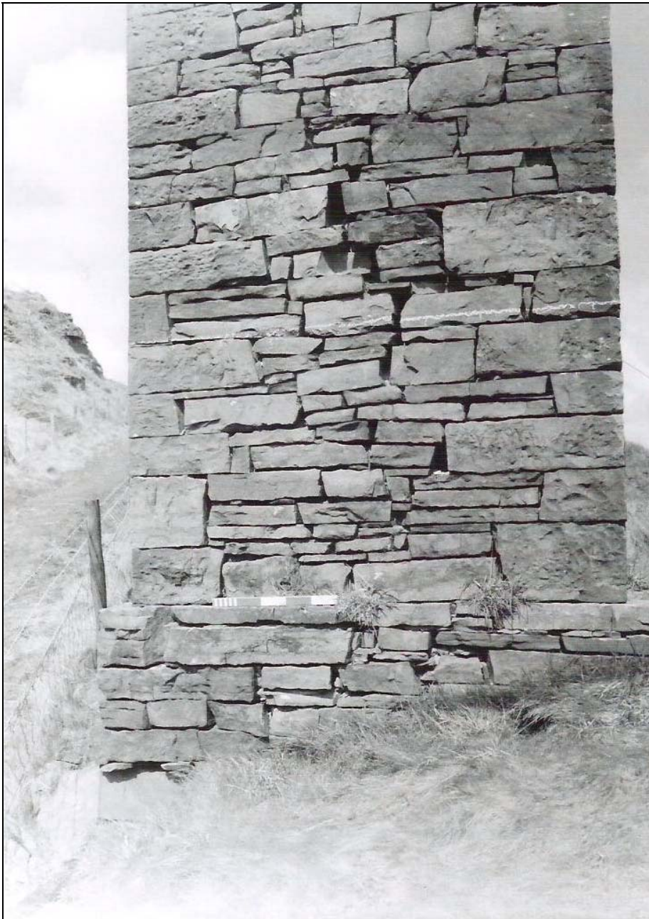
Plate 2: Plinth at Base of South Elevation
