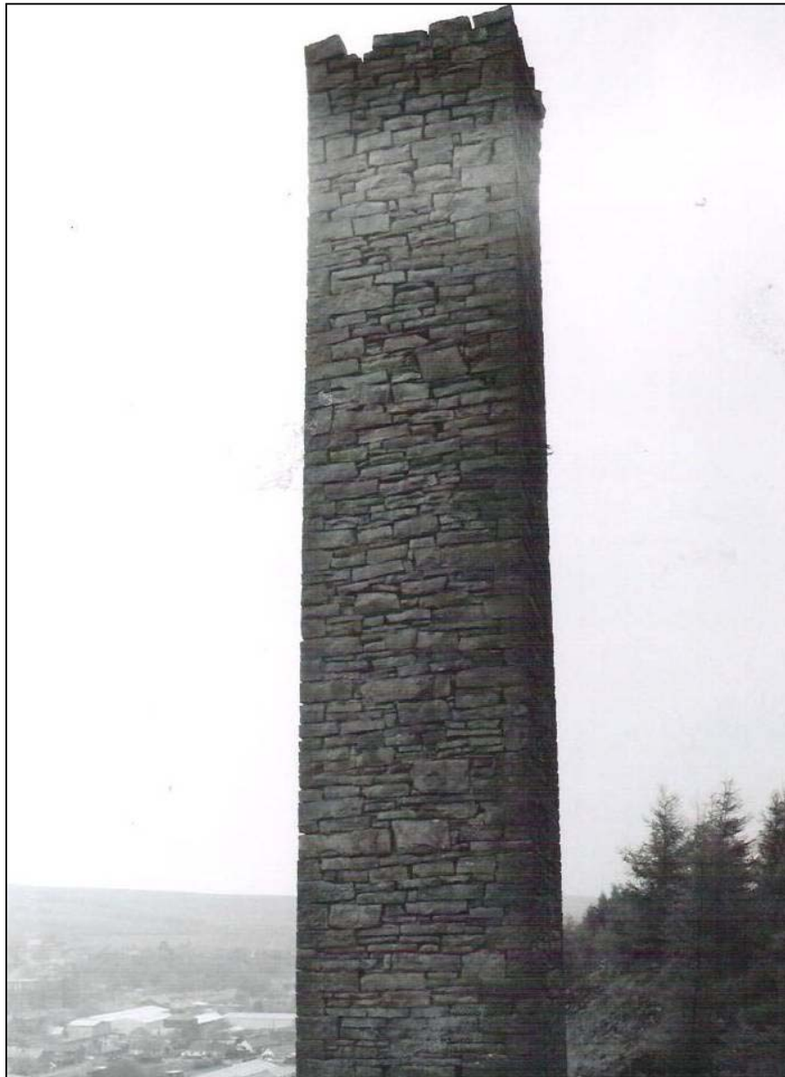
Plate 10: Top of North Elevation
