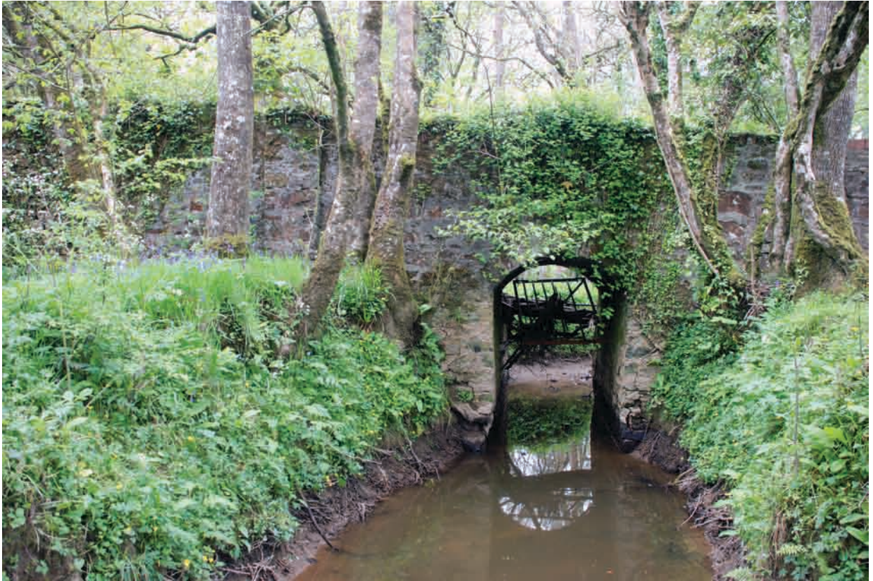
Plate 5 The downstream side of the open flood arch.
