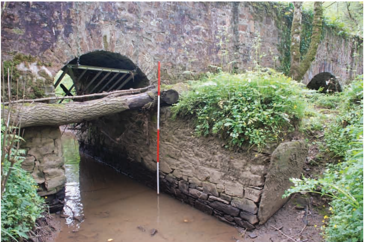
Plate 6 The upstream side of the open flood arch.
