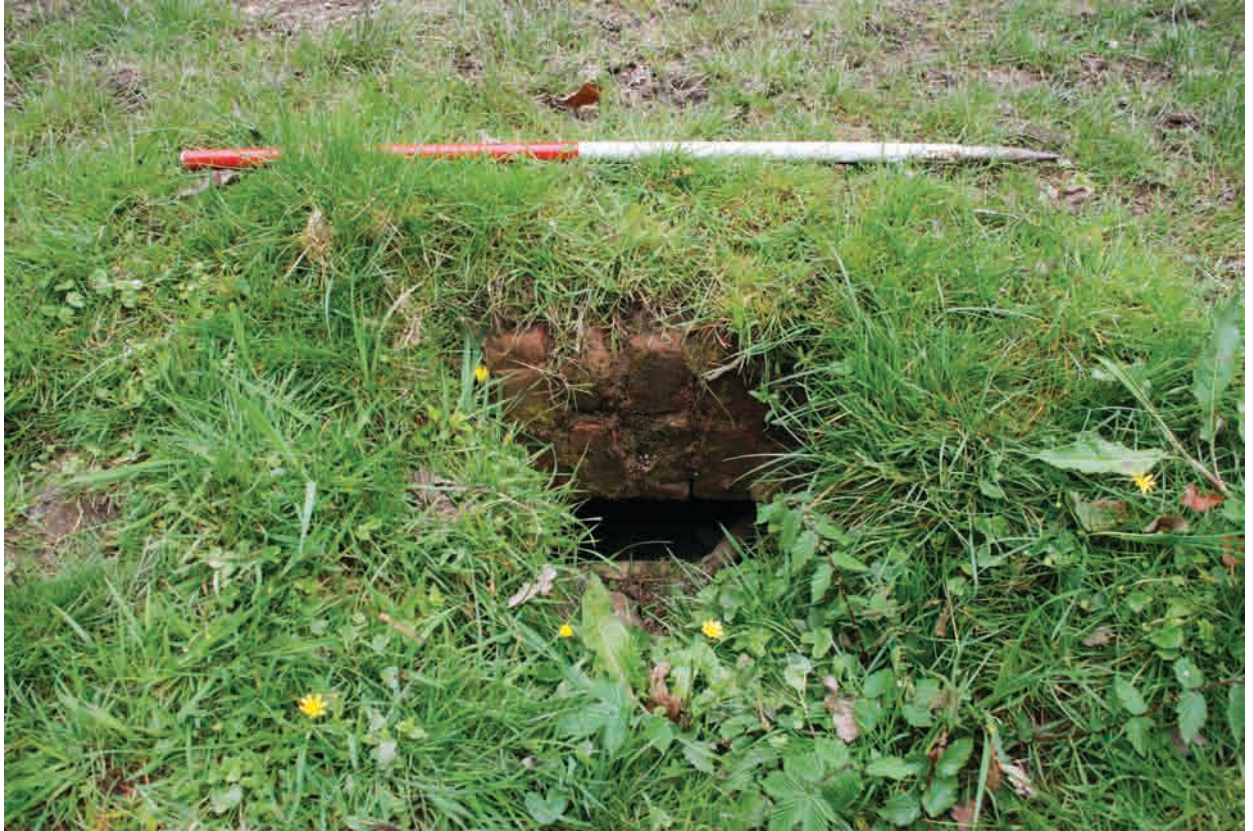
Plate 9 The hand-made brick vault of the disused flood arch, looking northwest.
