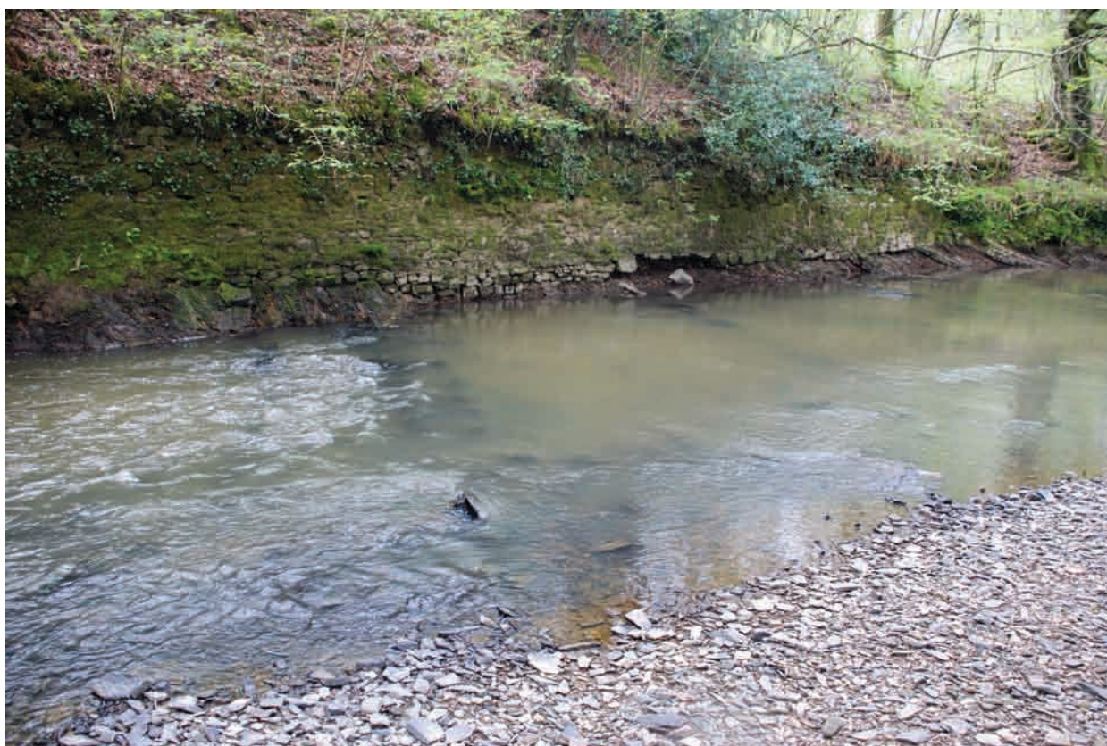
Plate 14 The stone wall revetting of the riverbank upstream from the bridge, looking west.
