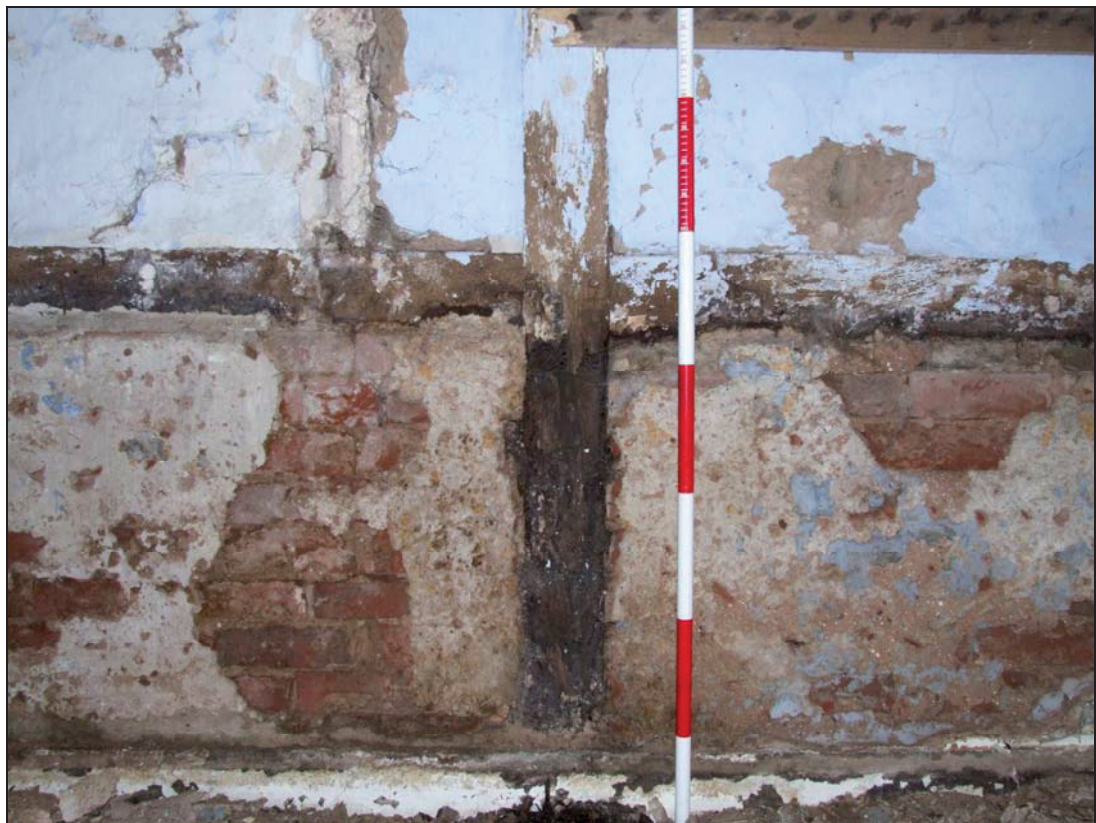
Plate 20. Detail of the timber framed partition – Room 3
