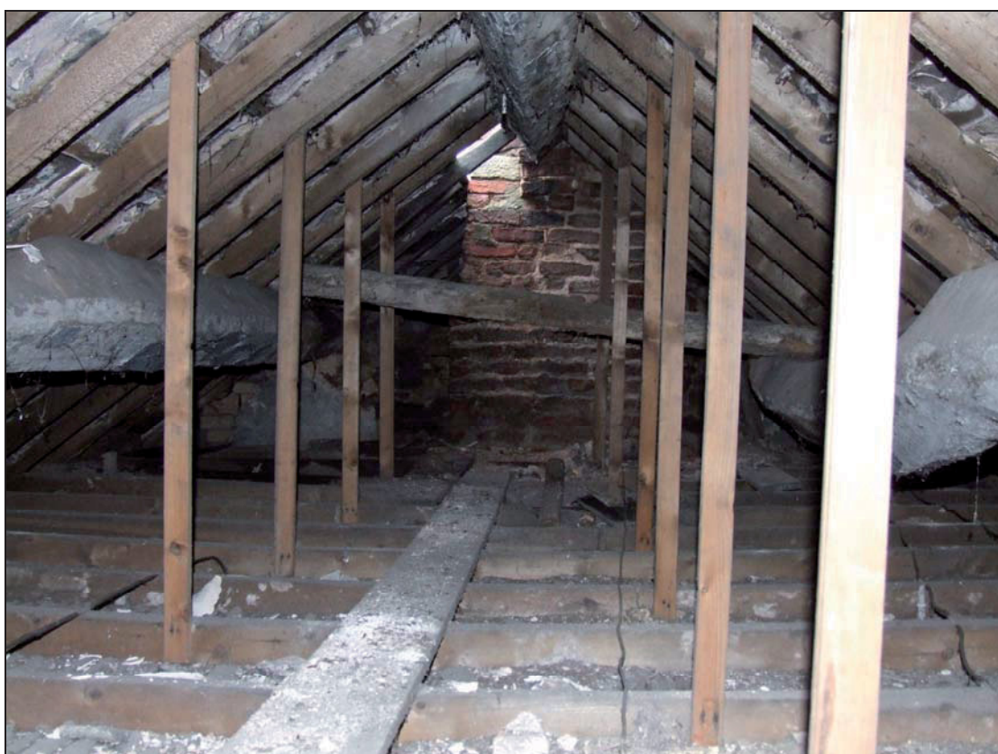
Plate 32. The handmade brick chimney and vertical timber supports from the west
