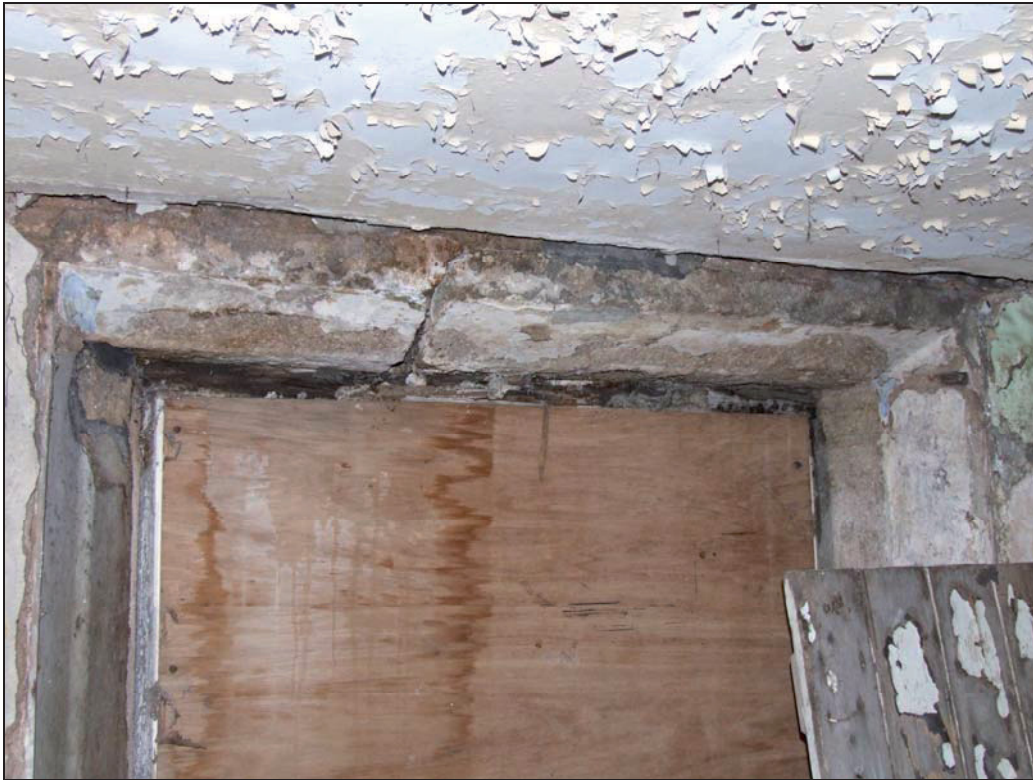
Plate 21. Detail of chamfered window lintel and jambs – Room 3
