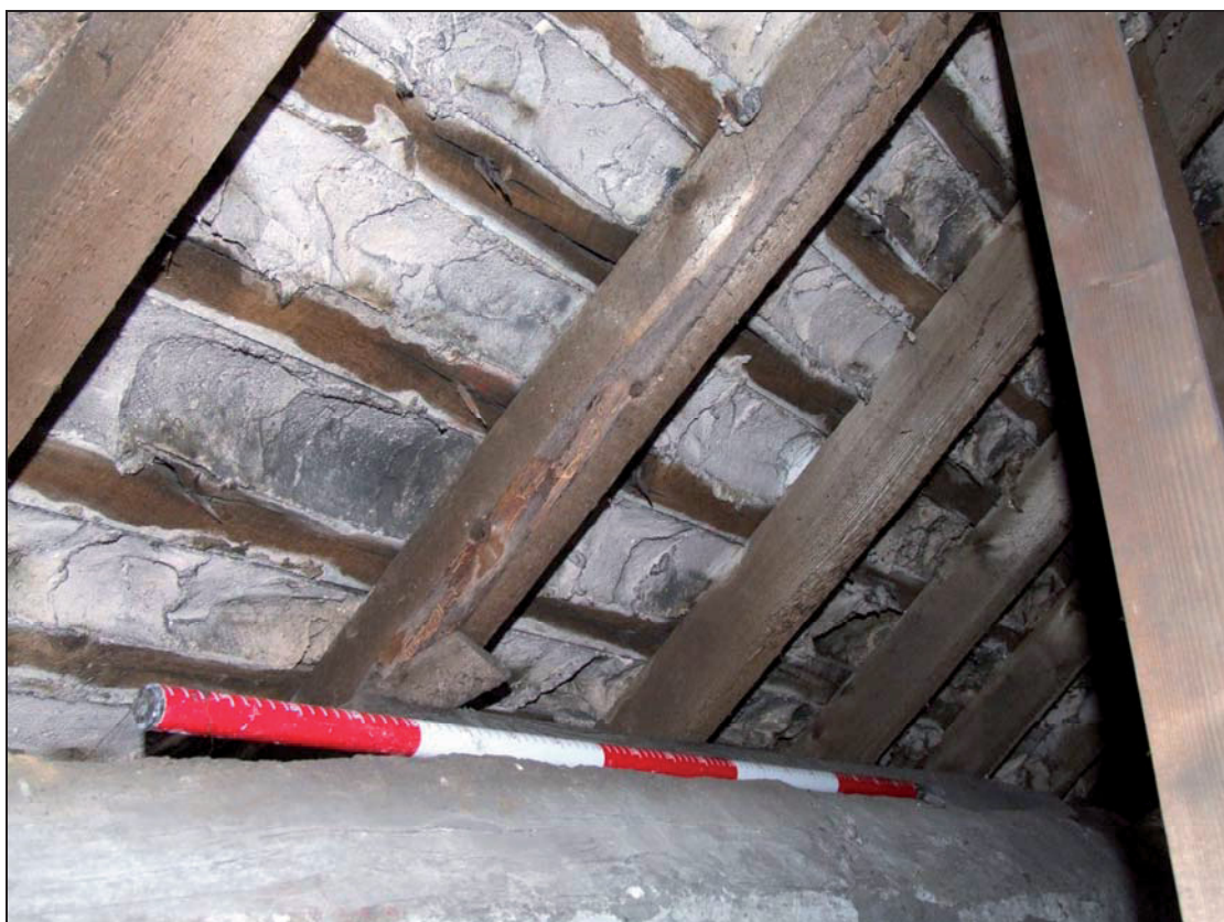
Plate 33. Machine cut timber rafters
