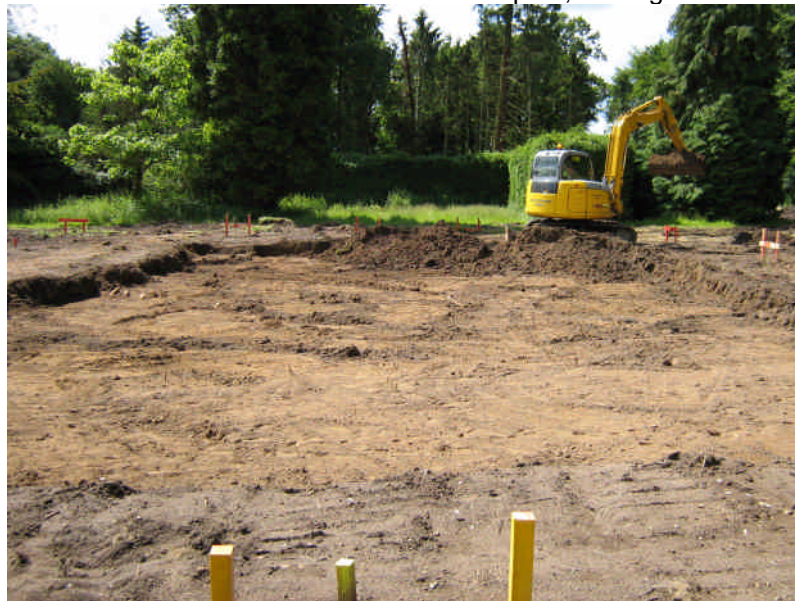
Plate 1 Excavation of the house footprint, looking west
