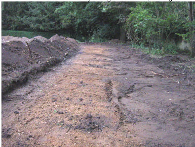
Plate 4 Driveway during excavations, looking east
