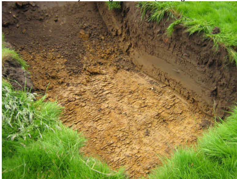
Plate 3 Soakaway 2 during excavation, looking southwest
