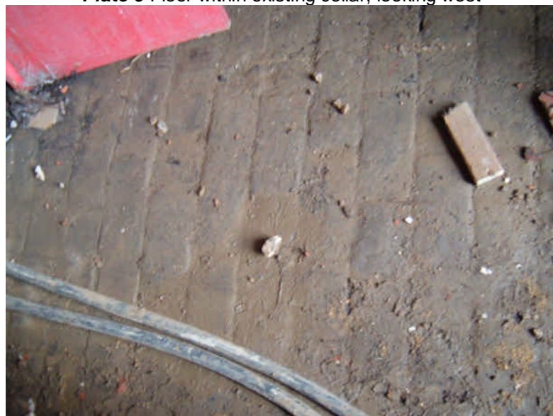
Plate 6 Floor within existing cellar, looking west
