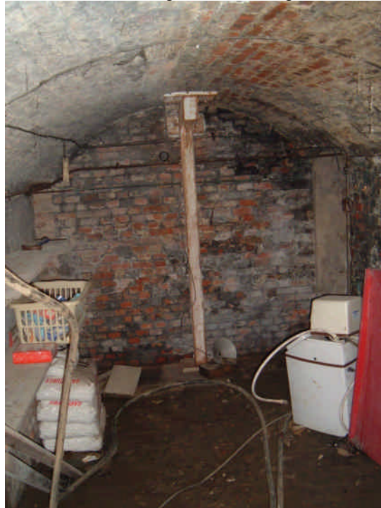
Plate 5 Existing cellar, looking south
