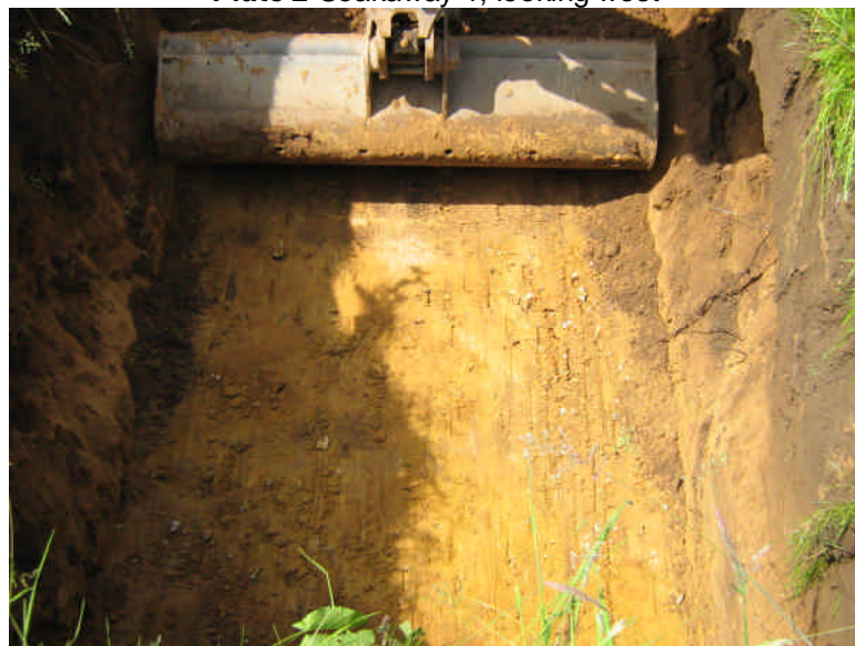
Plate 2 Soakaway 1, looking west
