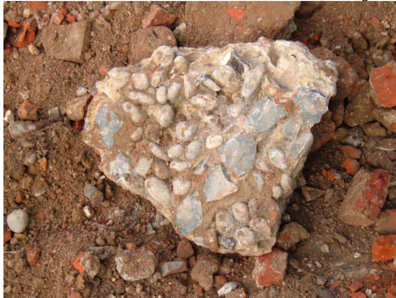
Plate 9 Flint cobbles onto which concrete floor was laid, looking north
