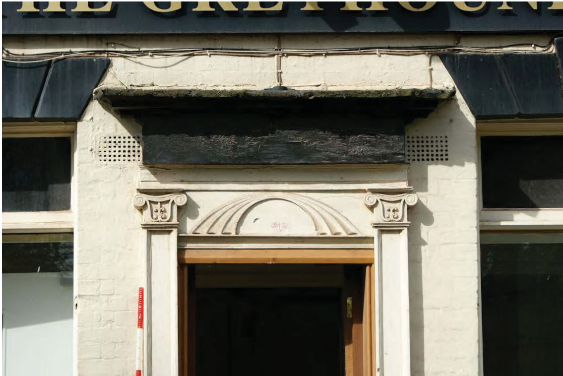
Plate 4: Above the main entrance to The Greyhound Inn is a fan frieze and moulded cornice
