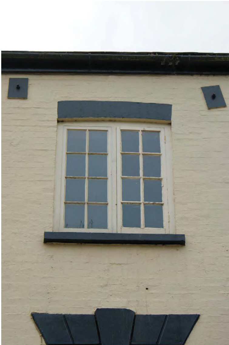
Plate 3: Detail of a second floor window opening, including slightly segmental brick arch
