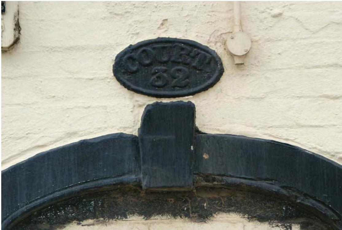
Plate 6: Detail of the oval sign above the blocked opening saying 'Court 32'
