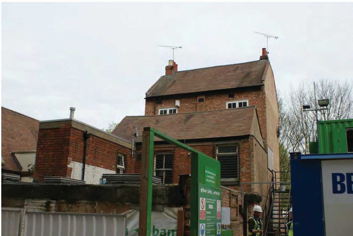
Plate 7: The rear elevation of The Greyhound Inn, from the south west
