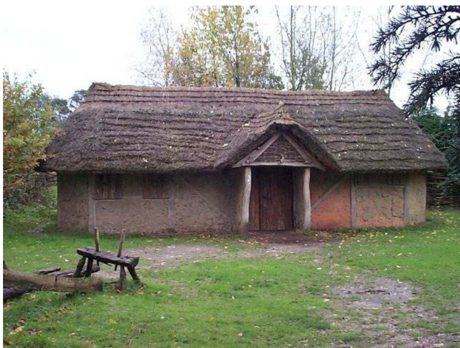
Figure 9.81. Reconstruction of a Romano-British rectangular, single-storey dwelling made of timber and wattle and daub, Upton Country Park, Dorset. (Source: World Wide Web http://www.boroughofpoole.com ).
