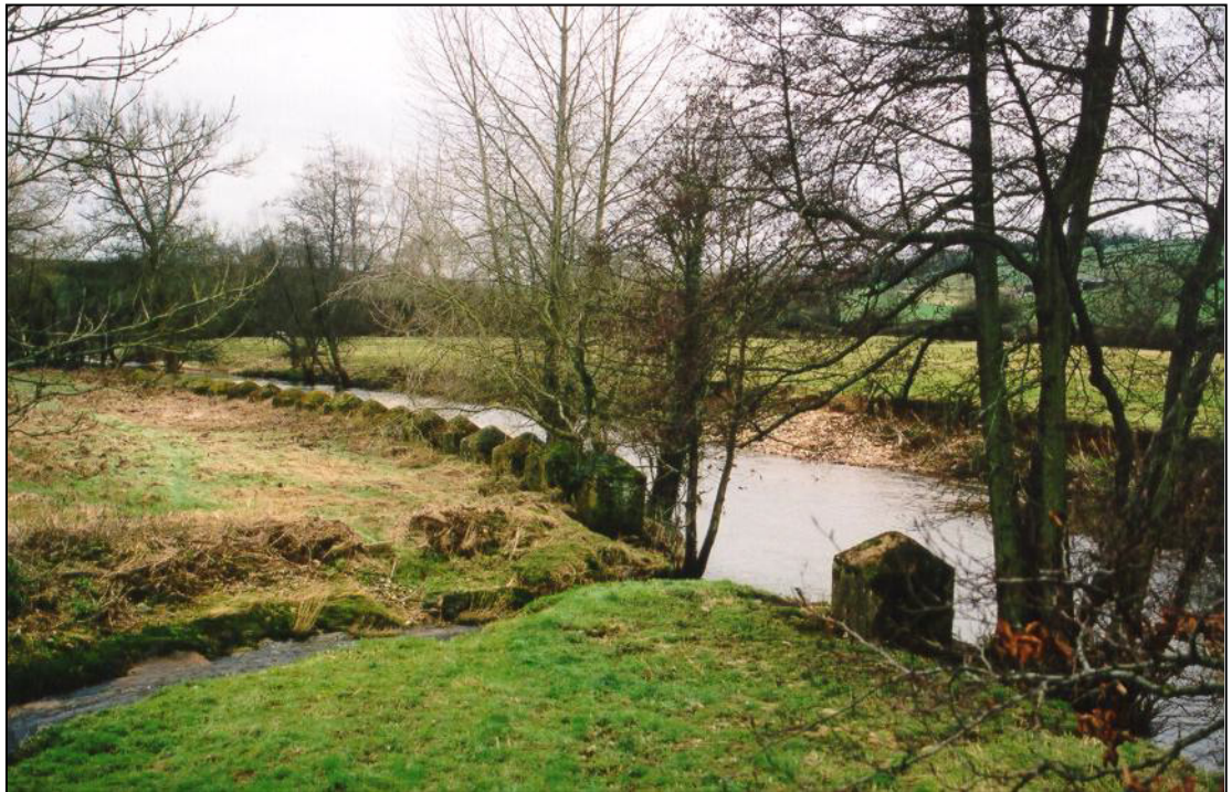
Fig. 6 - UORN 1243: a fine line of pyramidal-topped anti-tank cubes strengthening the main anti-tank obstacle of the River Axe.
