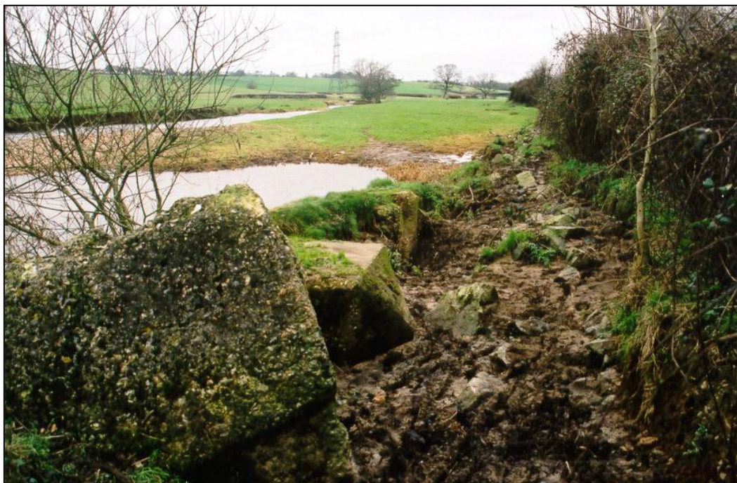
Fig. 9 - Anti-tank cubes used as river bank reinforcement [UORN 1242].
