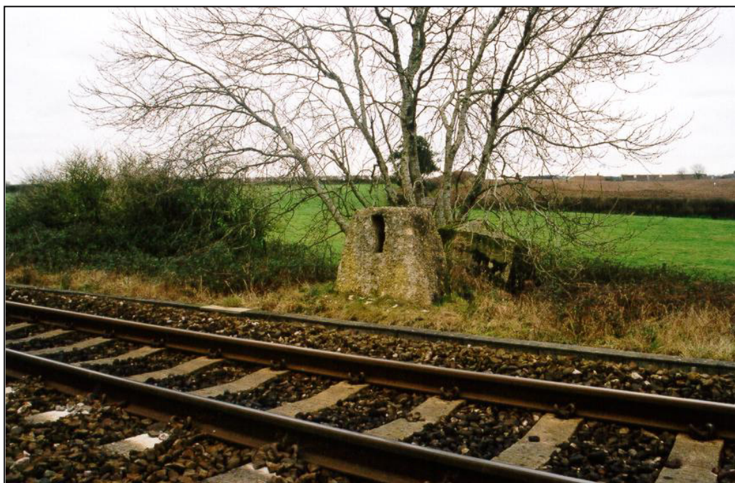
Fig. 8 - UORN 16430: one of the two facing concrete plinths of a railblock, a rare survival.
