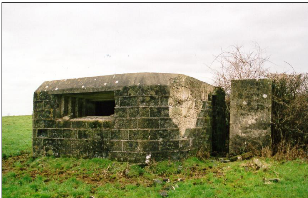
Fig. 4 - UORN 1315: powerful-looking Vickers machine gun emplacement, with large stepped embrasure and detached blast wall covering the entrance. The breeze-block shuttering is falling away in part.
