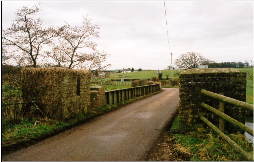
Fig. 7 - UORN 1339: fine examples of roadblock plinths to take horizontal steel beams at Axe Bridge. The rising land beyond the river can be seen: this was defended by infantry pillboxes and Vickers machine gun emplacements.
