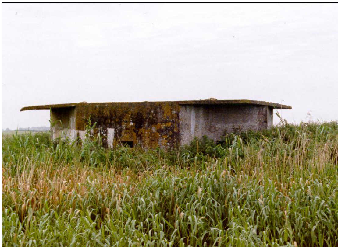
Fig. 4 - UORN 6388: type 24 pillbox, with distinctive and highly unusual overhanging roof.
