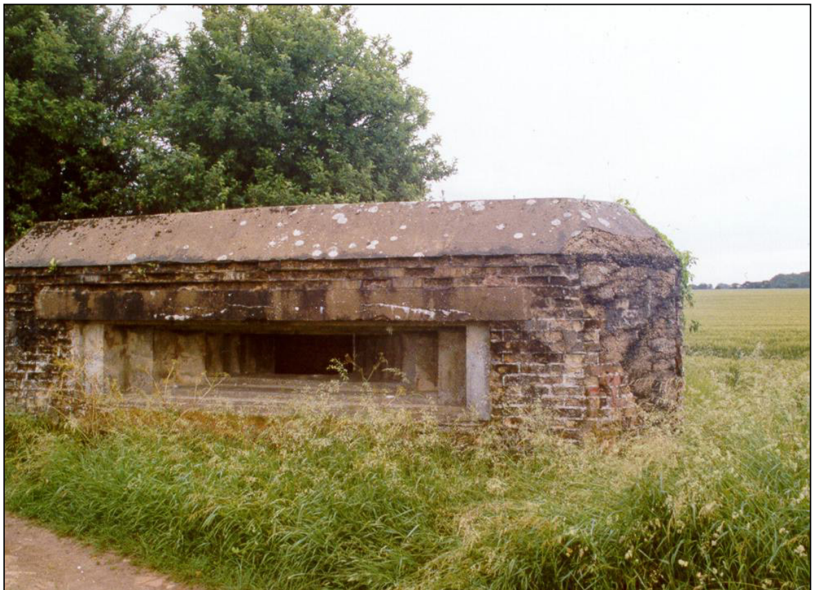
Fig. 2 - UORN 6440: brick-shuttered anti-tank gun emplacement south-east of Jude's Ferry Bridge. The holdfast survives inside to mount a 6pdr. anti-tank gun firing towards the bridge.
