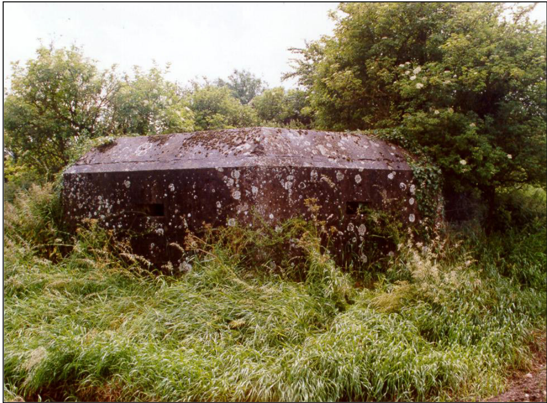
Fig. 5 - UORN 6392: type 24 concrete-faced pillbox, with chamfered roof edge to deflect incoming shells.
