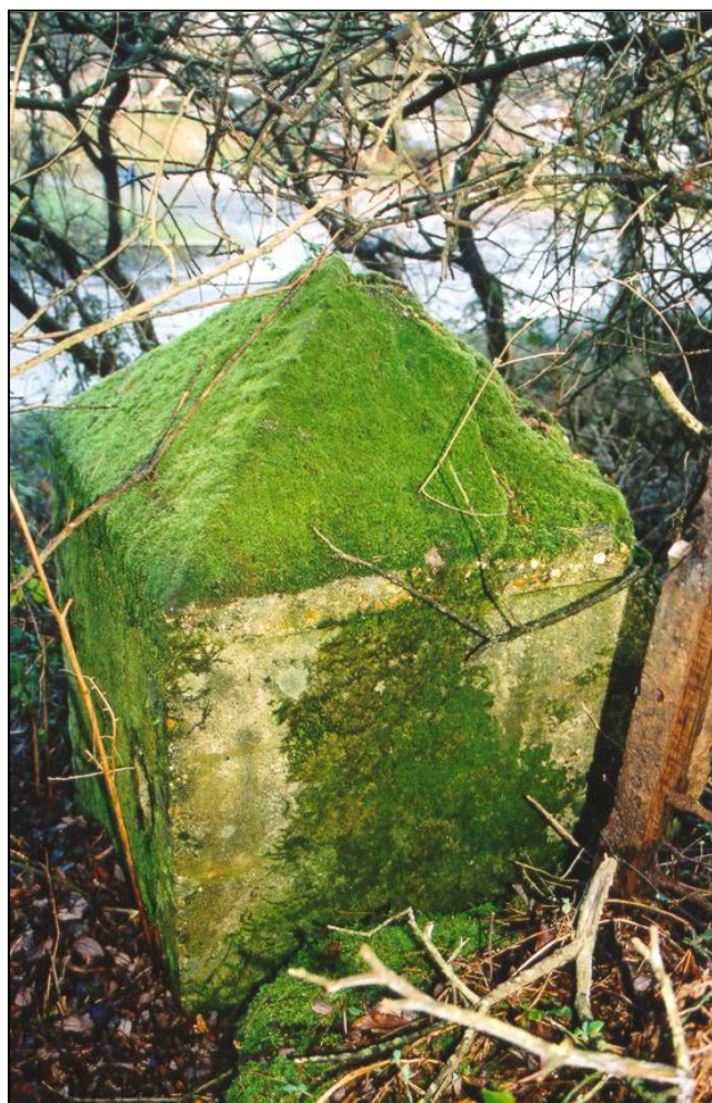
Fig. 11 - UORN 16326: a single surviving anti- tank cube, with a pyramidal top, from a long line of these that once blocked an exit from the beach just north of the present National Trust visitor centre at Knoll Beach [see as well Fig. 4].
