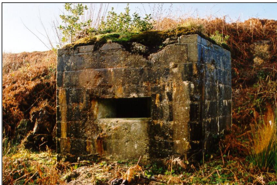
Fig. 9 - UORN 7716: pillbox with a large embrasure for a medium machine gun. It shows damage probably caused during assault training in 1944.
