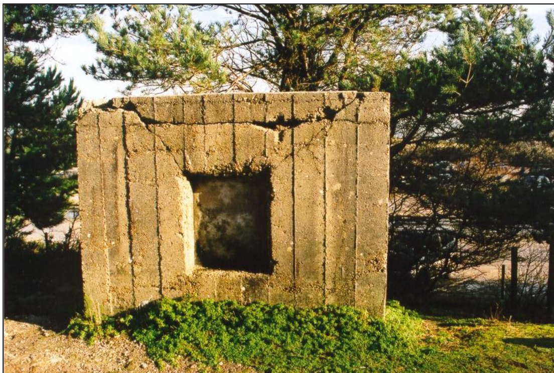
Fig. 10 - UORN 7704: the blocked doorway of a pillbox standing within the National Trust car park at Knoll Beach. Unusually, the pillbox was constructed using vertical wooden shuttering.
