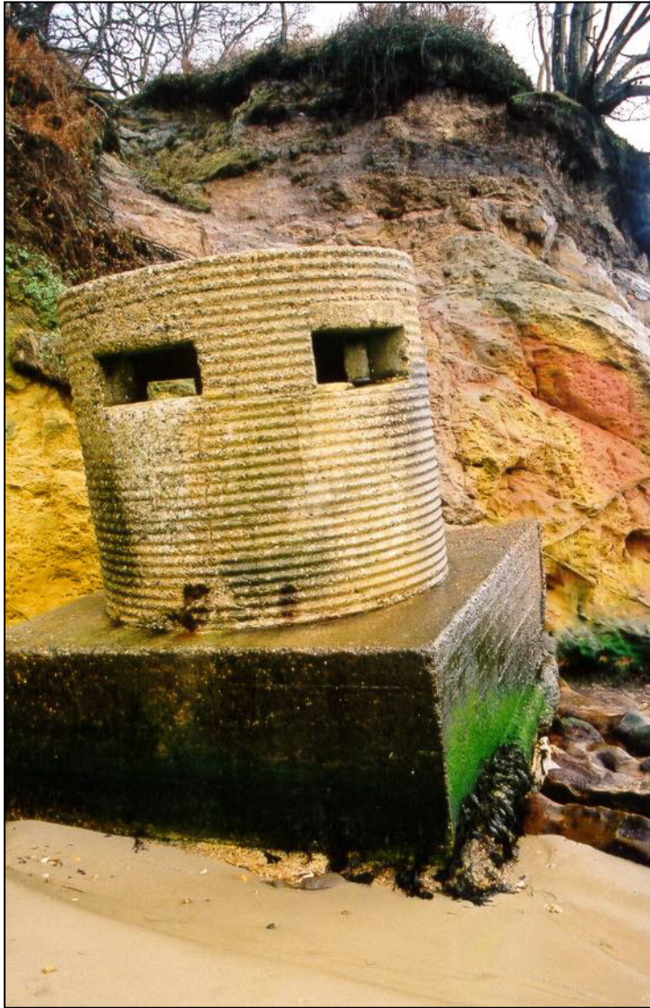
Fig. 8 - UORN 7718: type 25 corrugated-iron shuttered pillbox in a remarkably exposed position beneath the cliffs of Redend Point. It has survived for sixty years, but is unlikely to do so for a further sixty.
