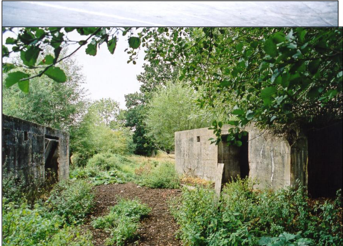
Fig. 5 - UORN 2681: the interior of the type 28A anti-tank gun emplacement, with two main embrasures [now blocked in]. There are two side chambers, to right and left, for LMG fire.
