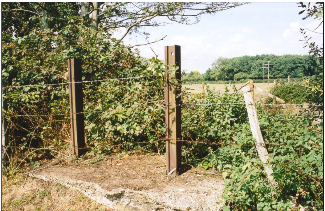
Fig. 11 - UORN 5717: these two steel vertical rails, used today as posts for a barbed wire fence, once helped block a gap in the anti-tank ditch at this point. Other rails are perhaps hidden by bushes.
