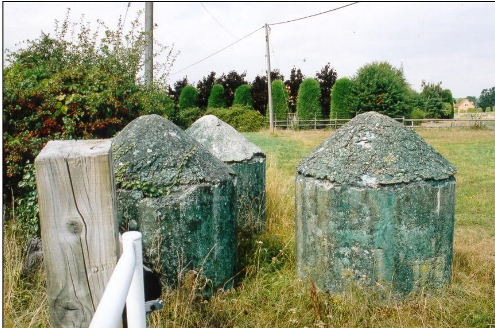
Fig. 10 - UORN 2684: anti-tank cylinders that once formed part of a roadblock at a crossing of the anti-tank ditch stand in a field by the lane.
