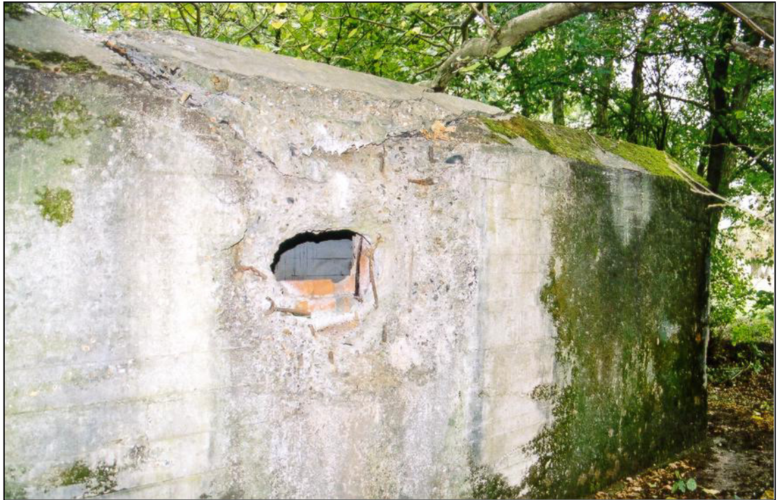
Fig. 8 - Damage to one of the faces of UORN 2683, possibly occasioned in wartime tests of concrete-piercing weapons.
