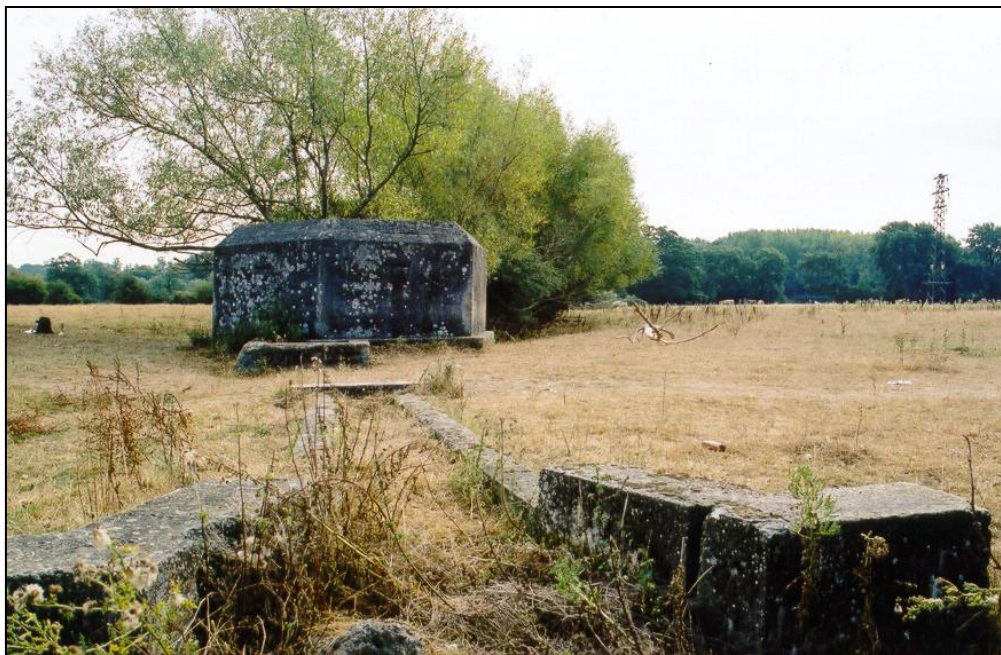
Fig. 9 - UORN 5709: small, thick-walled pillbox standing in the open grassland at the north of the defence area. The structure in the foreground is a drainage sluice, which might be associated with the square structure projecting from the concrete base of the pillbox.
