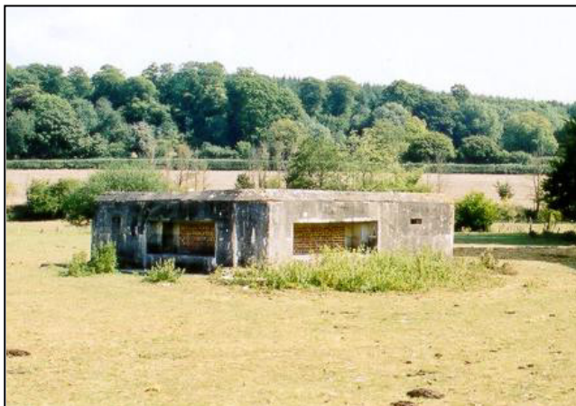
Fig. 4 - UORN 5719: anti-tank gun emplacement with two main embrasures [now blocked in] firing in different directions along the adjacent anti-tank ditch.
