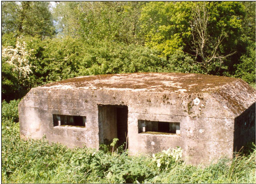
Fig. 6 - UORN 12995: an excellent example of a shell-proof type 24 pillbox with chamfered roof edges dug into the bank of the River Chelmer west of Hartford End.
