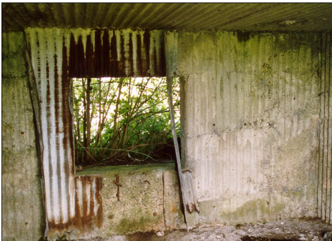
Fig. 8 - UORN 7186: interior of the anti-tank gun emplacement commanding Hartford End bridge, with some of its corrugated-iron shuttering still in place.
