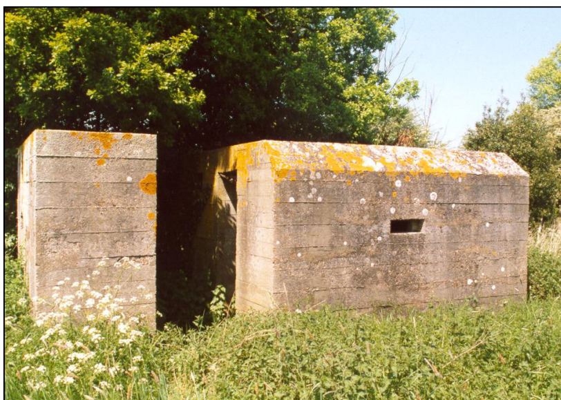
Fig. 5 - UORN 7571: Eastern Command type of heavy infantry pillbox with detached external blast wall.
