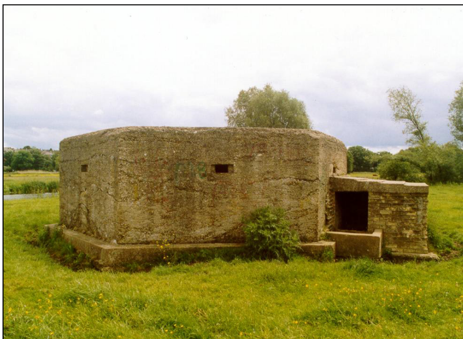
Fig. 2 - UORN 6433: a type 27 pillbox with covered entry porch. Almost all the original external brick shuttering has gone.
