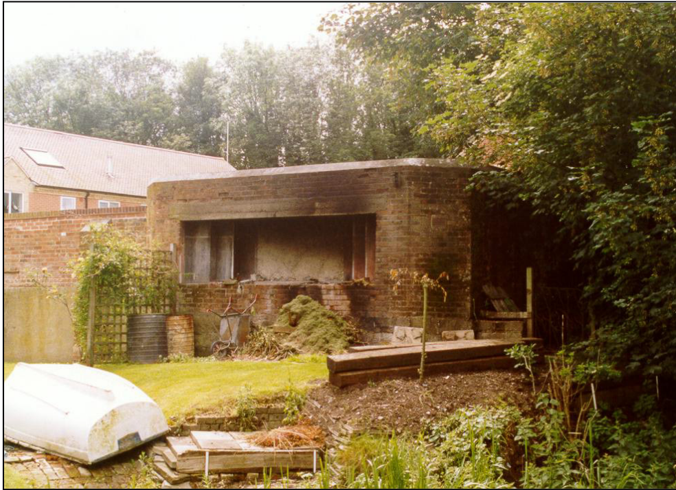
Fig. 4 - UORN 11781: anti-tank gun emplacement with mounting for a 6pdr. gun. The main embrasure has been blocked. This is an important structure surviving in a back garden.
