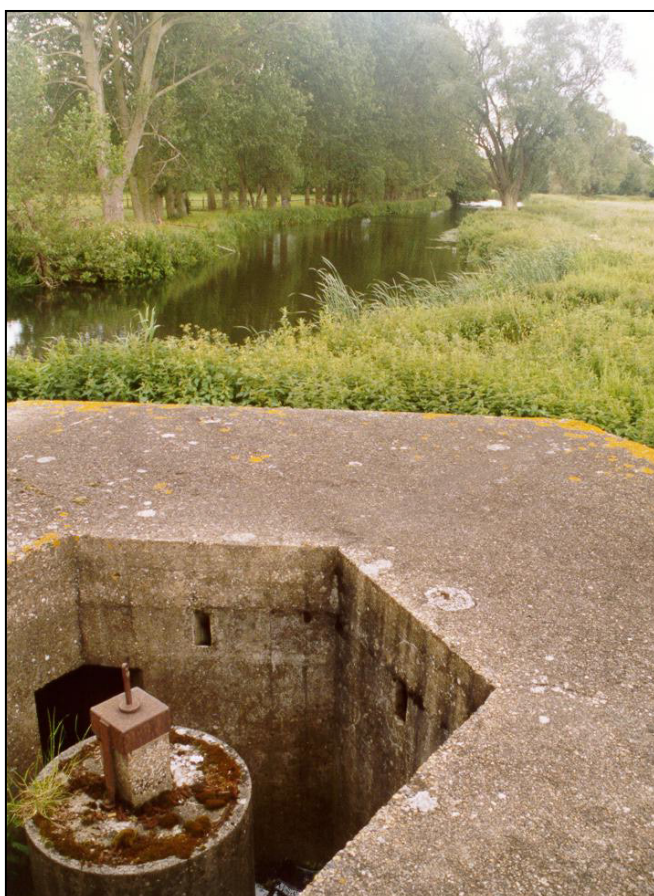
Fig. 3 - UORN 648: type 27 pillbox showing the central AA gun mounting.
