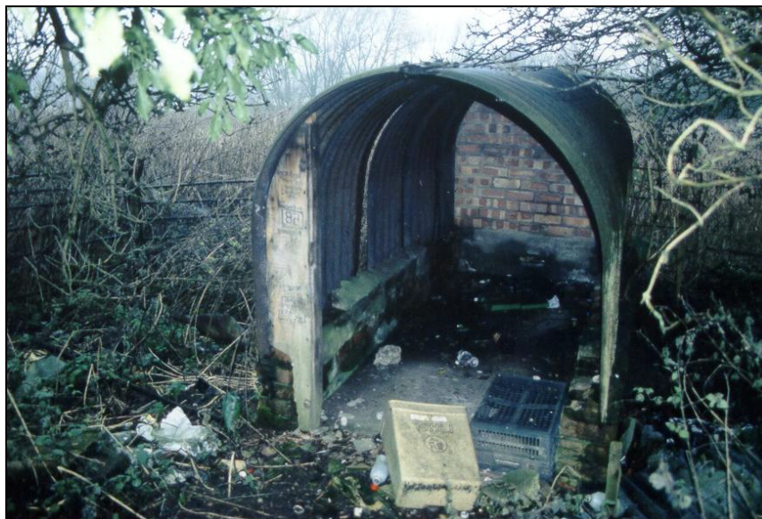
Fig. 11 - UORN 16253: Home Guard ammunition store made from the corrugated iron framework of an Anderson air raid shelter.
