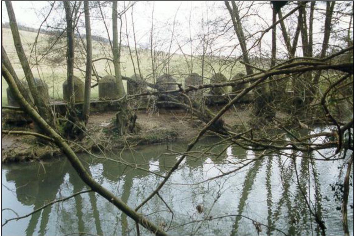
Fig. 11 - UORN 9431: a line of concrete cylinders strengthens the bank of the River Mole as an anti-tank obstacle.
