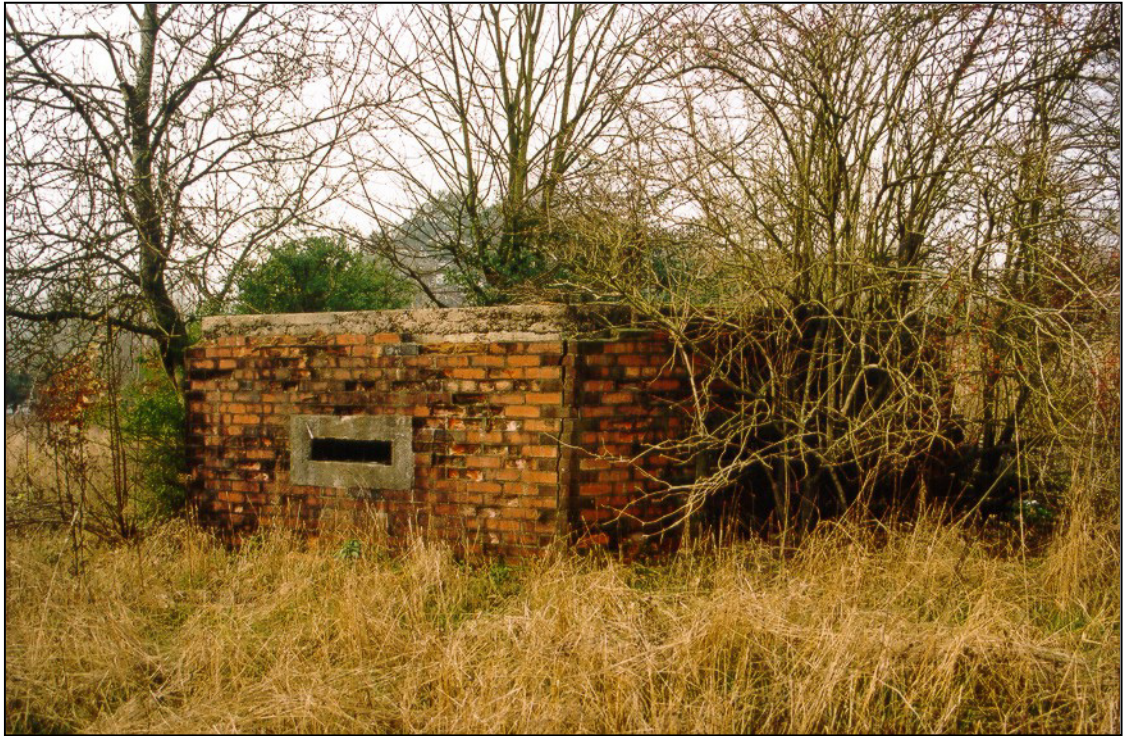
Fig. 13 - UORN 9436: brick-shuttered type 24 pillbox firing towards the A24 road at the extreme north of the defence area.
