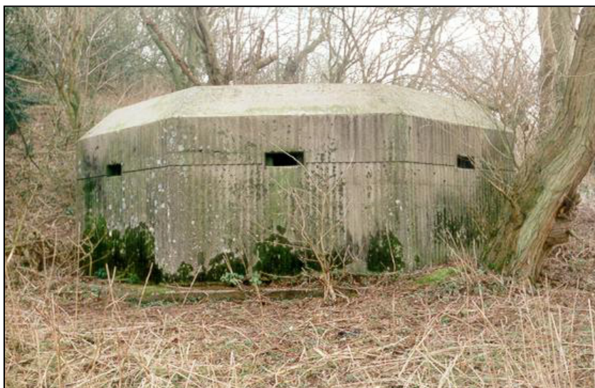
Fig. 10 - UORN 6830: type 24 pillbox with an unusual appearance, having been constructed using corrugated iron for the exterior shuttering.
